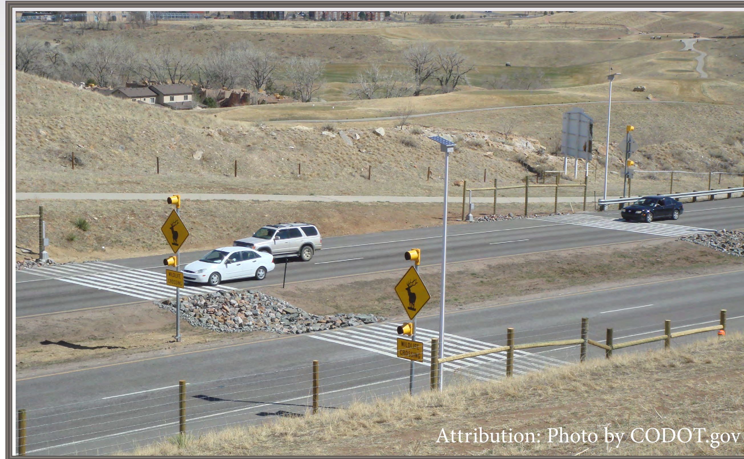
At-Grade Wildlife Crossing with Detection System
