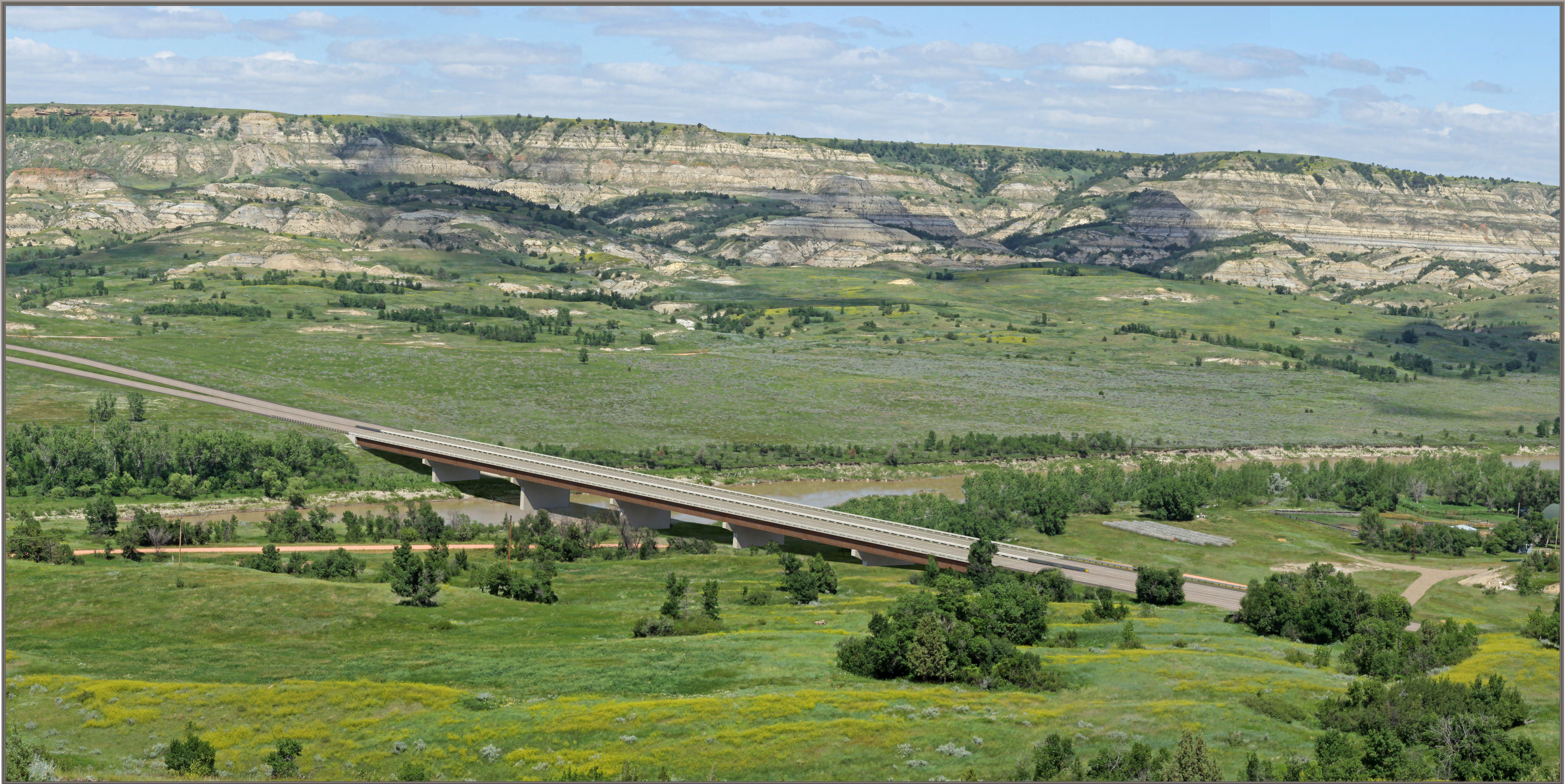
Remove & Replace Existing Bridge with New Four-Lane Bridge
