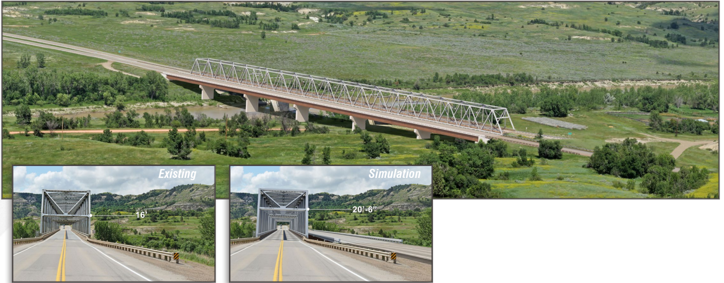
figure 8. Increase Vertical Clearance of Existing Bridge and Construct New Two-Lane Bridge Adjacent
