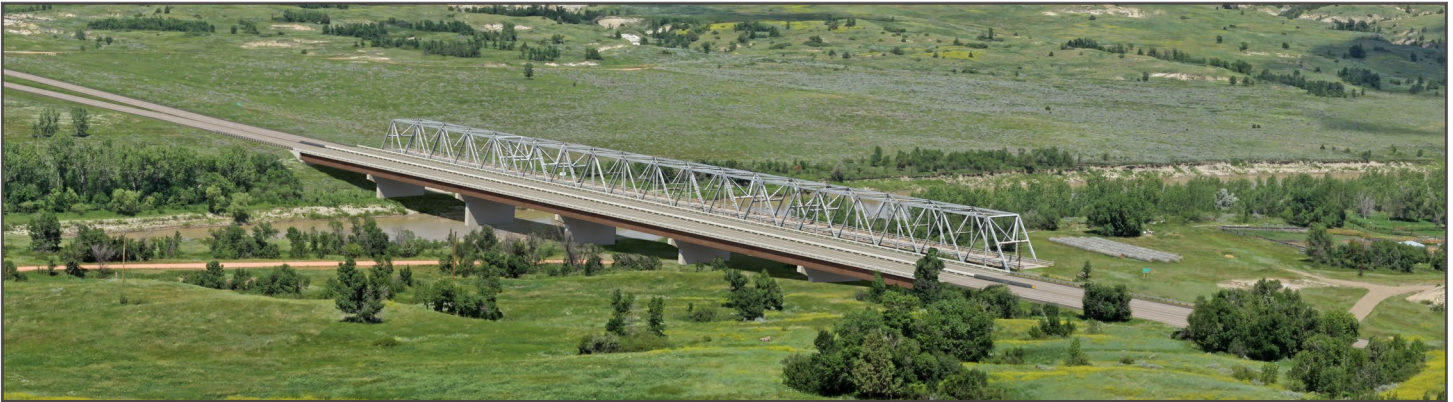
figure 9. Retain Existing Bridge for Alternative Use and Construct New Four-Lane Bridge Adjacent
