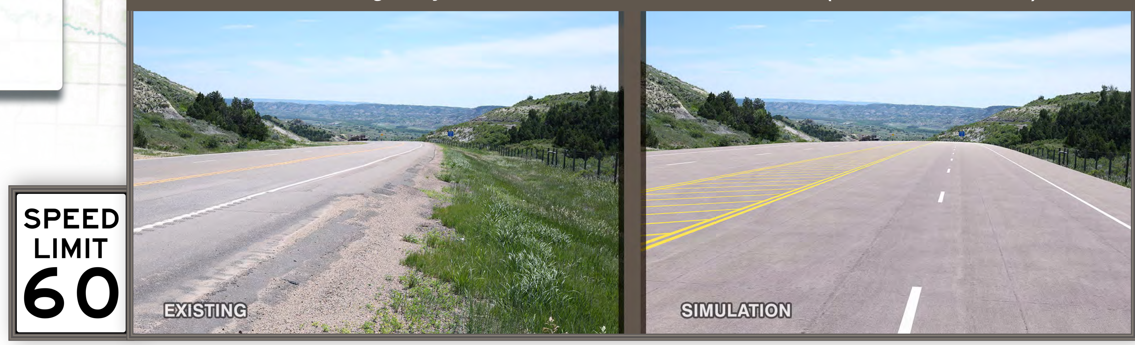
Four-lane Divided Highway with Flush, 12-foot-wide Median (RP 127.2 to 130.0)
