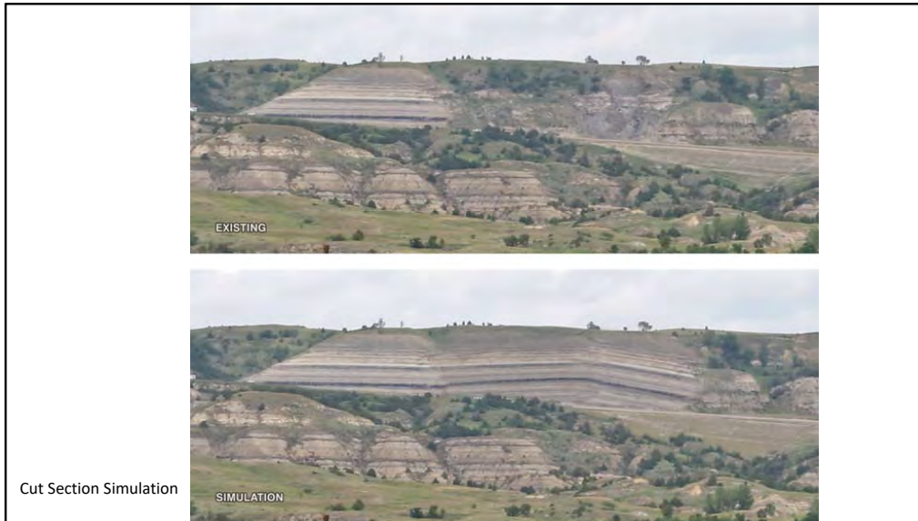
This viewshed analysis simulation depicts the extension of an existing cut section where stratified geological layers are visible, as viewed from the Maah Daah Hey trail.
