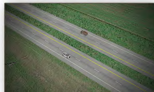
Alternative B: 4-Lane Divided—Depressed Median
