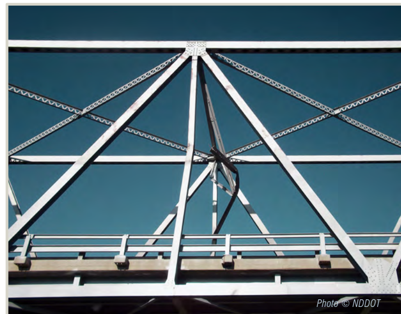
Numerous collisions have caused appreciable damage to the Long X Bridge, including the bent and displaced portal member and damaged truss vertical member shown.
