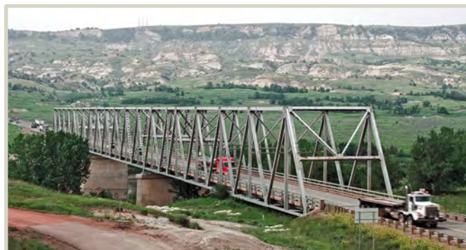
Setting Area 6, Long X Bridge
