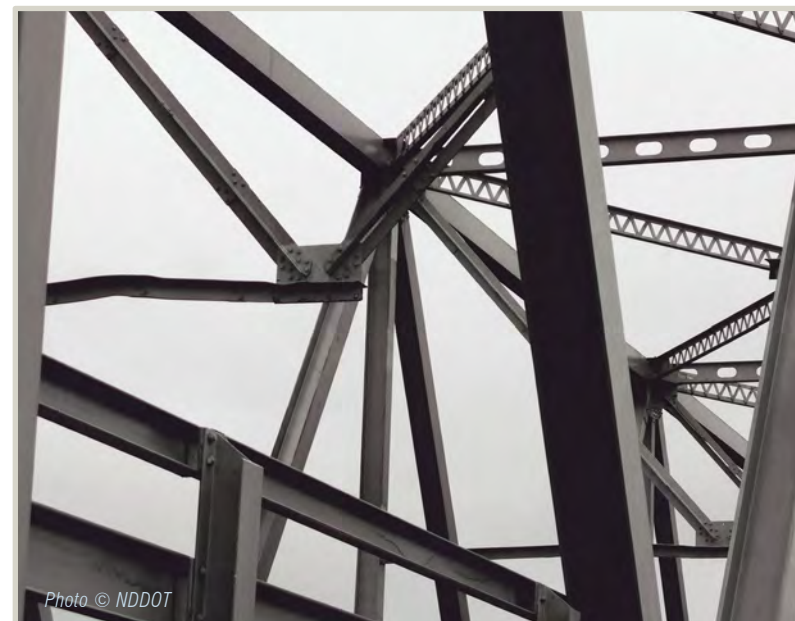
Numerous collisions have caused appreciable damage to the Long X Bridge, including the bent and displaced portal member and damaged truss vertical member shown.
