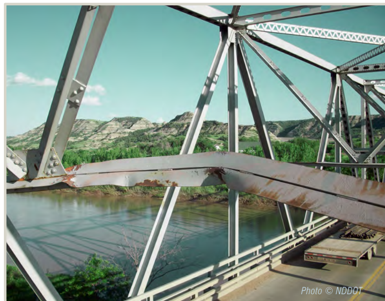
Numerous collisions have caused appreciable damage to the Long X Bridge, including the bent and displaced portal member and damaged truss vertical member shown.
