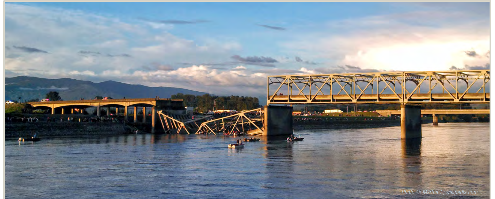
Figure 85, Example of Fracture Critical Bridge Failure caused by an oversized load striking portal members on the Skagit River Bridge on Interstate 5 in Washington
