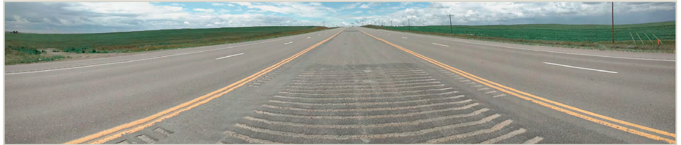
Figure 15, Example of Divided Four-lane Section with a Flush, Center Median along US Highway 85
