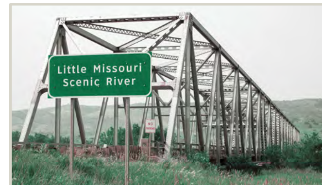
Long X Bridge (32MZ1807)
