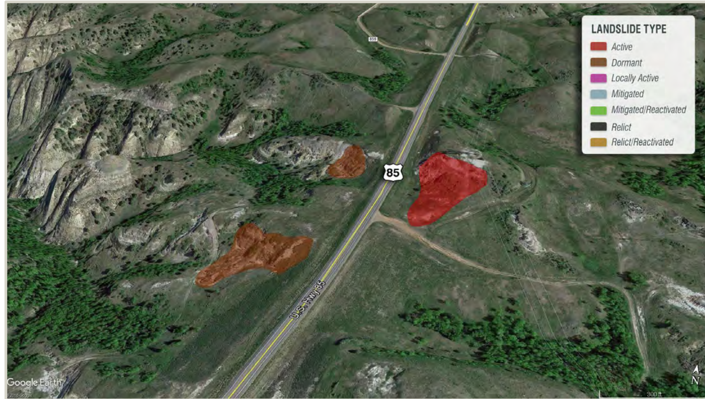
Figure 54, Google Earth Aerial Image of Mapped Landslides (Southern Portion of Badlands)
