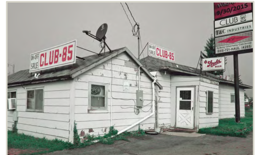
Club-85, located in Fairfield, along US Highway 85
