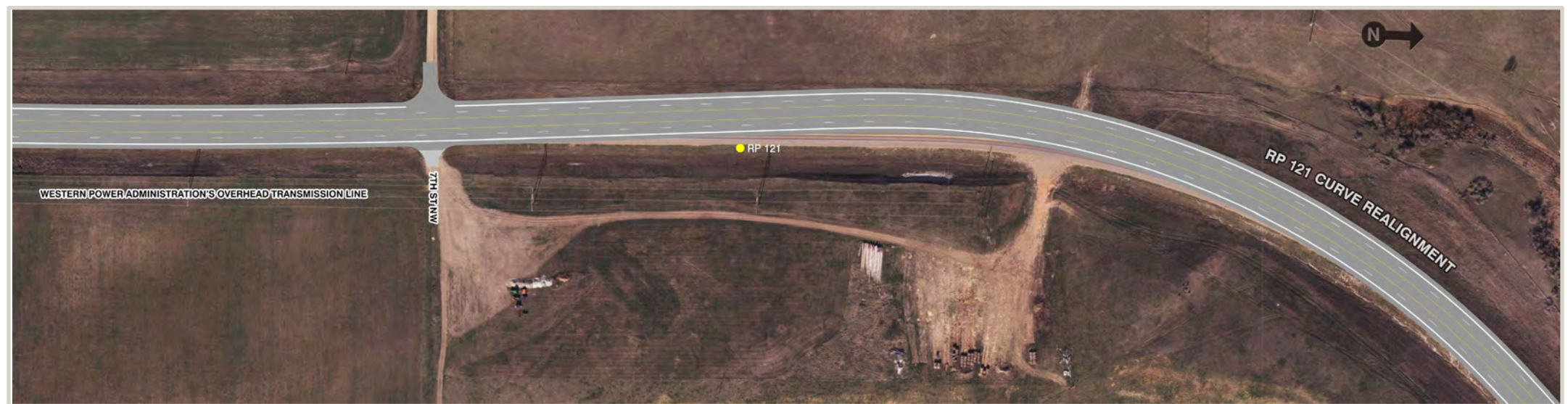
Figure 31, Curve Realignment at RP 121
