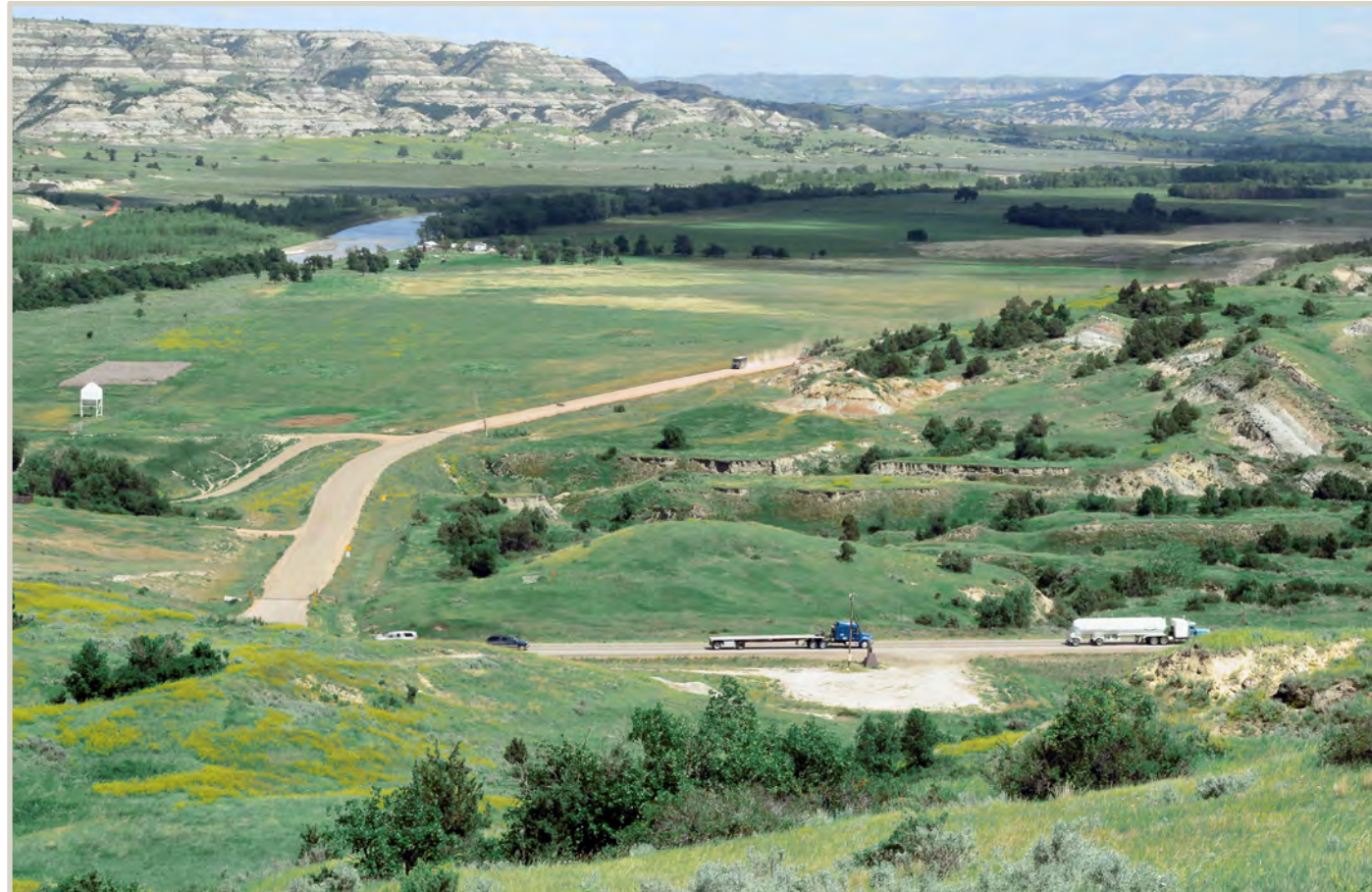
Setting Area 6, view east toward Long X Road
