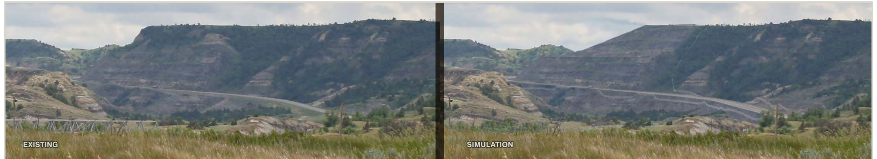
Figure 78, Large Flattened Slope and Wildlife Fencing (Temporary Visitor Center Vantage Point)
