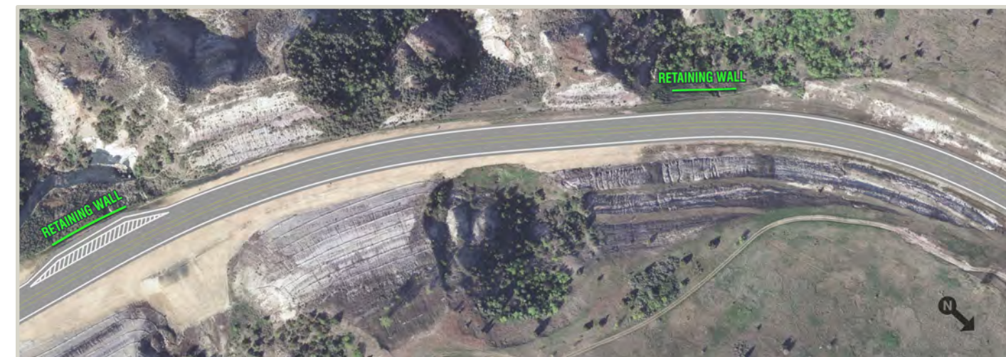
Figure 25, Retaining Walls along TRNP–North Unit
