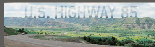
I-94 Interchange to Watford City Bypass (McKenzie County Road 30) Project 9-085(085)075 PCN 20046 • Stark, Billings and McKenzie Counties, North Dakota
