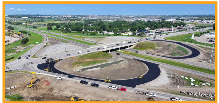
From the SE, crews paving temporary loop ramps.
