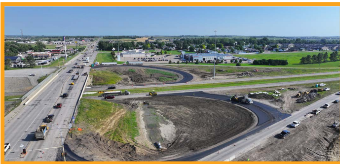
From the S, looking at the two temporary loop ramps
