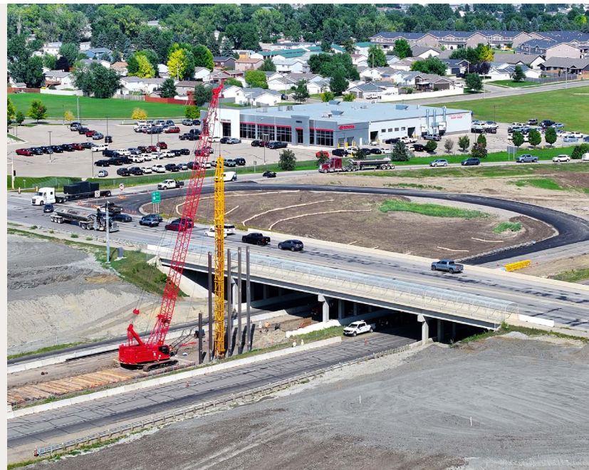
From the SE, crews paving temporary loop ramps.
