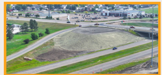
From SW, looking at the NW bridge abutment embankment.
