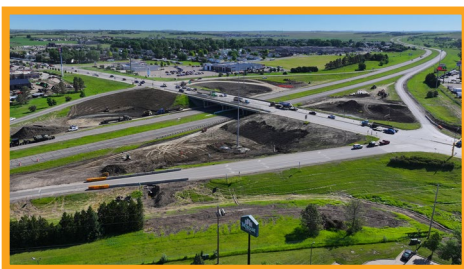
From the SW, showing progress on bridge abutment embankment areas.
