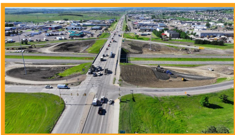
From the N, showing north bridge abutment
