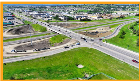
From the NE, showing temporary loop ramp embankment
