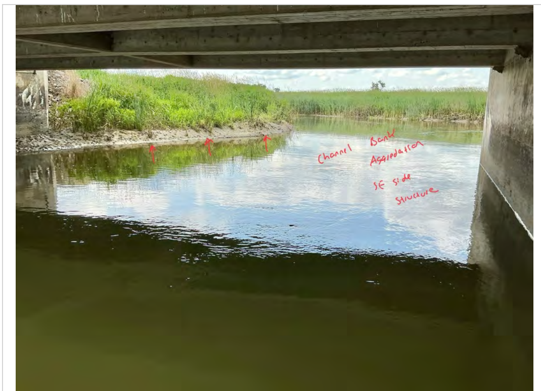
Facing South. East Channel Bank Aggradation South of Structure.
