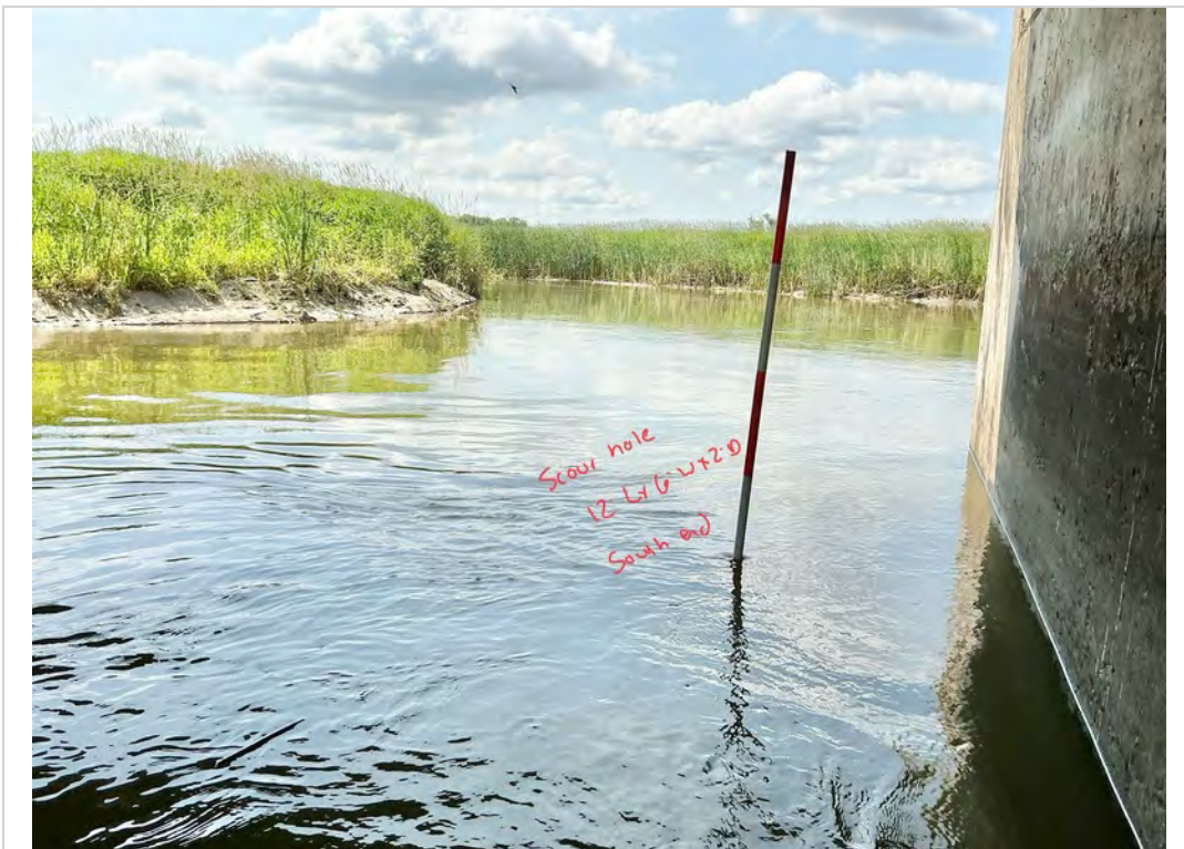
Facing South. Range Pole used to determine Scour Depth along West Abutment.
