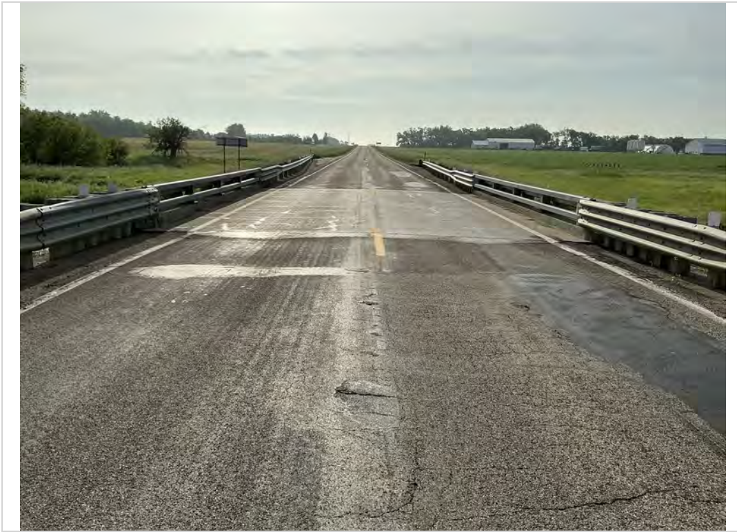
Facing East. Approach View.
