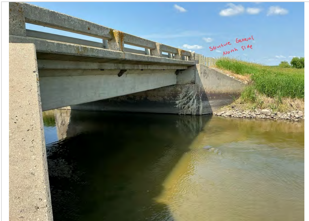
Facing West. Structure General along North Side.
