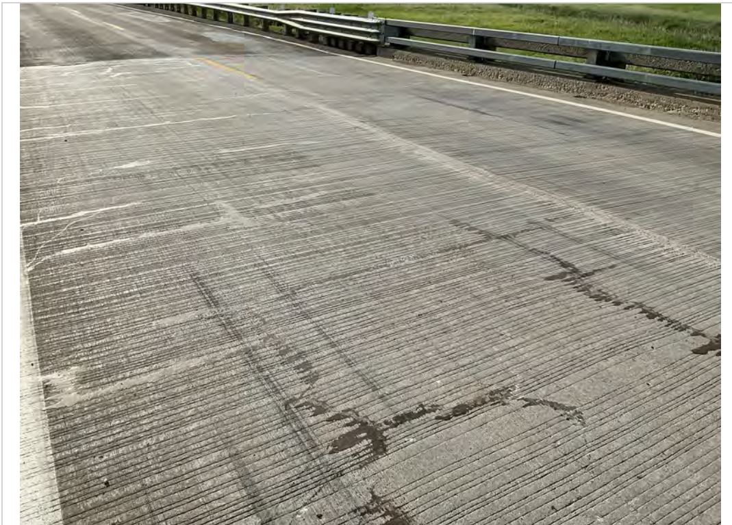
Facing SE. General of Top Flange Deck Wearing Surface.
