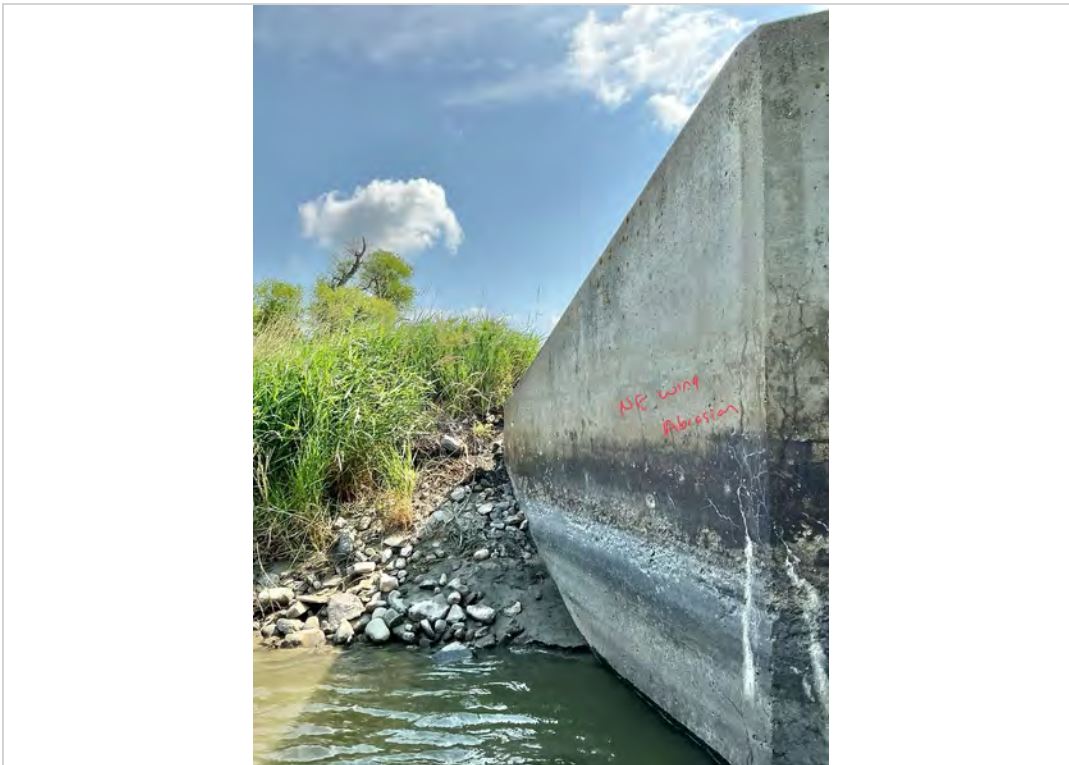
Facing East. Abrasion to NE Wing.
