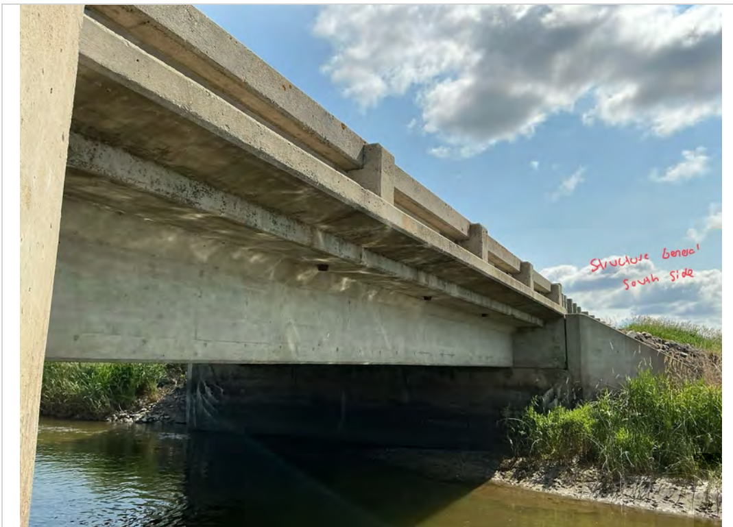
Facing East. Structure General along South Side.
