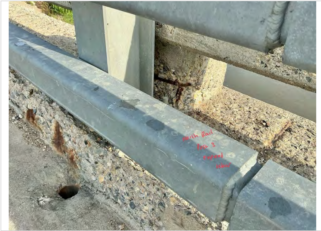
Facing NW. Exposed Rebar to North Railing Post 3.
