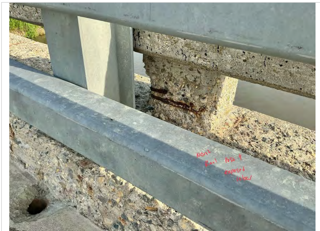
Facing NW. Exposed Rebar to North Railing Post 4
