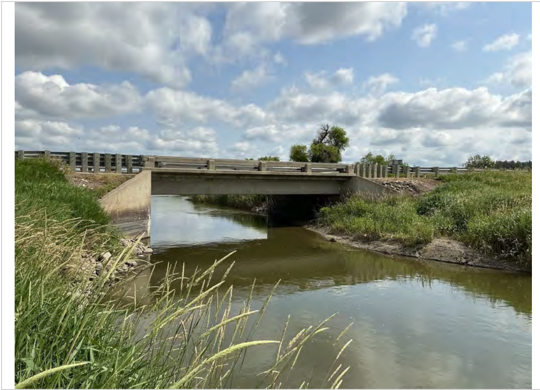
Facing North. Side View.
