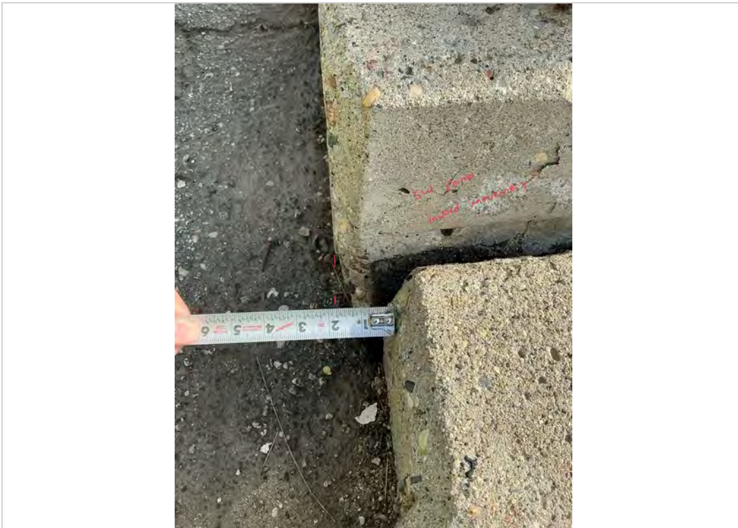
Facing North. SW Wing at Top Inward Movement measurement.
