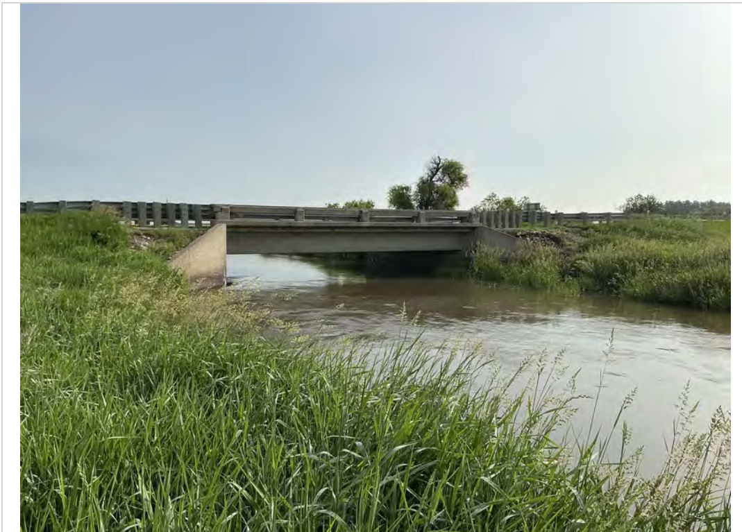
Facing North. Side View.
