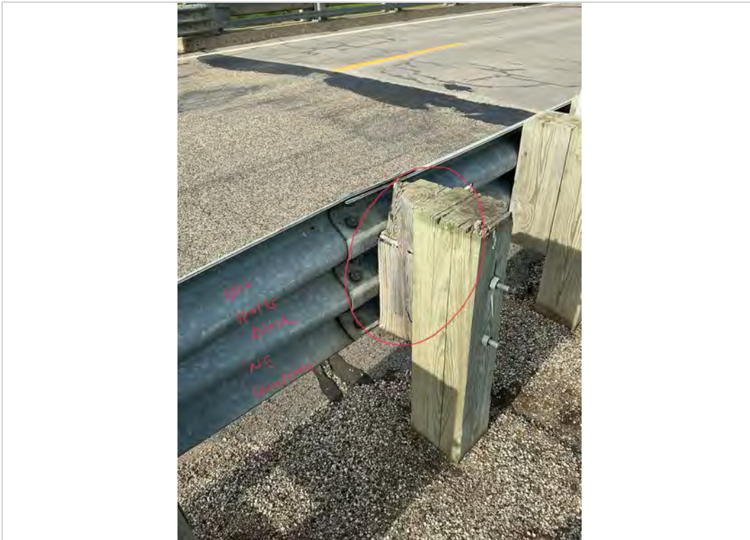
Facing SW. Split Wood Spacer Block NE Quadrant.
