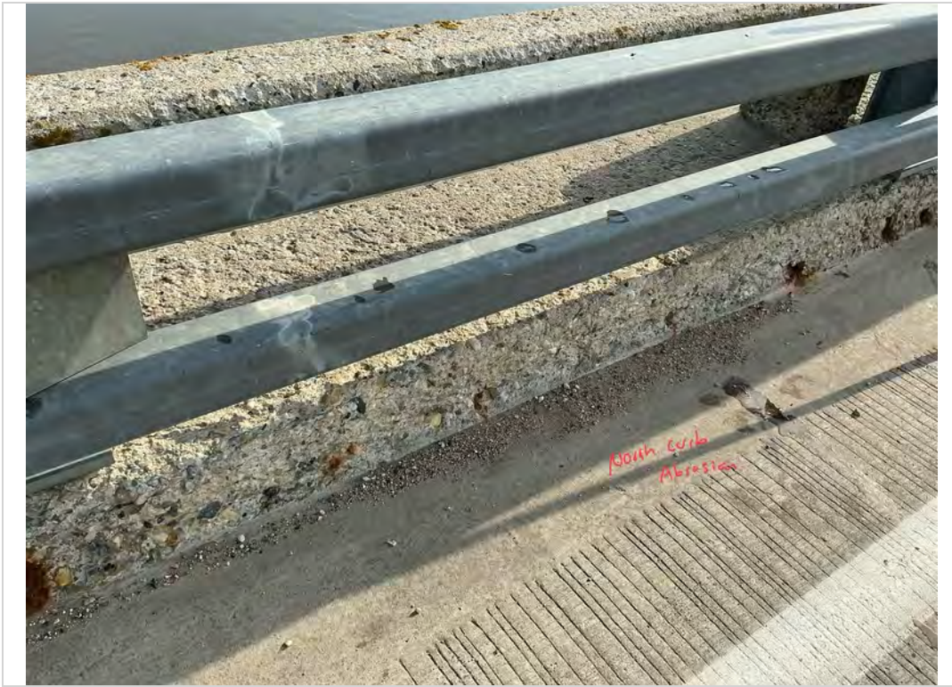
Facing NE. Abrasion to North Curb.
