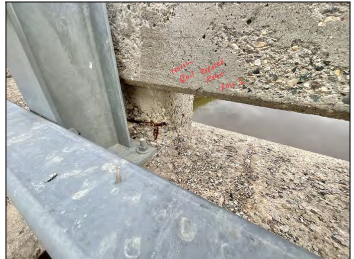
Facing NE. Exposed Rebar to North Railing at Post 3.
