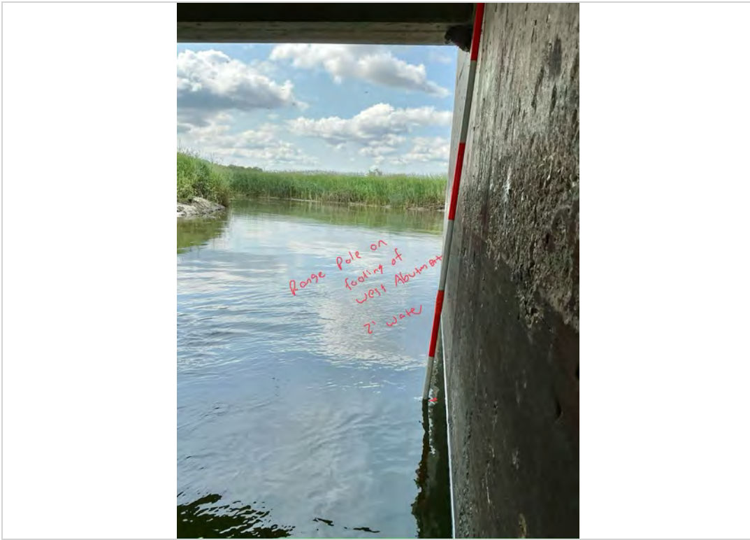
Facing South. Range Pole I used to determine water depth along Exposed Top of Footing.
