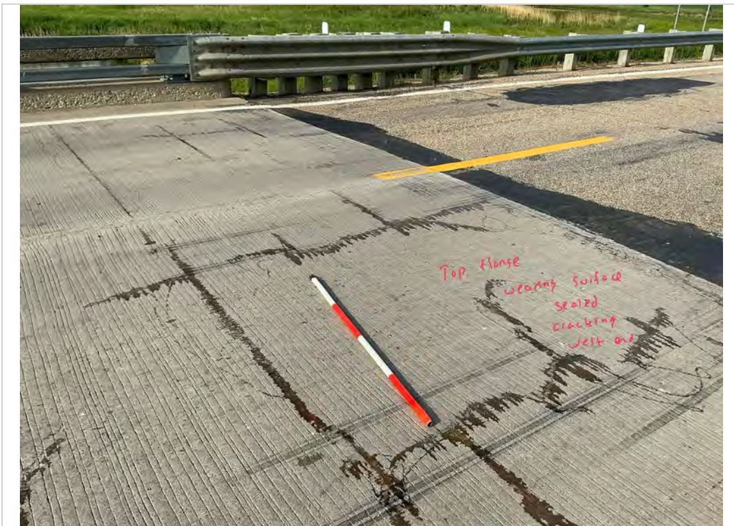
Facing SW. Sealed Cracking to Top Flange Deck Wearing Surface West End.
