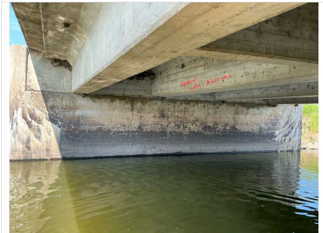
Facing West. General of West Abutment.
