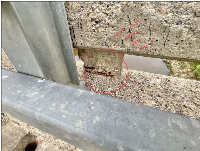
Facing North. Exposed Rebar to North Railing Post 4.
