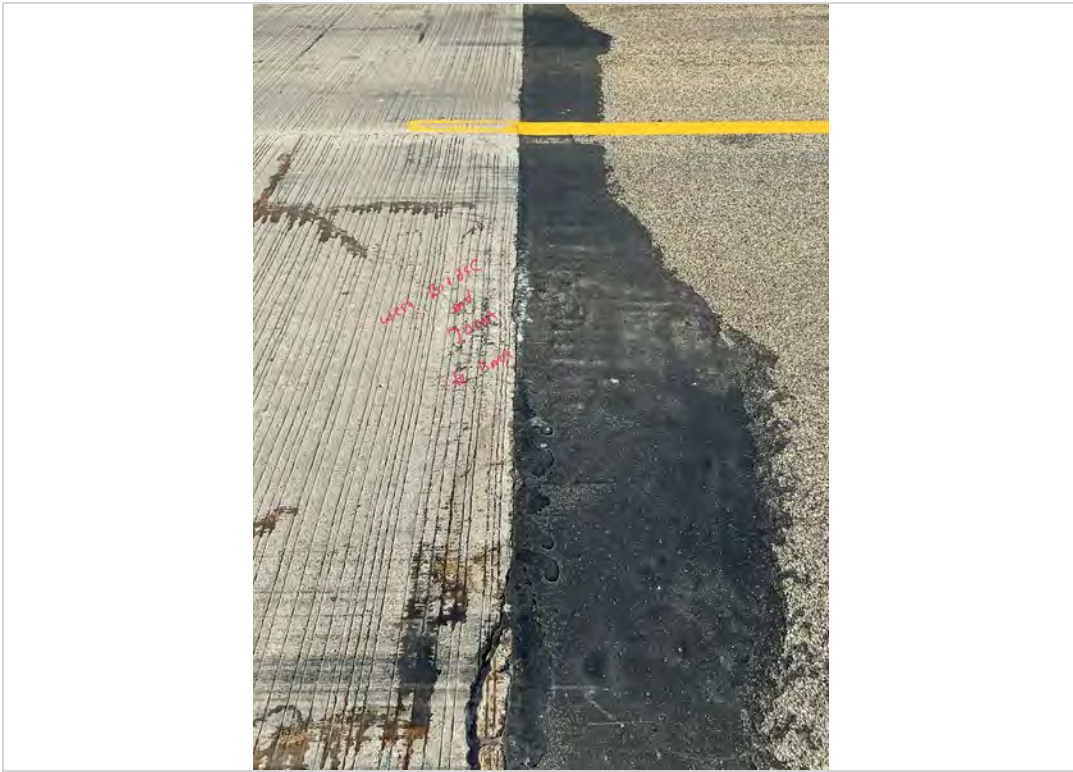
Facing West and Downward. West Bridge End Joint
