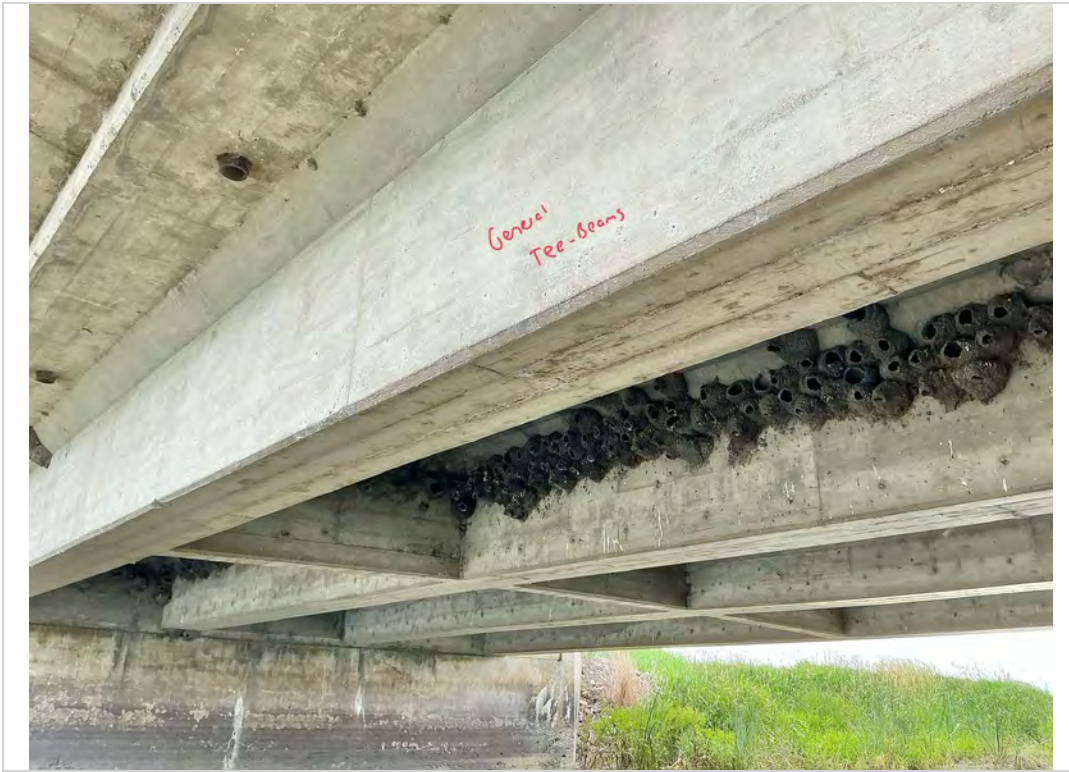
Facing SE. General of Tee Beams.
