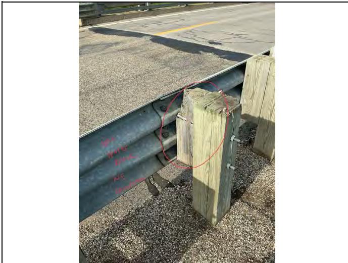
Facing SW. Split Wood Spacer Block NE Quadrant.
