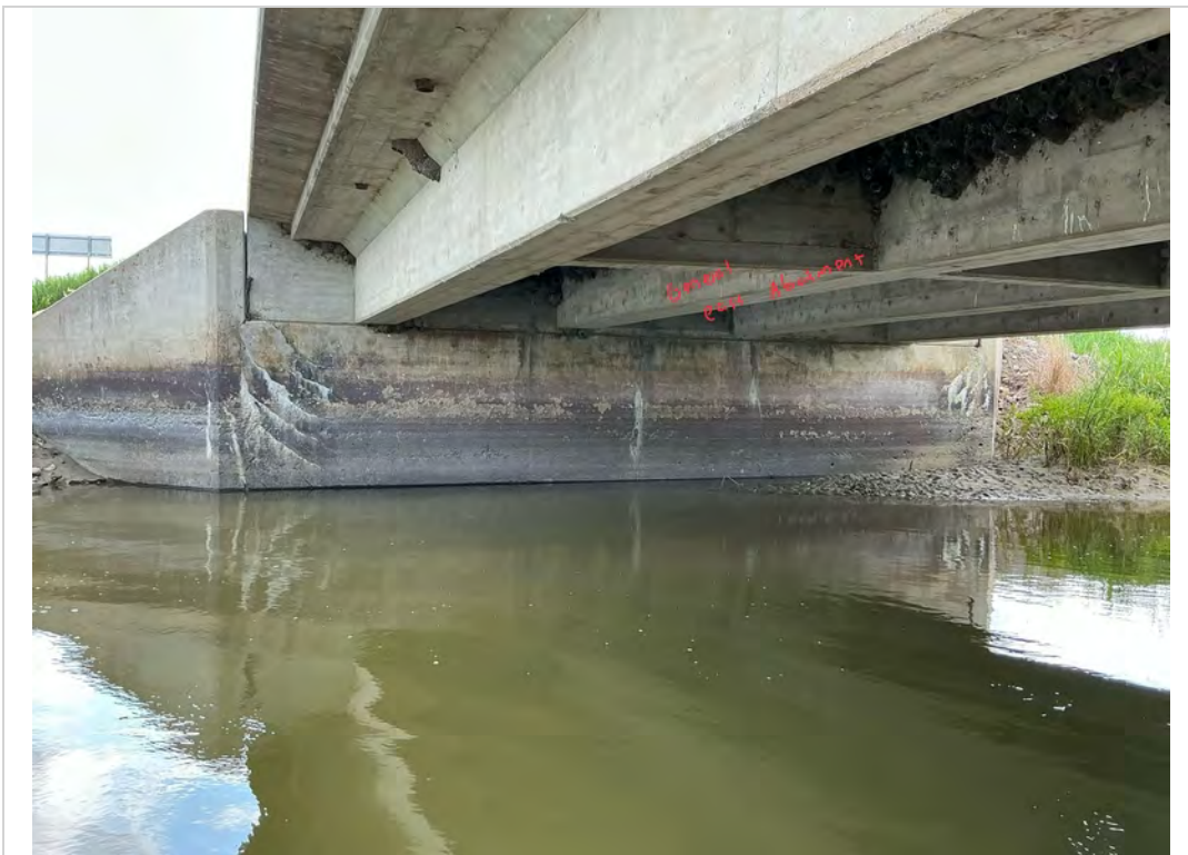
Facing East. General East Abutment.
