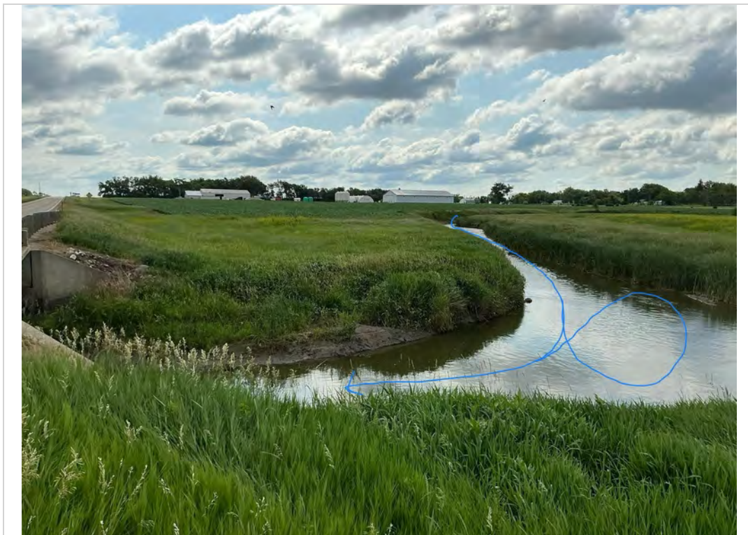
Facing SE. Channel alignment from the SE.
