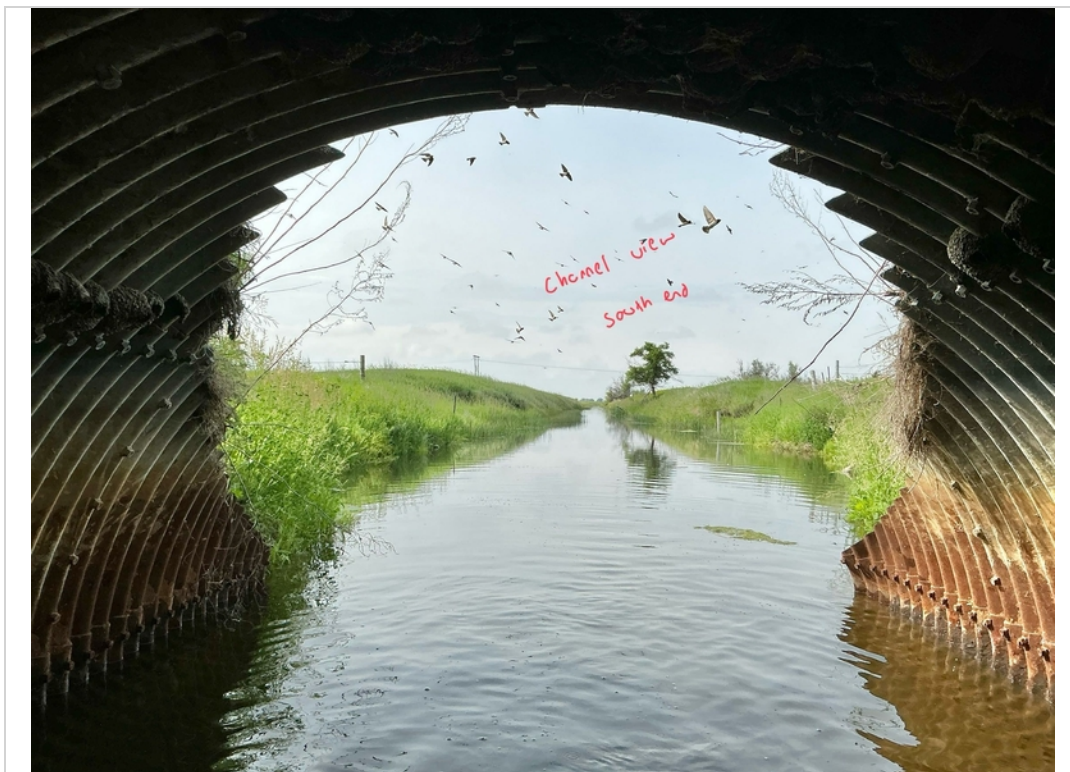
Facing South. Channel View South End.
