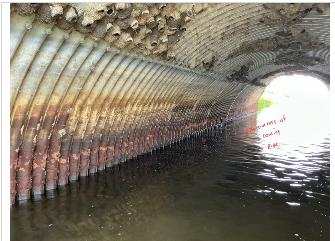
Facing South. Effectiveness of coating throughout Pipe.
