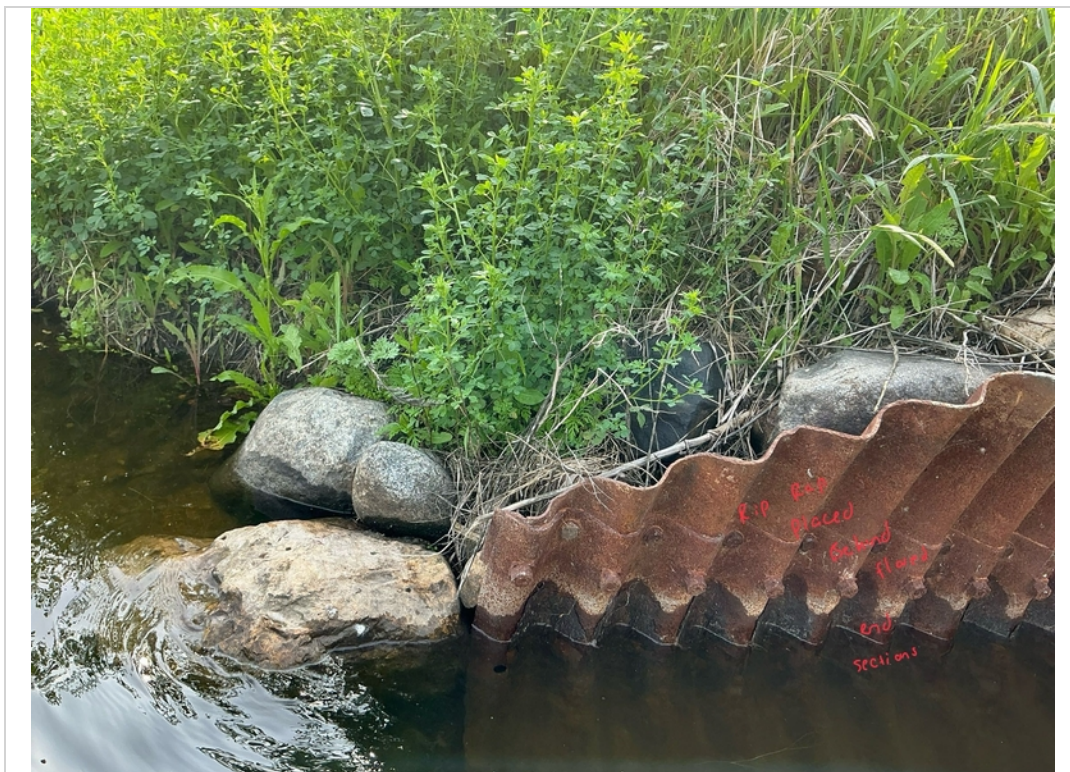
Facing East. Rip Rap placed behind NE Flared End Section. Typical all corners.
