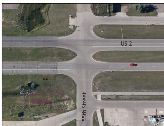
Figure 21: Shared Use Path Terminates at 55th Street Existing Facilities
