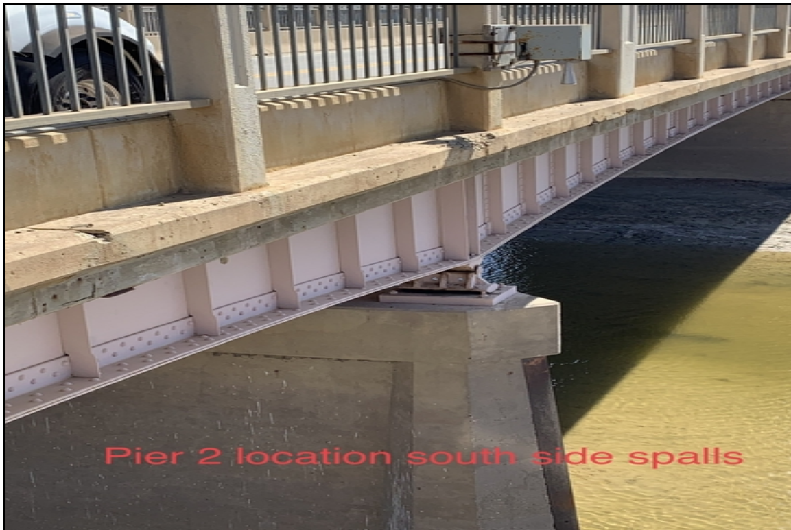
Pier 2 location south over hang spalls
