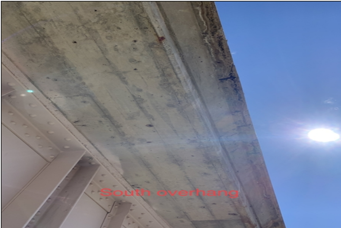
South side soffit spalling exposed rebar
