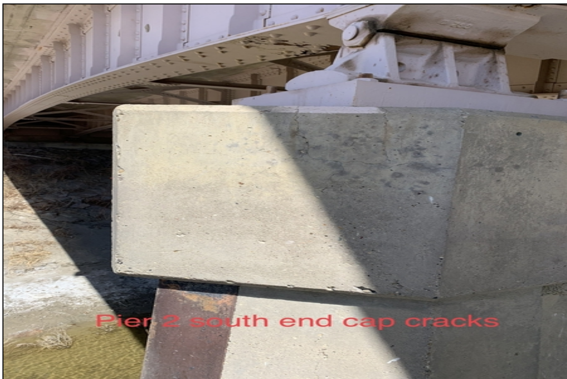
Pier 2 south end cap cracks
