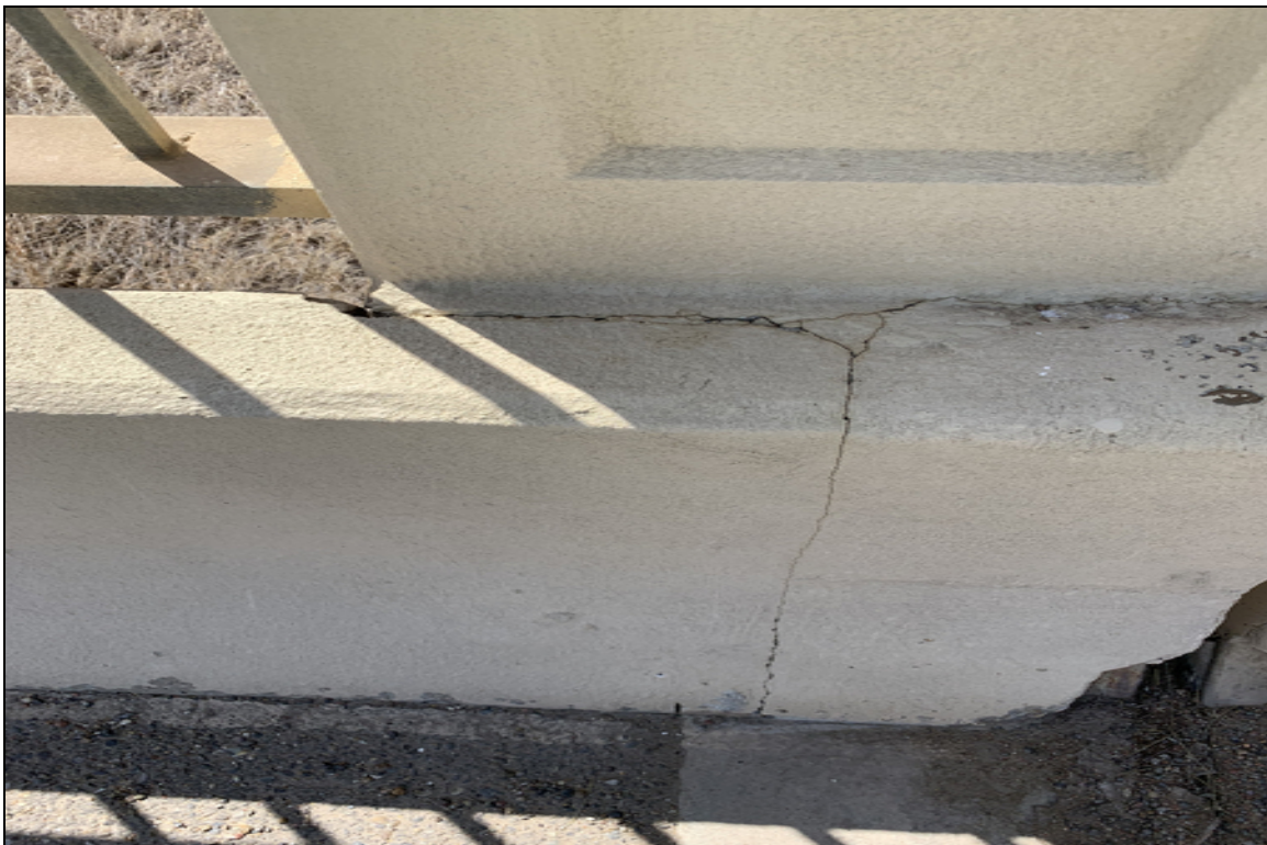
South barrier crack
