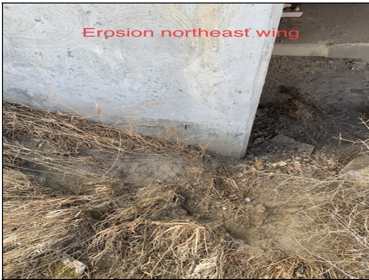
Erosion NE wing
