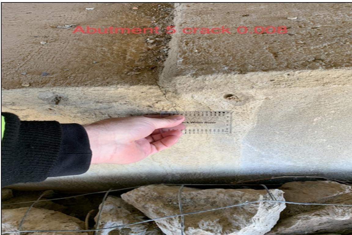
Abutment 5 cracks .008
