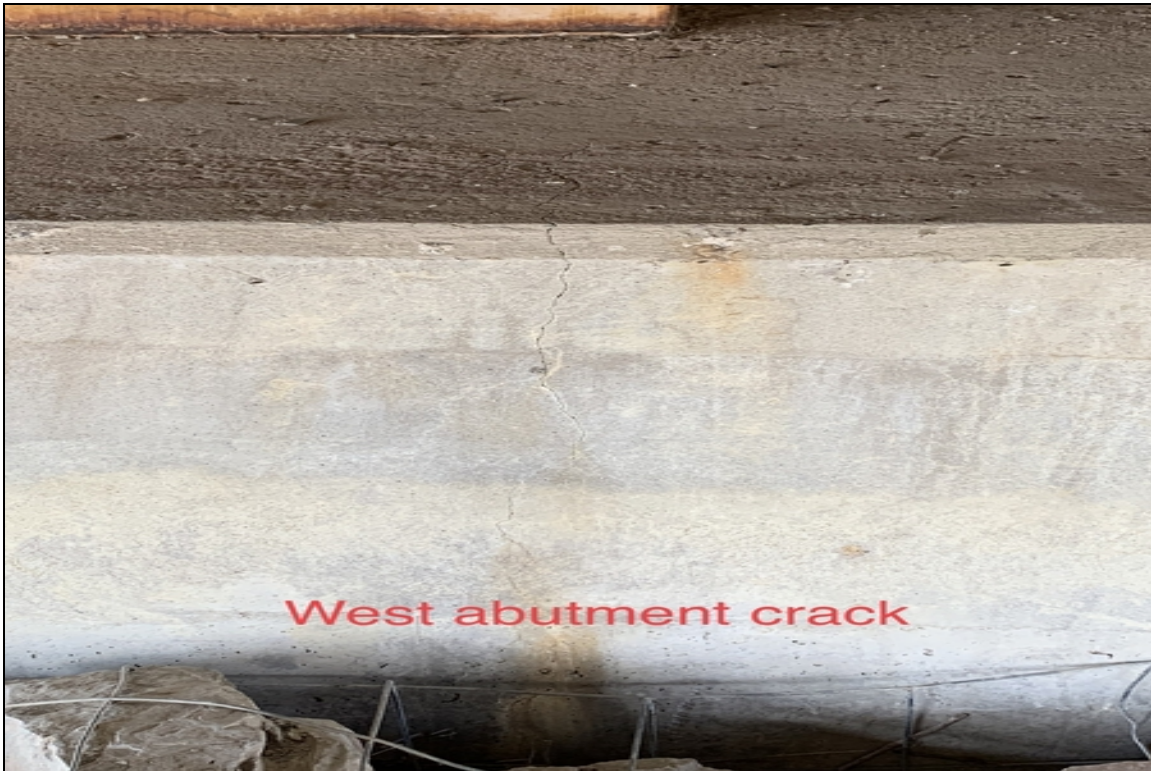
West abutment crack
