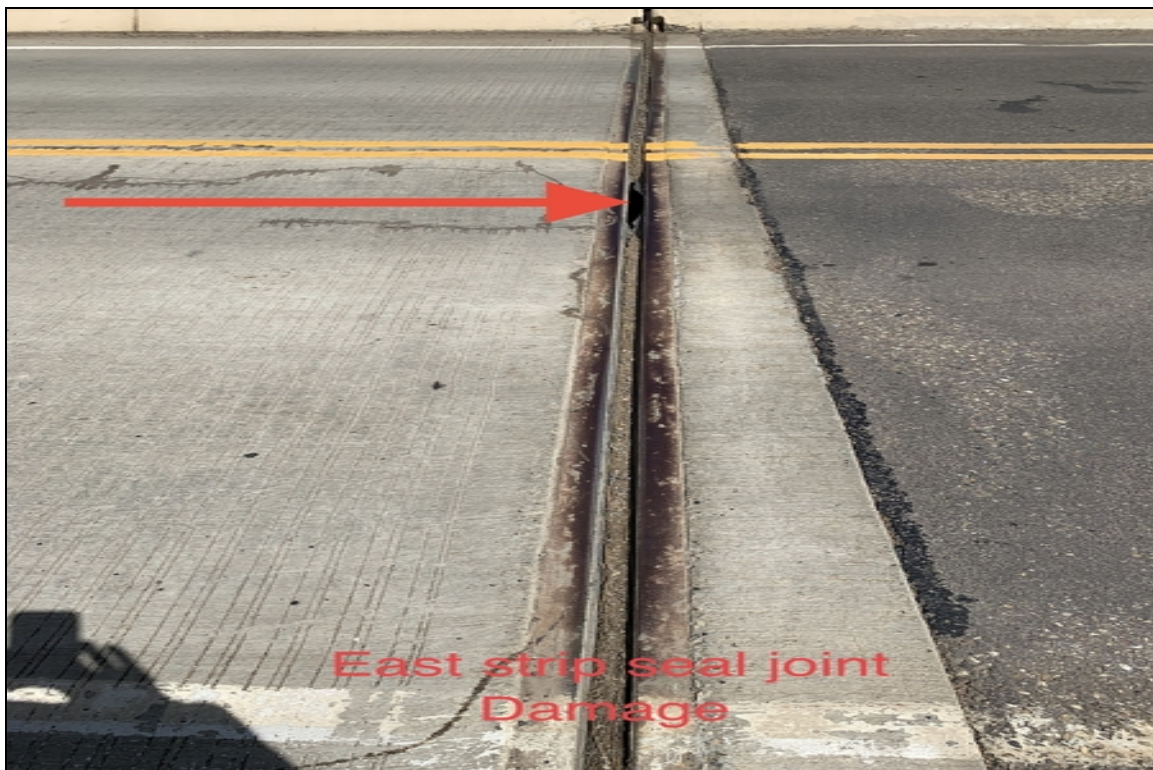
East strip seal joint damage
