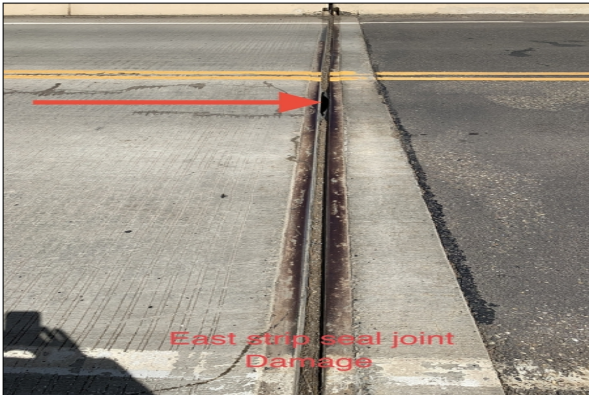
East strip seal joint damage
