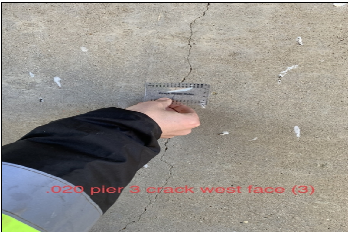
.020 pier 3 cracks
