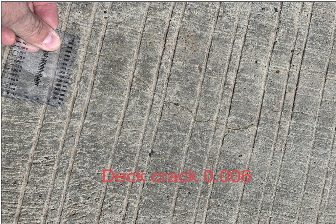
Deck crack .006
