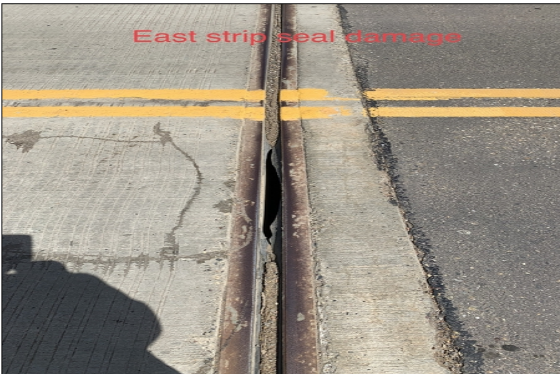
East strip seal damage
