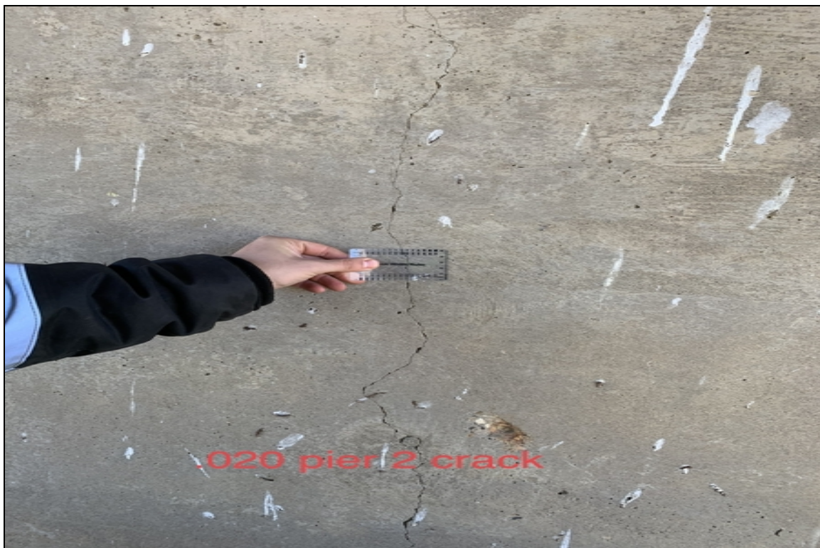
.020 pier 2 crack
