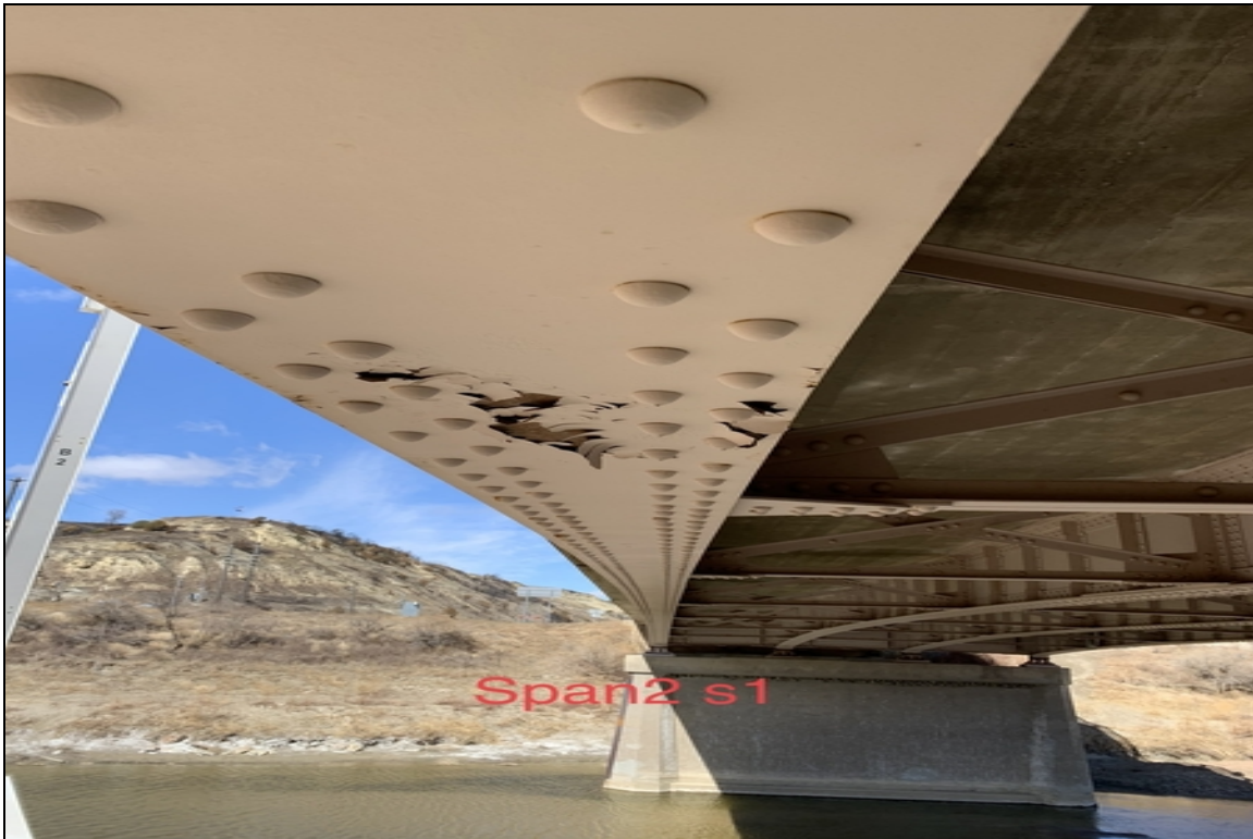
Span 2 s1 paint failure
