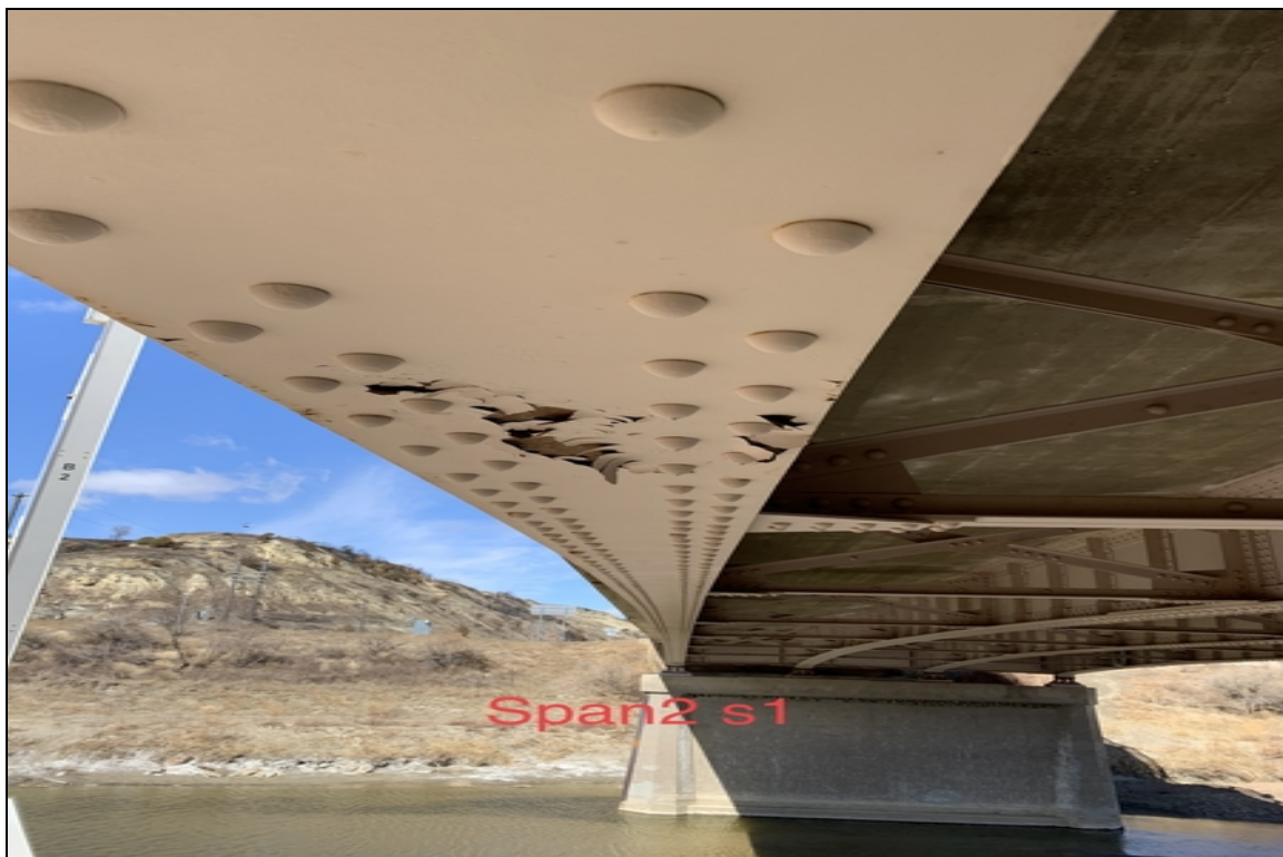
Span 2 s1 paint failure
