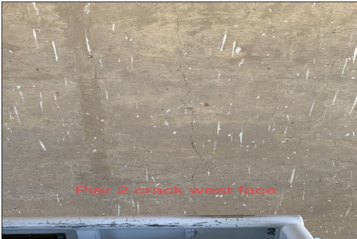
Pier 2 crack west face
