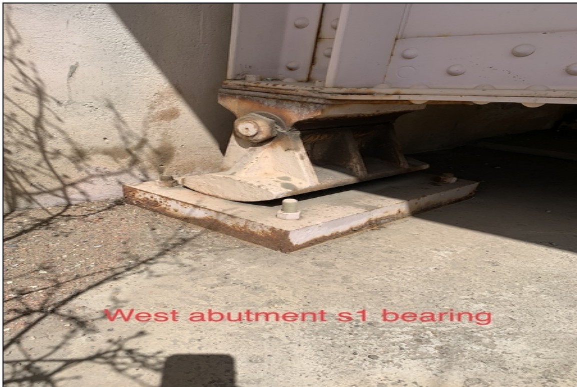
West abutment s1 bearing
