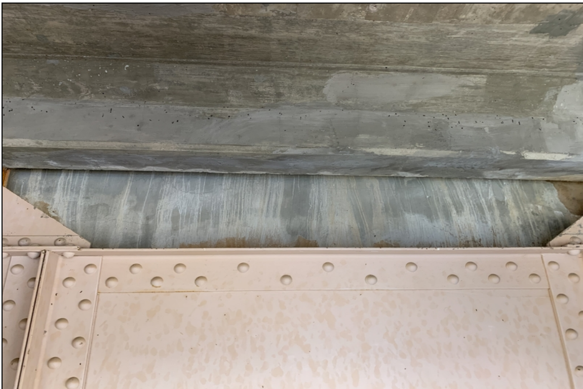
West backwall and deck lips repairs
