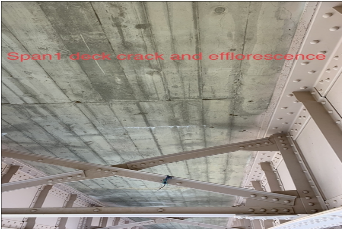
Span 1 deck crack and efflorescence
