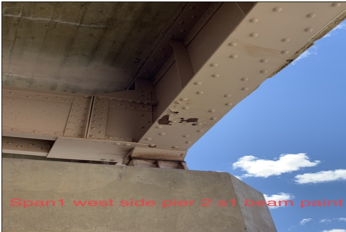
Span 1 west side pier 2 s1 beam paint failure
