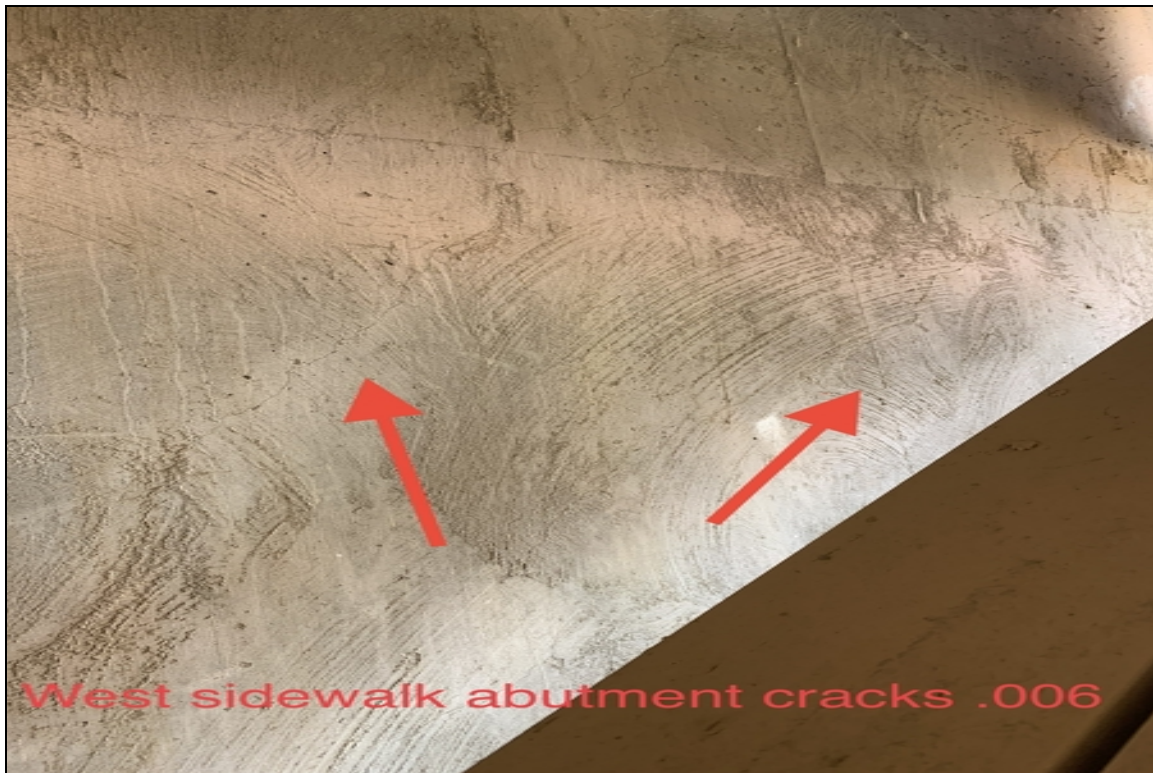
West sidewalk abutment cracks .006
