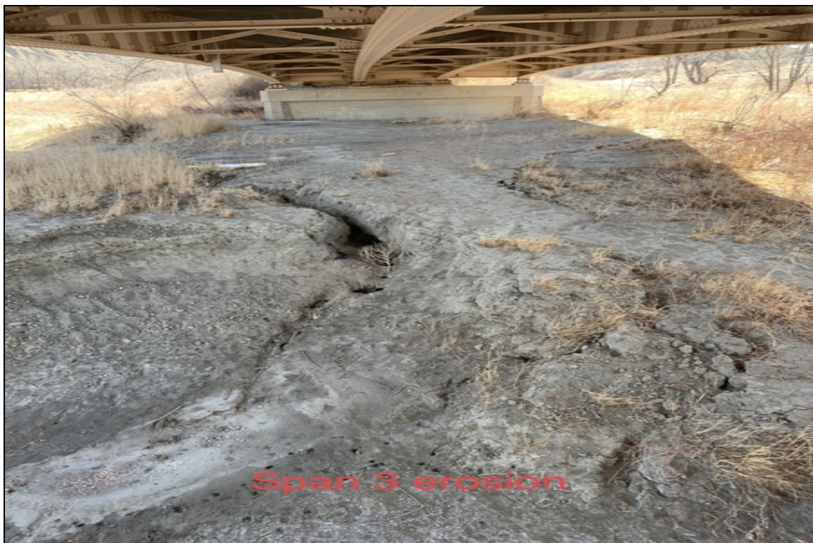
Span 3 erosion
