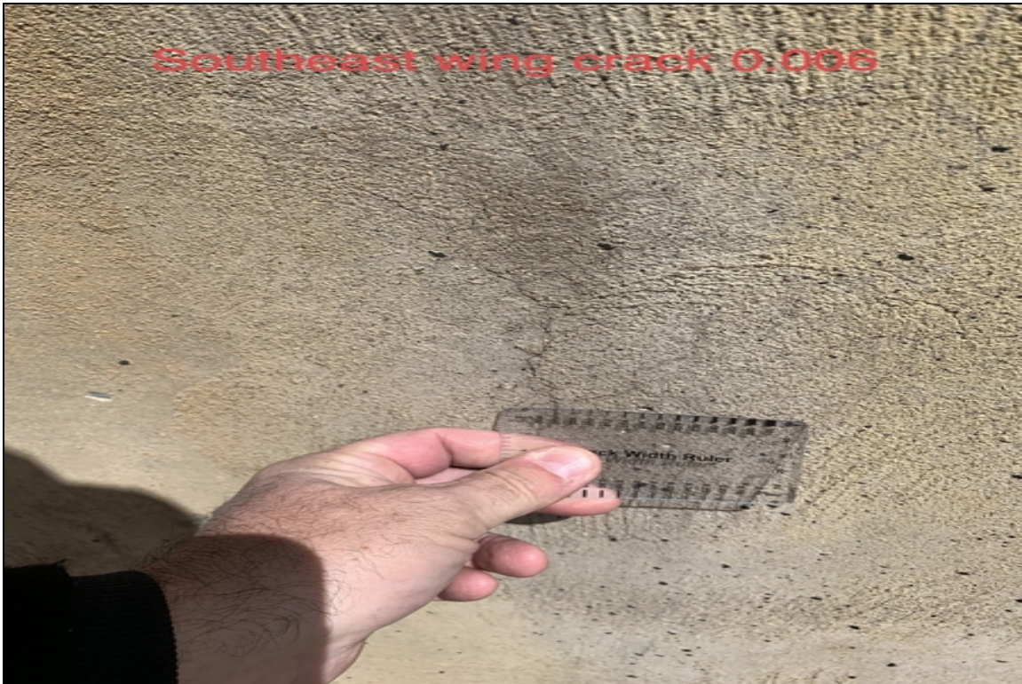
SE wing crack .006
