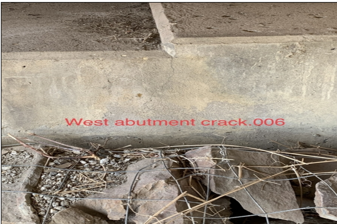
West abutment crack .006
