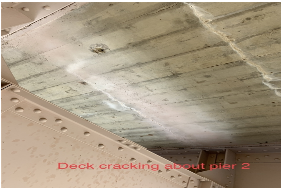
Deck cracking above pier 2 with small pop out
