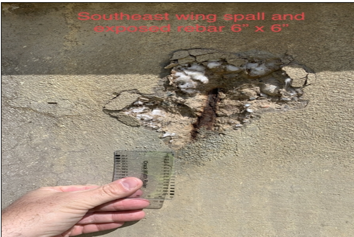
SE wing spall and exposed rebar 6"x6"
