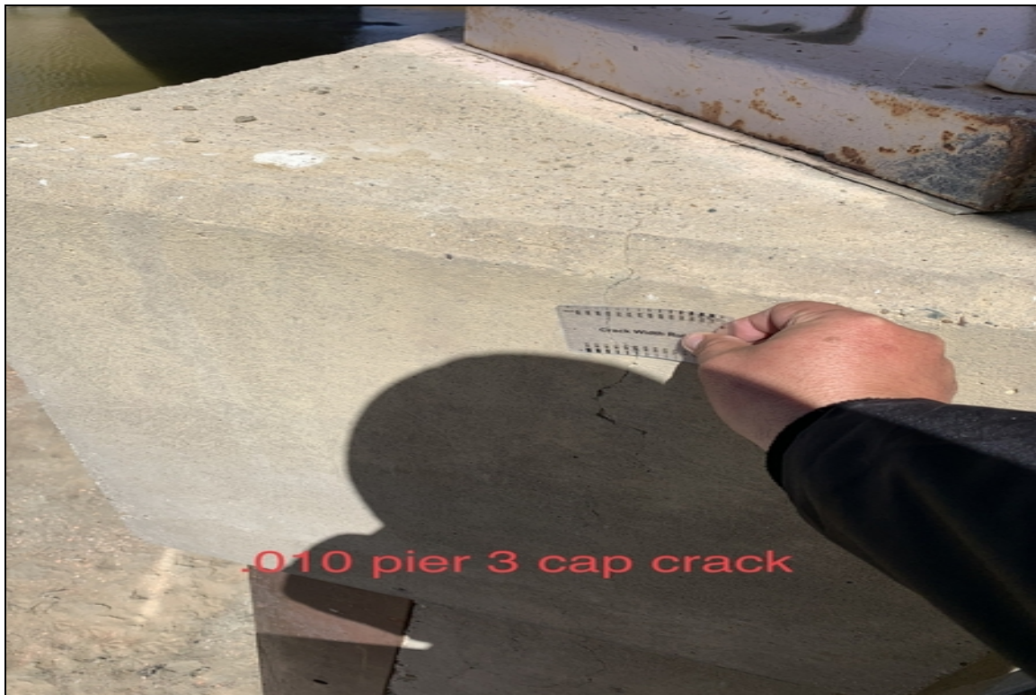
.010 pier 3 cap crack
