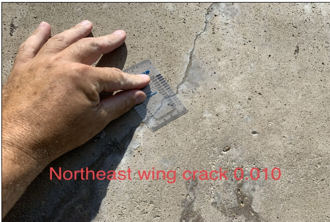
NE wing crack .010
