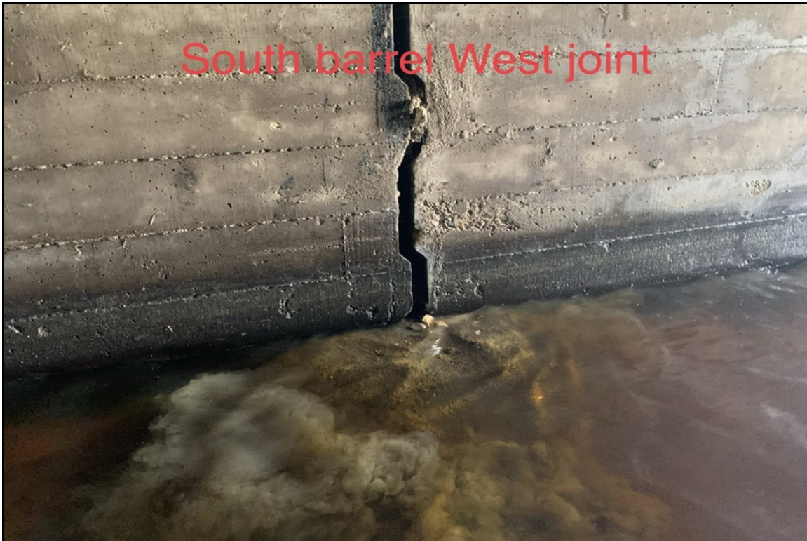
South barrel west joint fill loss
