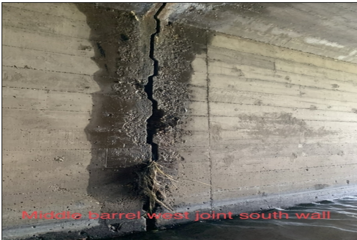
Middle barrel west joint south wall
