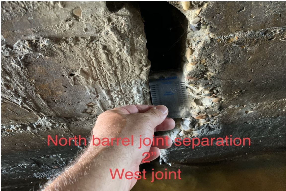
North barrel joint separation 2" west joint
