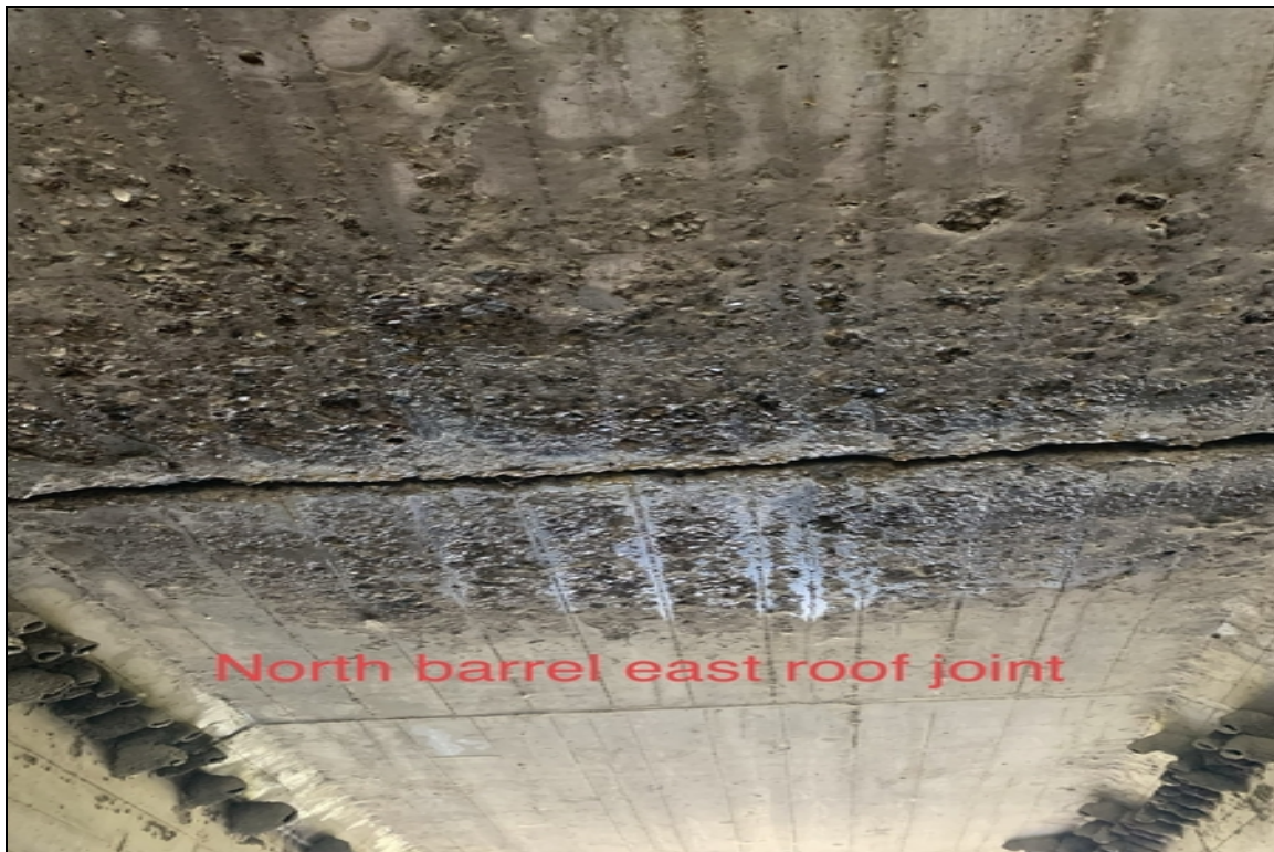
North barrel east roof joint
