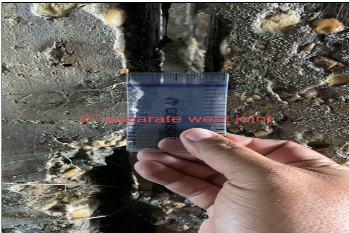
2" separation west joint
