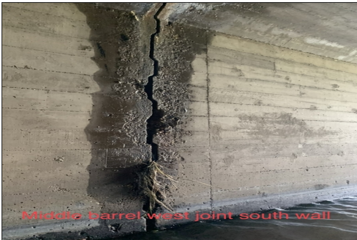
Middle barrel west joint south wall
