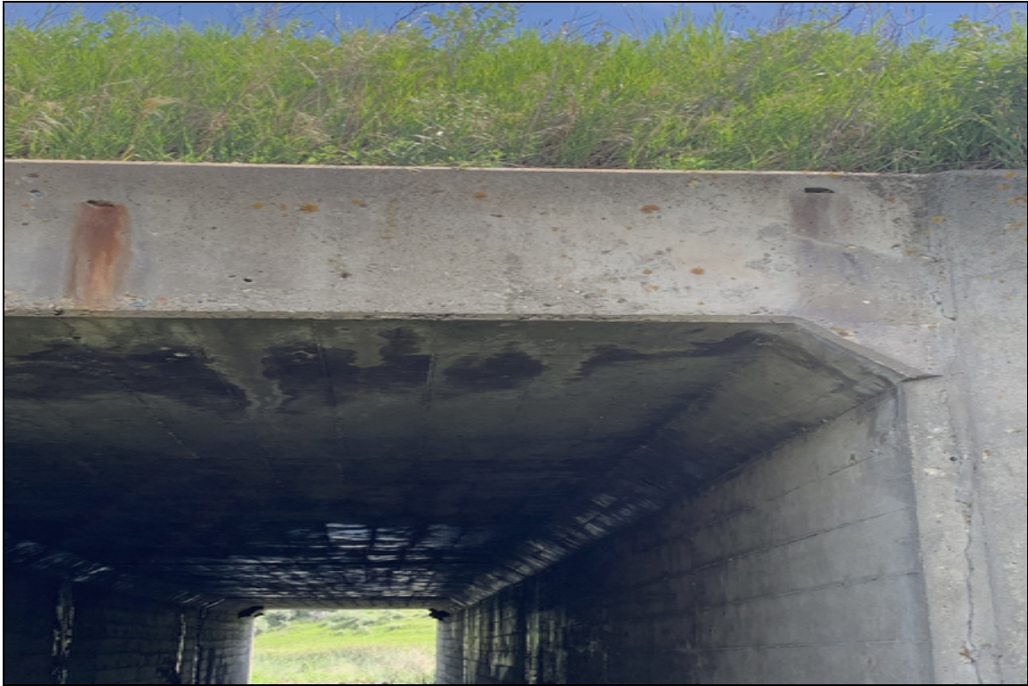
South headwall crack
