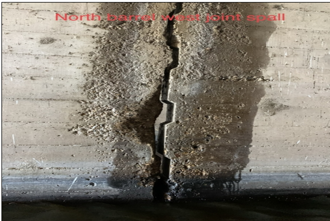
North barrel west joint spall
