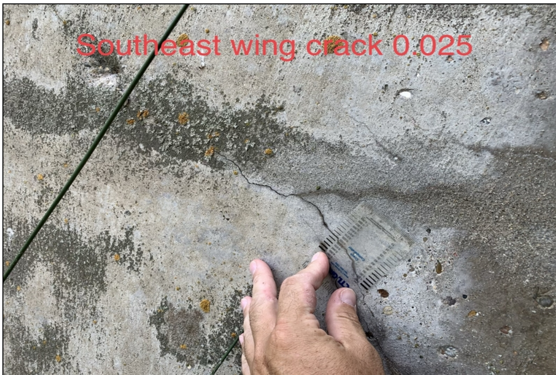
SE wing crack .025
