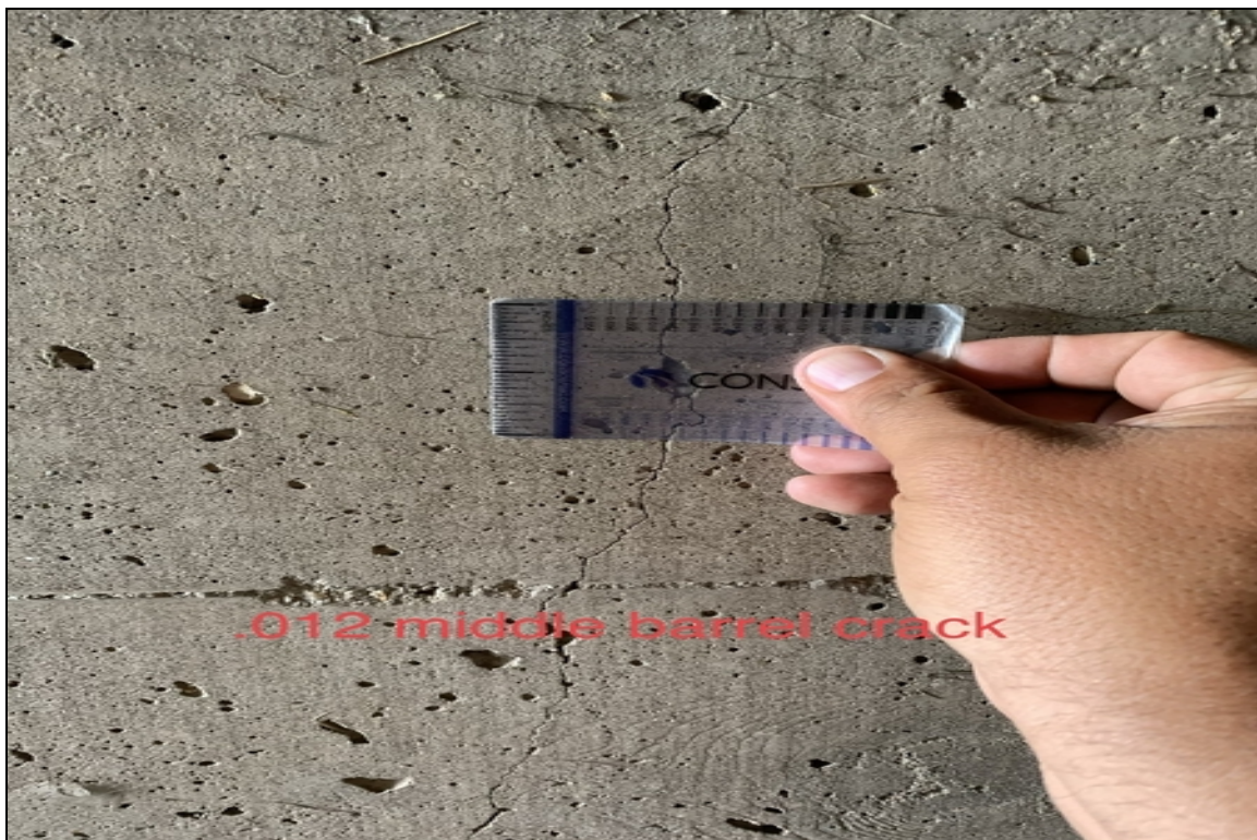
.012 middle barrel crack
