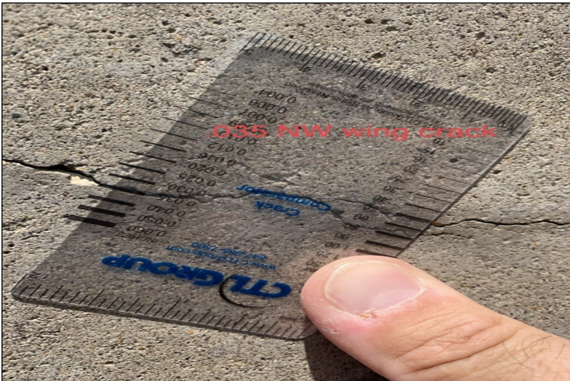
.035 NW wing crack
