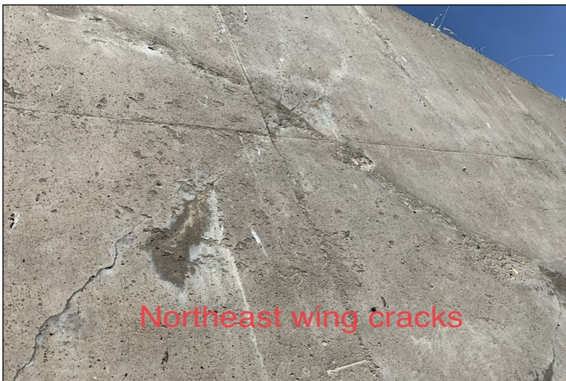
NE wing cracks
