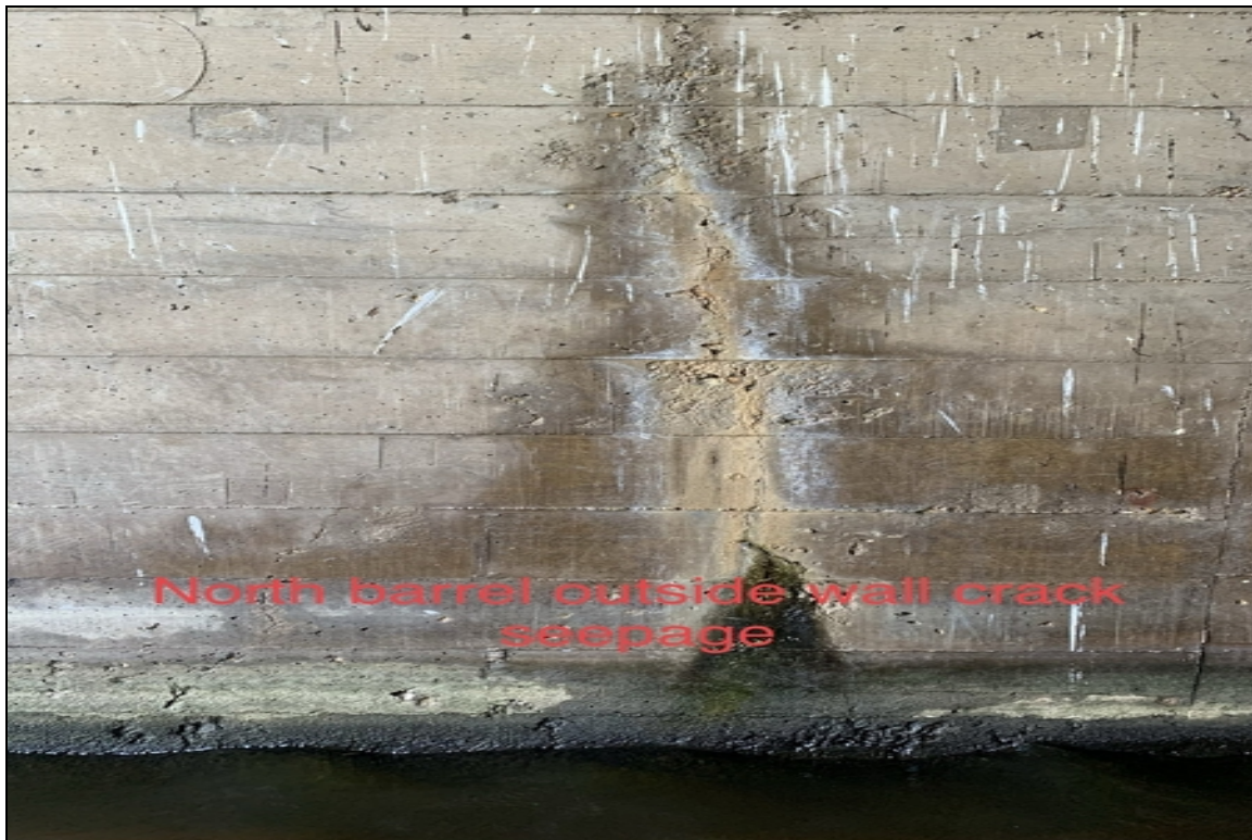
North barrel outside wall crack and seepage
