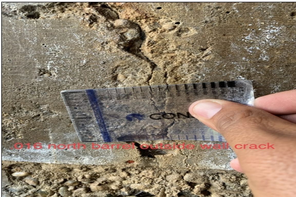
.016 north barrel outside wall crack
