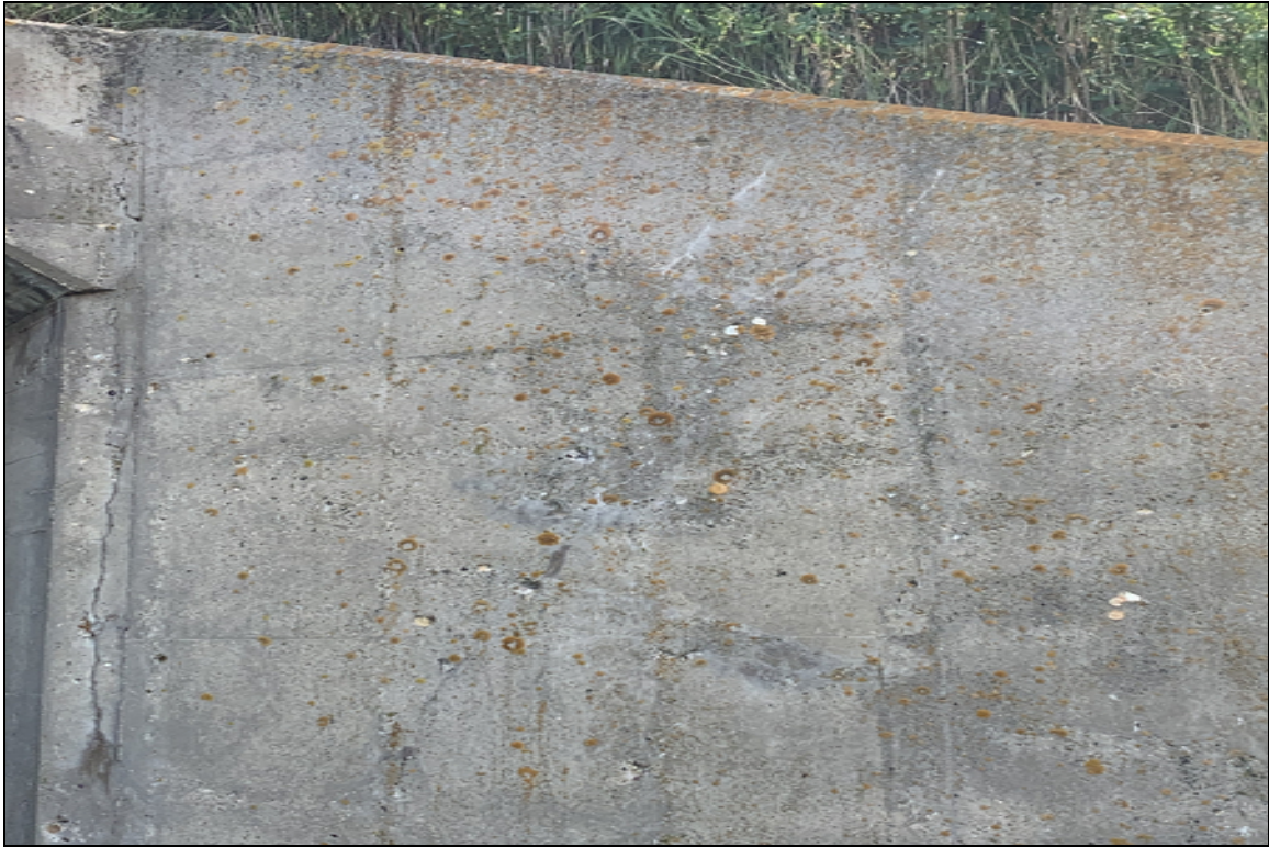
SW wing crack
