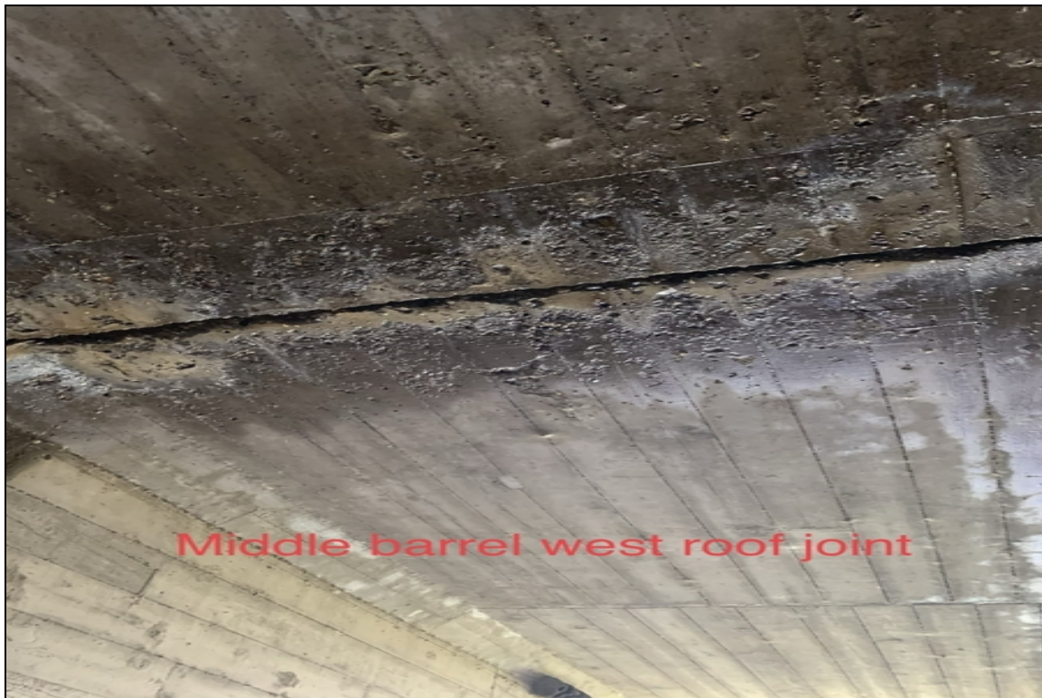
Middle barrel west roof joint
