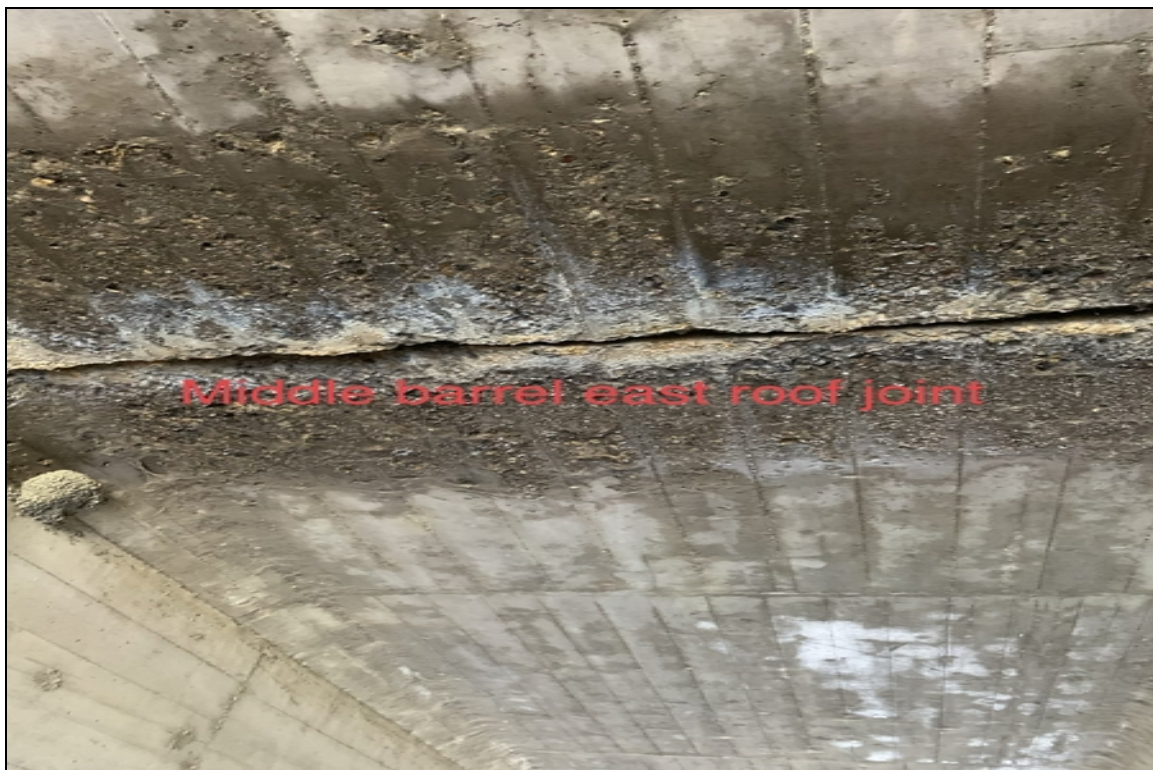
Middle barrel east roof joint
