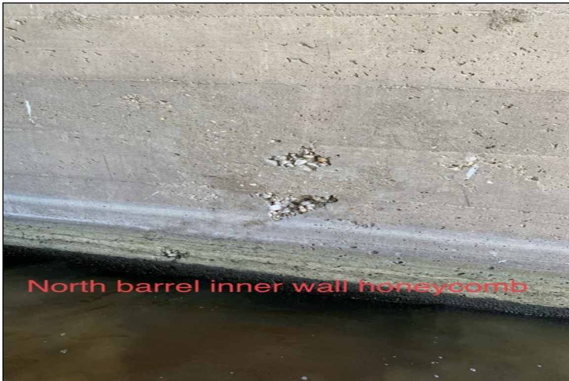
North barrel inner wall honeycomb
