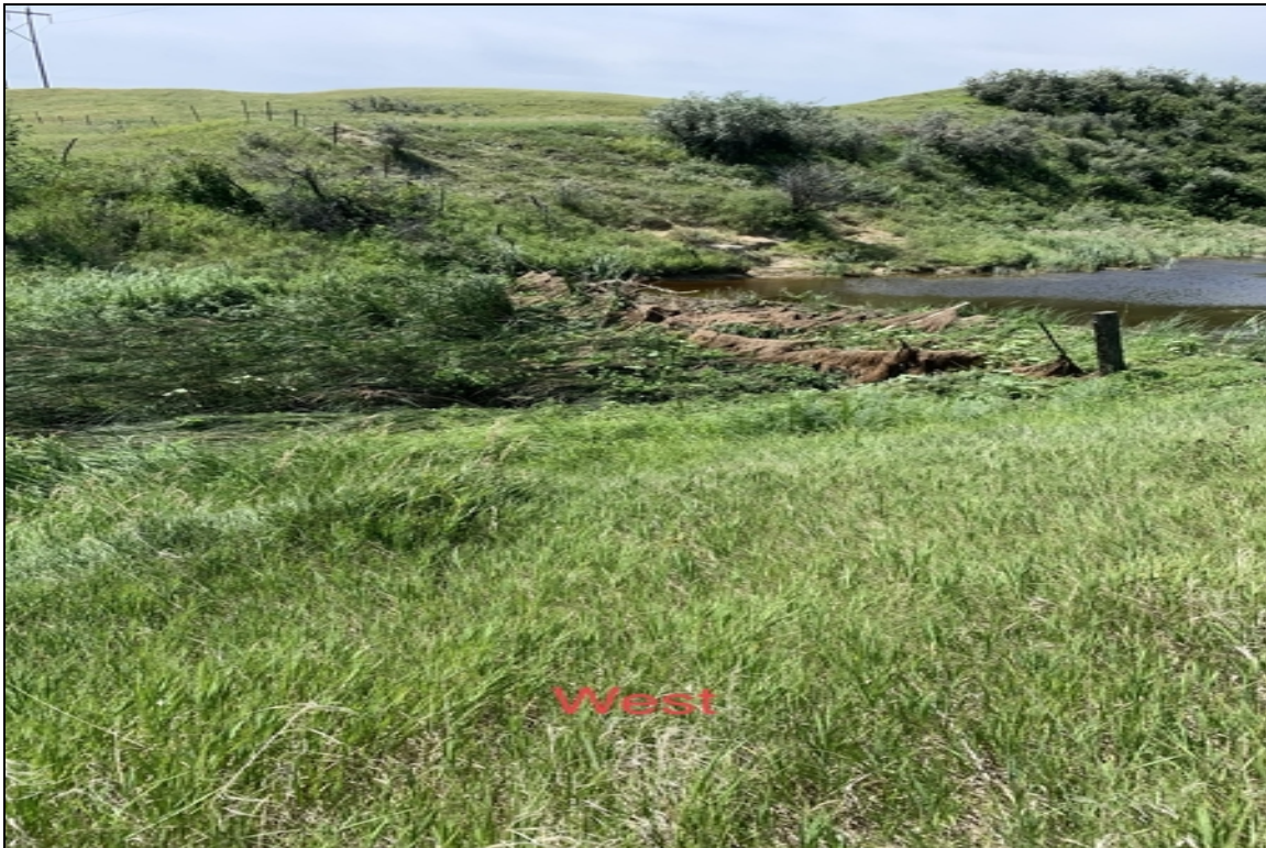
West side earthen dam build up
