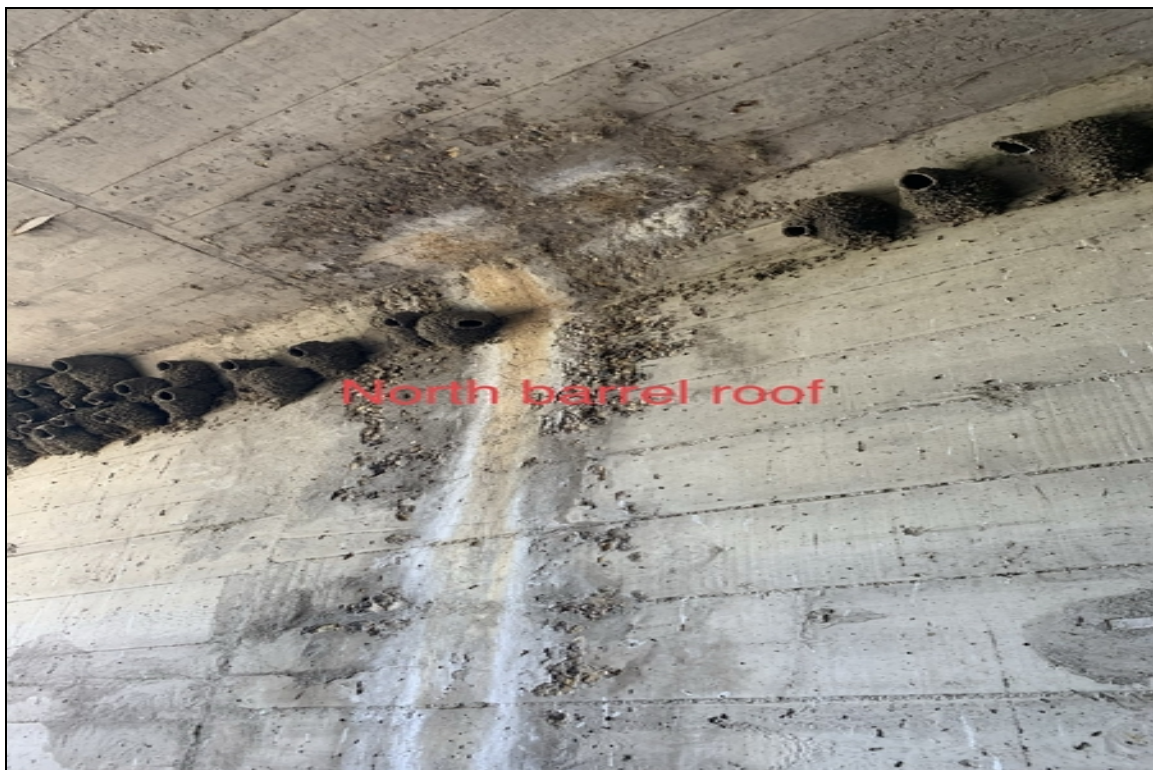
North barrel roof
