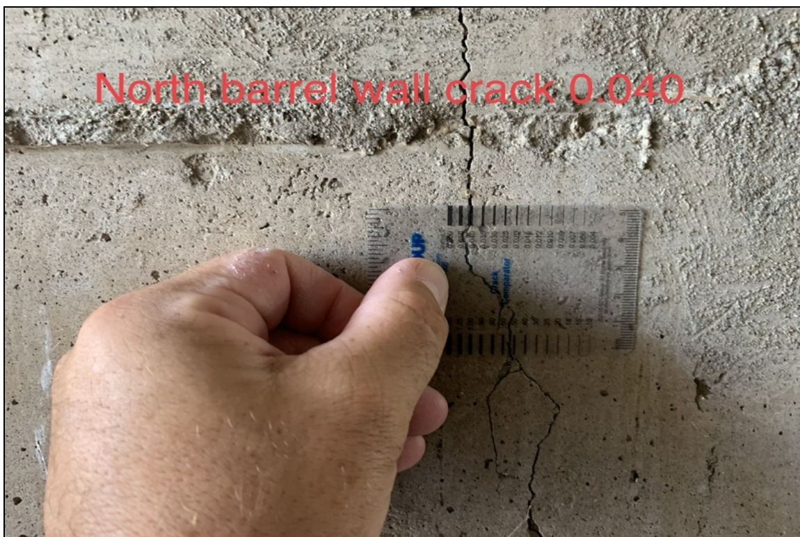
.040 north barrel crack
