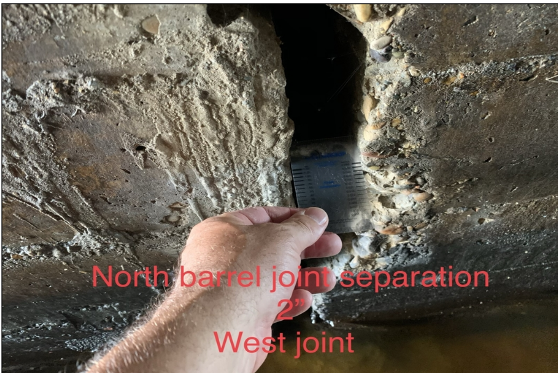
North barrel joint separation 2" west joint
