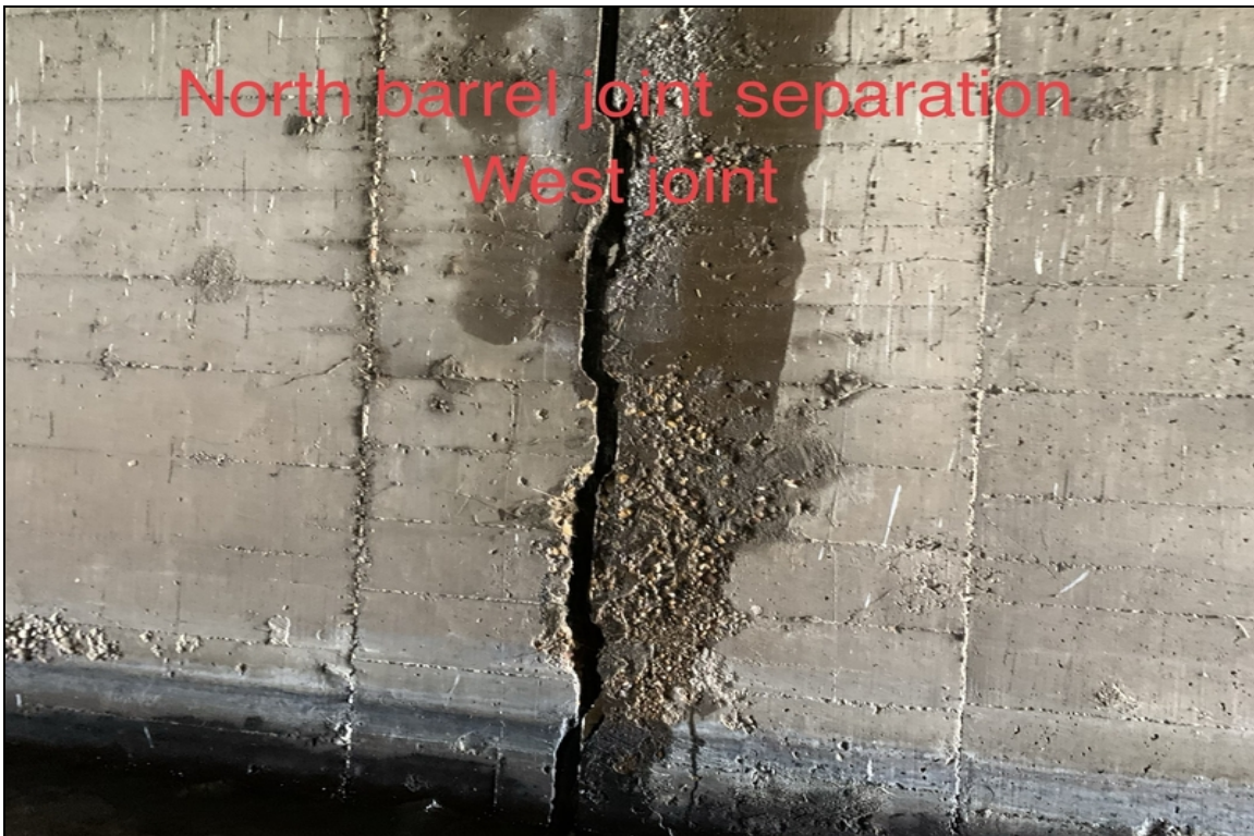
North barrel joint separation west joint
