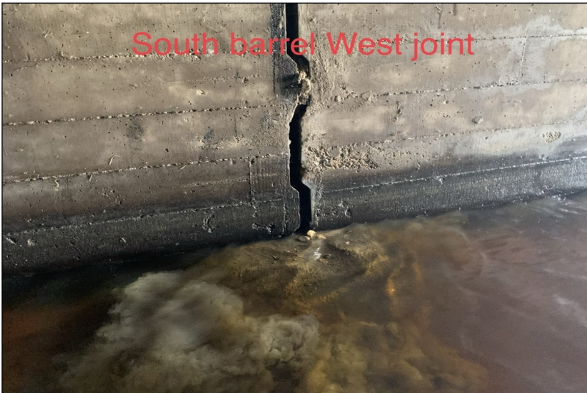
South barrel west joint fill loss
