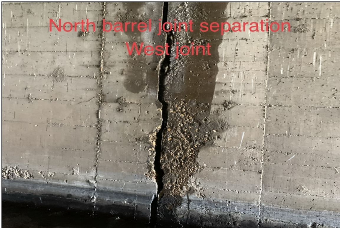
North barrel joint separation west joint
