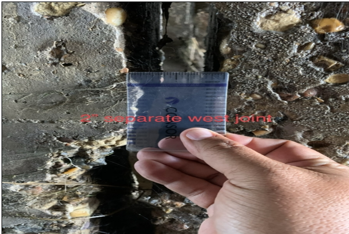
2" separation west joint
