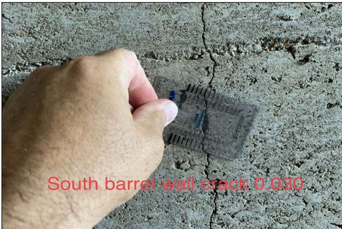
South barrel crack .030
