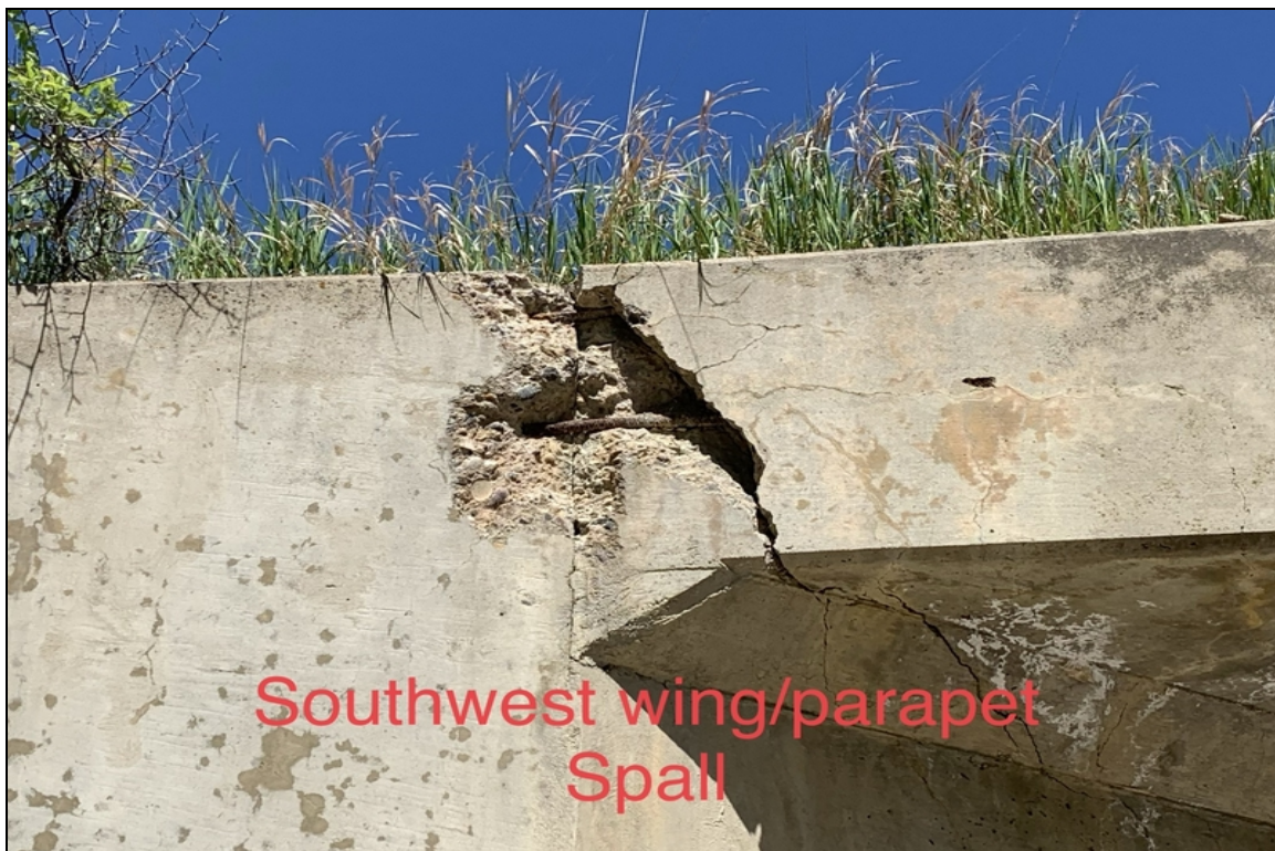
SW wing and parapet spall exposed rebar
