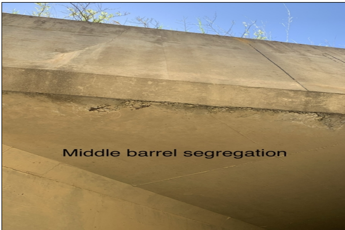
Middle barrel segregation under east headwall exposed rebar
