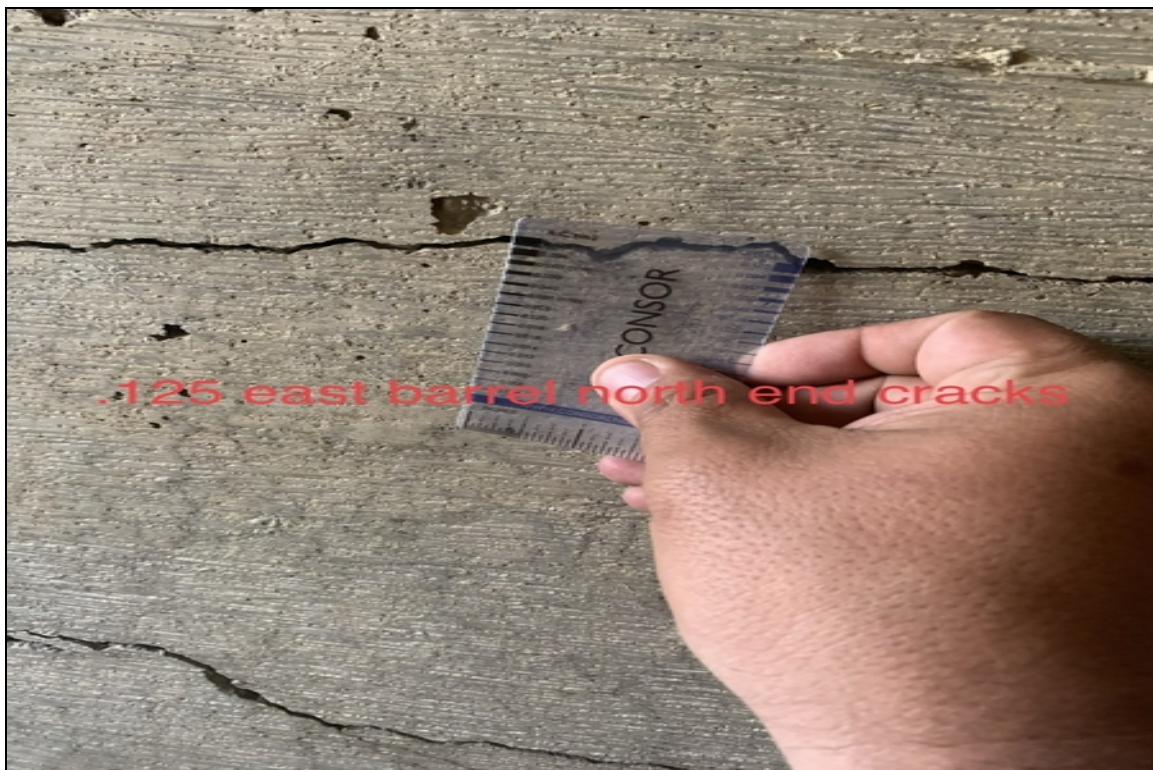
.125 east barrel outside wall crack north end
