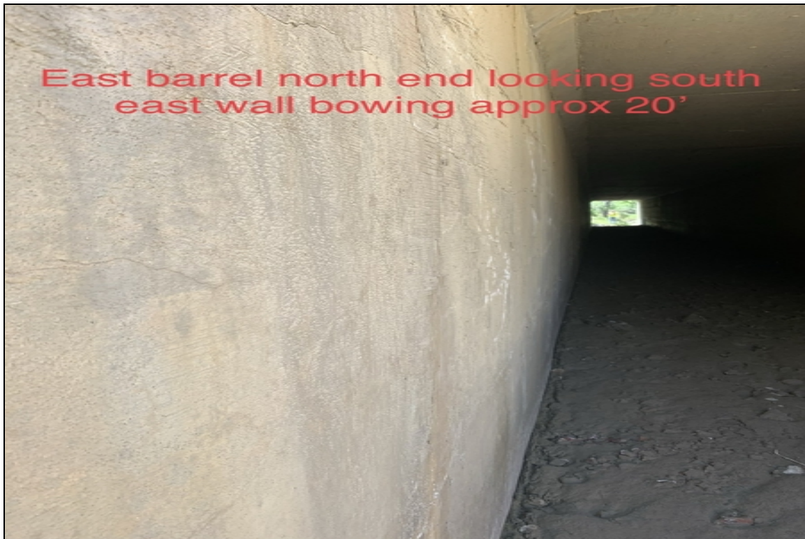
East barrel north end looking south wall bowing approx 20"
