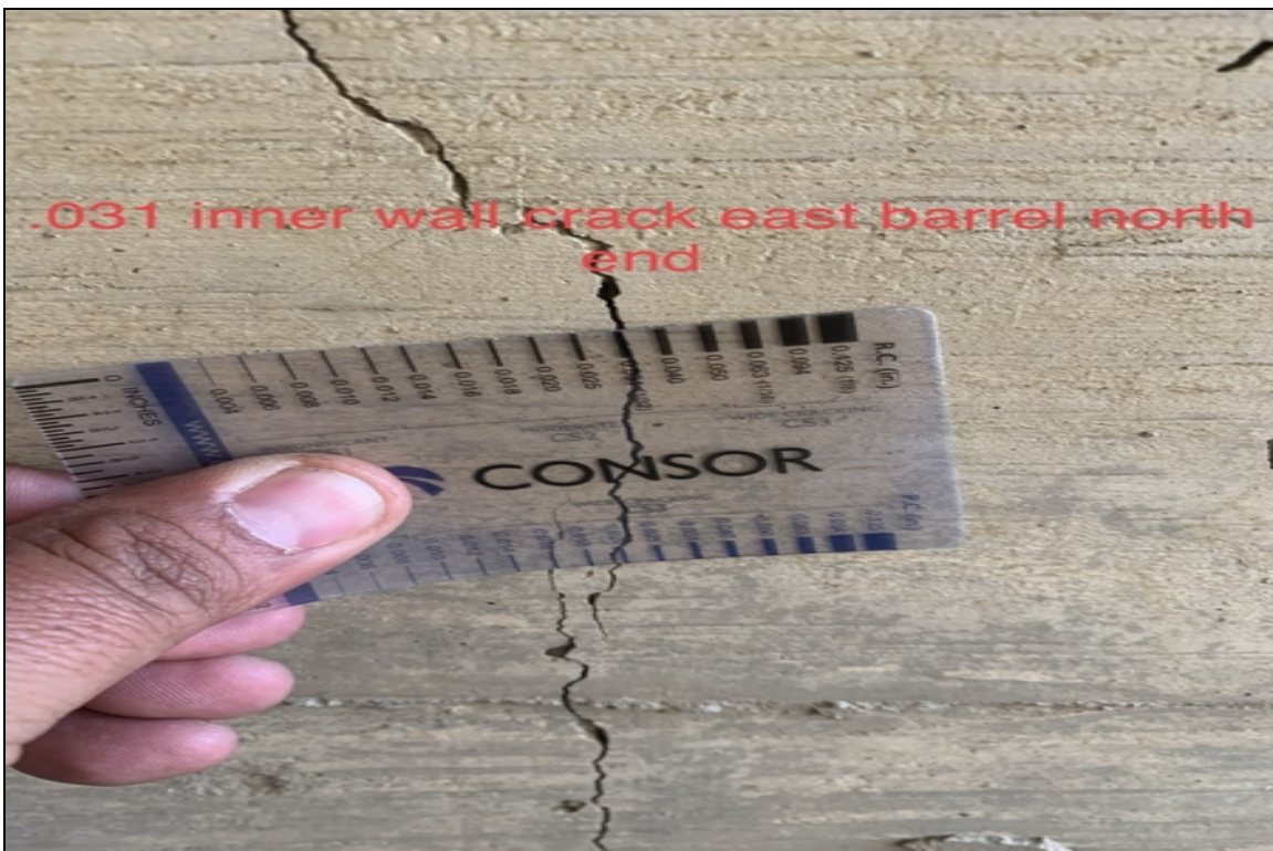
.031 inner wall crack east barrel north end
