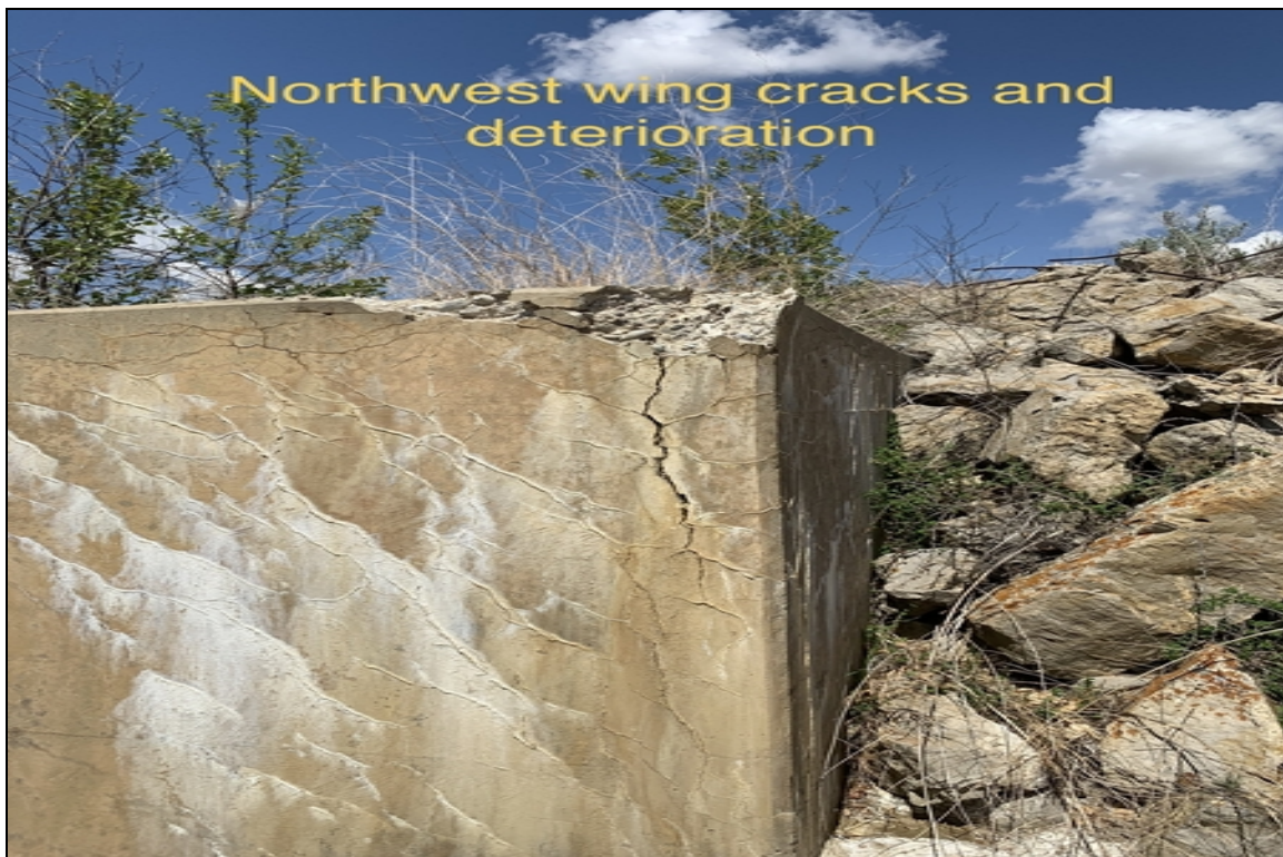
NW wing cracks and deterioration
