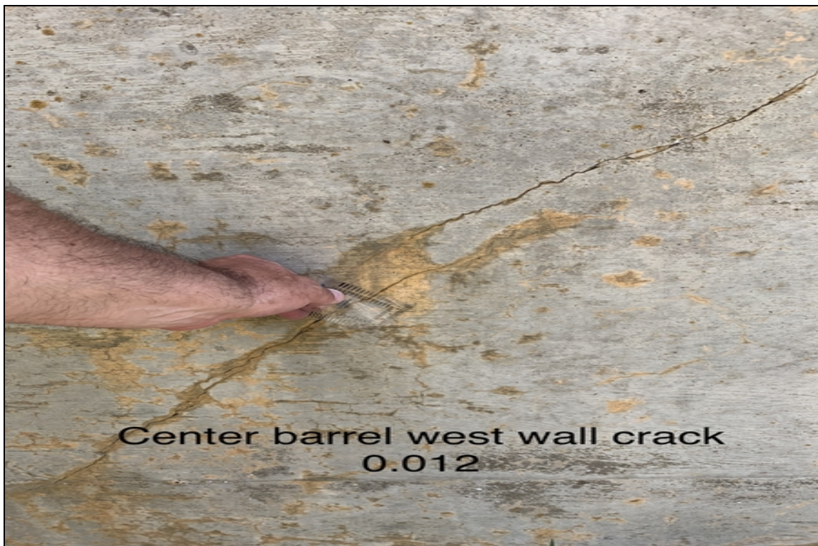
Center barrel west wall crack .012
