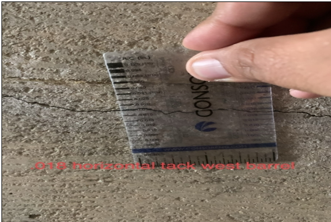
.018 horizontal crack west barrel outside wall
