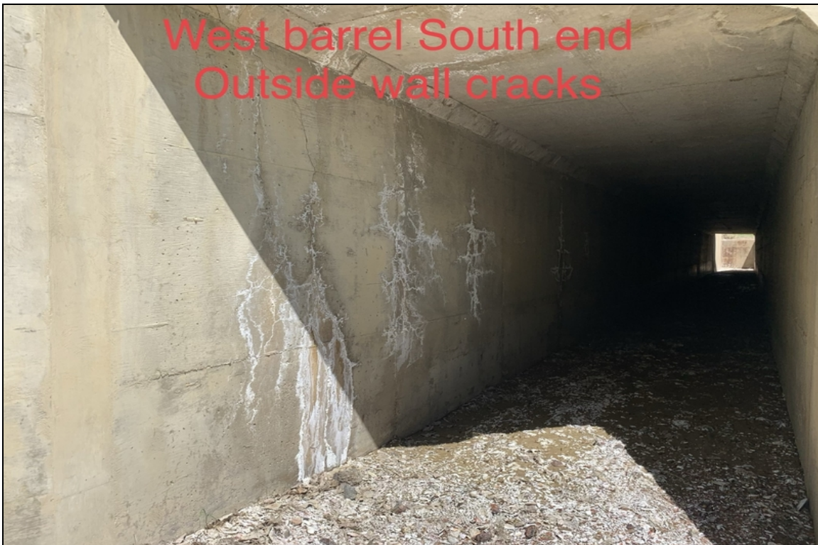
West barrel south end outside wall cracks
