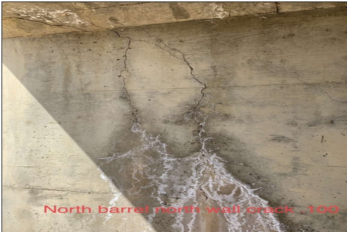
West barrel north wall crack .100 Not north
