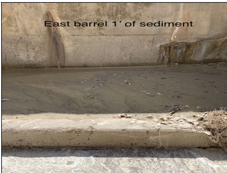
East barrel 1' sediment
