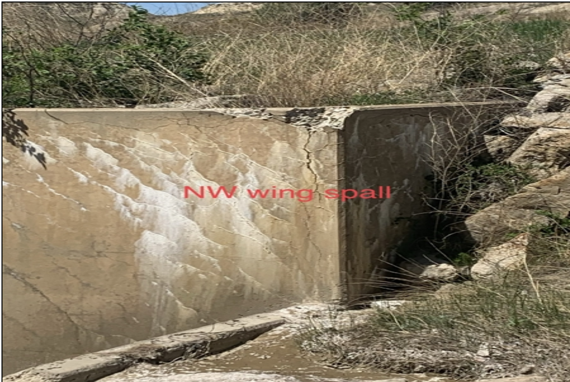
NW wing spall
