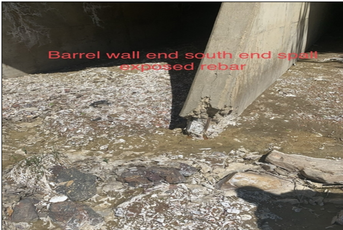
Bagel wall end south spill exposed rebar
