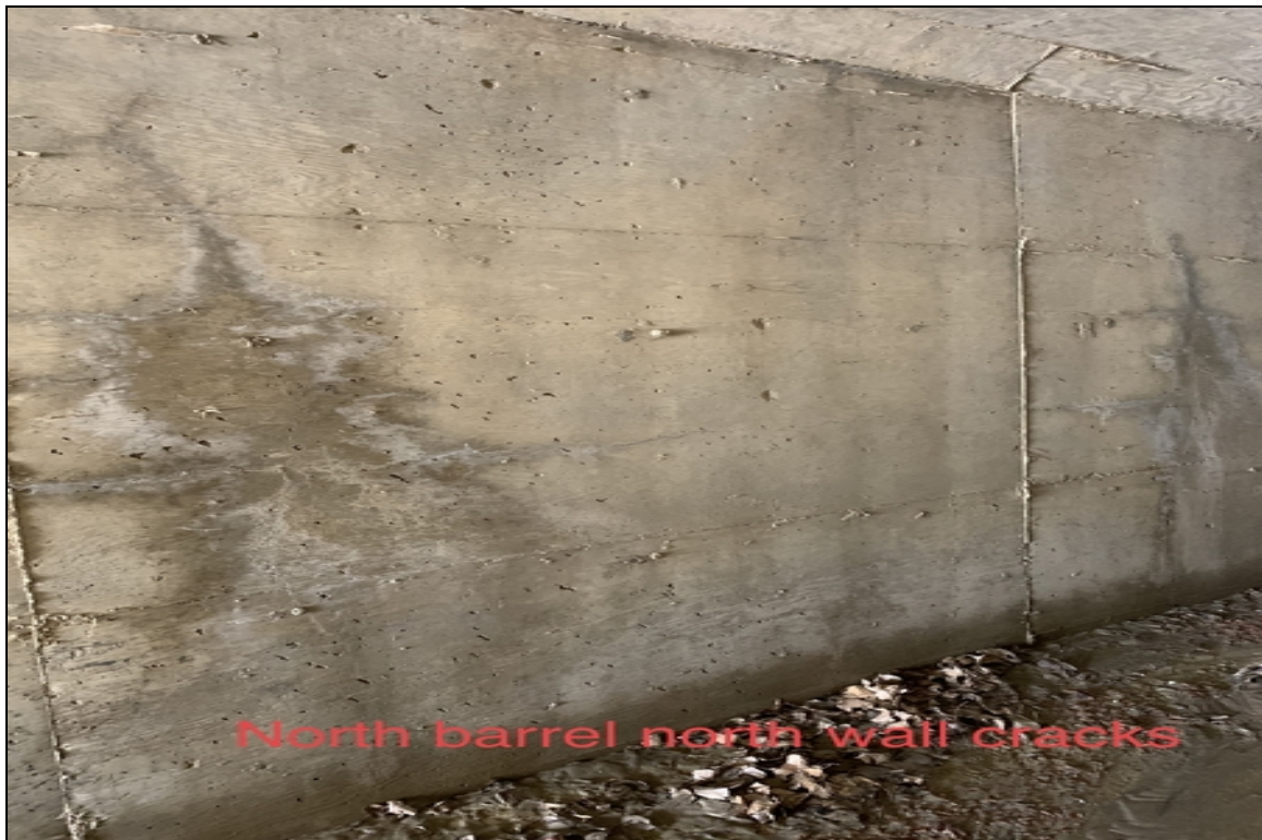
West barrel north wall cracks Not north barrel
