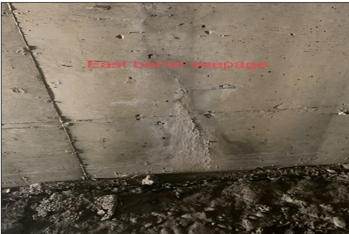
East barrel outside wall seepage
