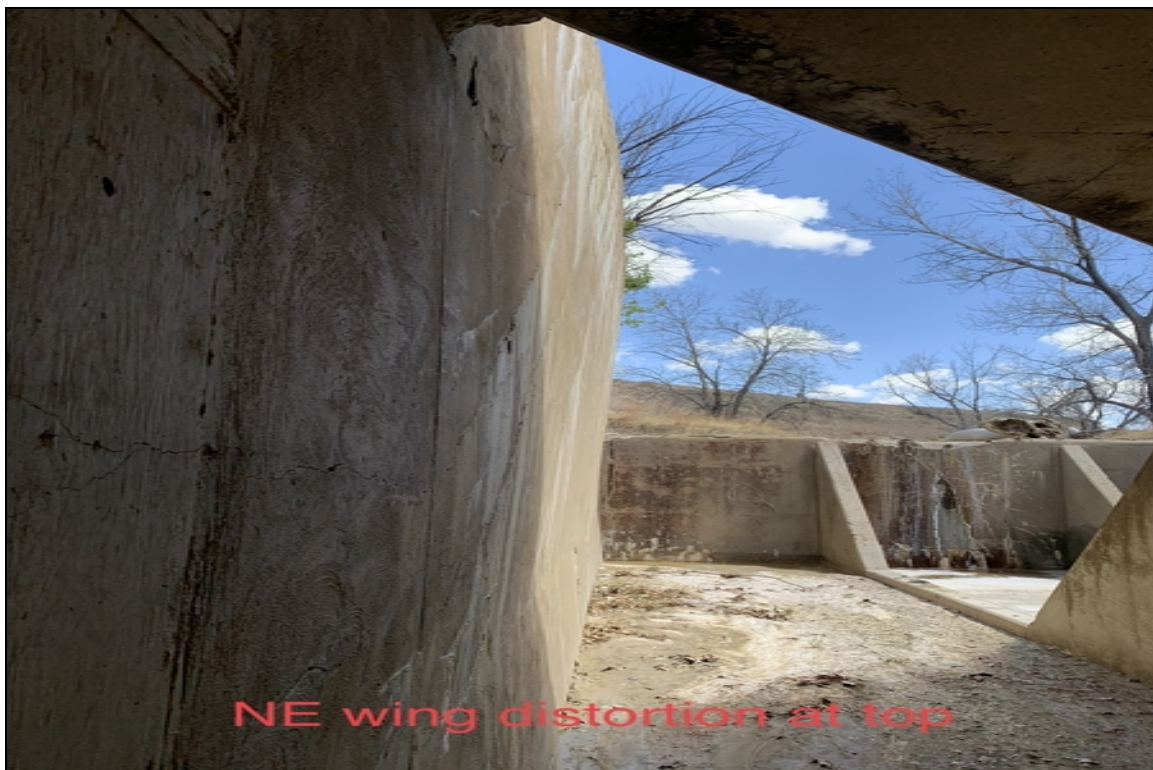
NW wing distortion at top Not NE
