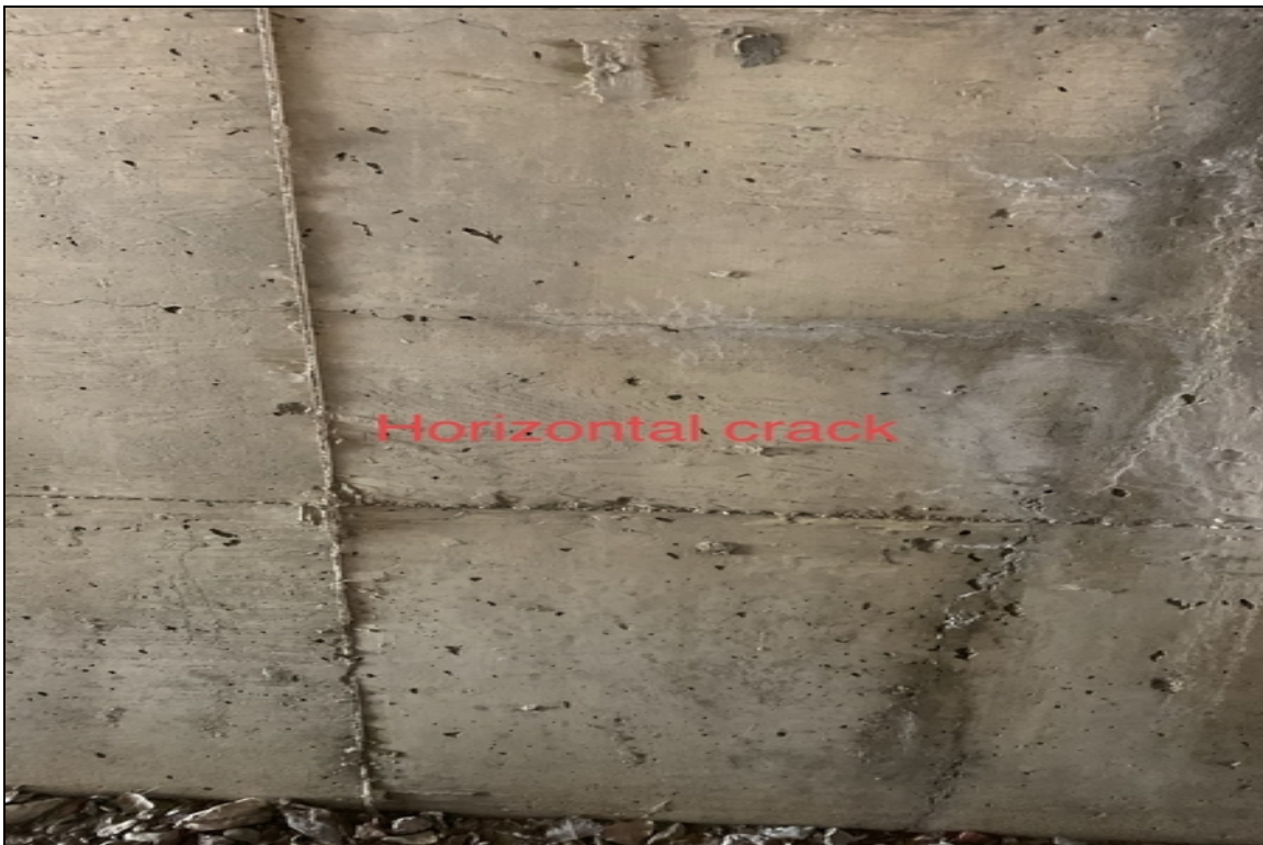
Horizontal cracks west outside wall south end
