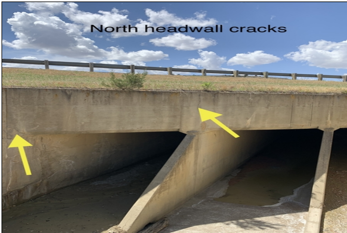
North headwall cracks
