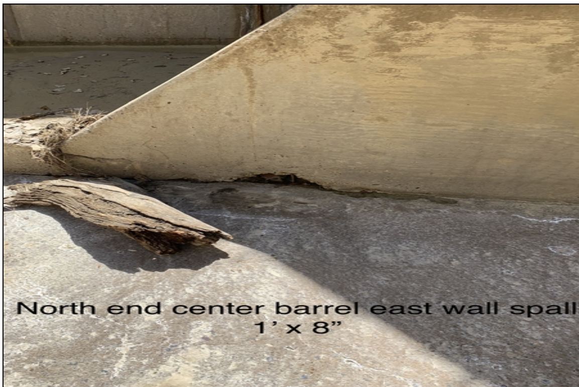
North end center barrel east wall spall 1'x8"
