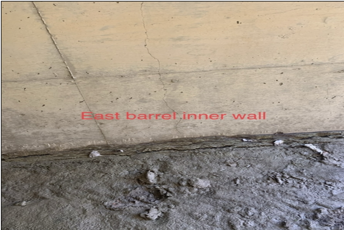
East barrel inner wall crack
