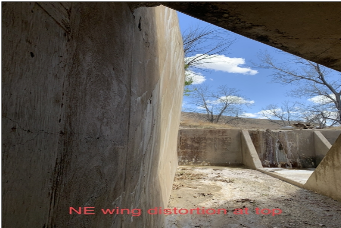
NW wing distortion at top Not NW
