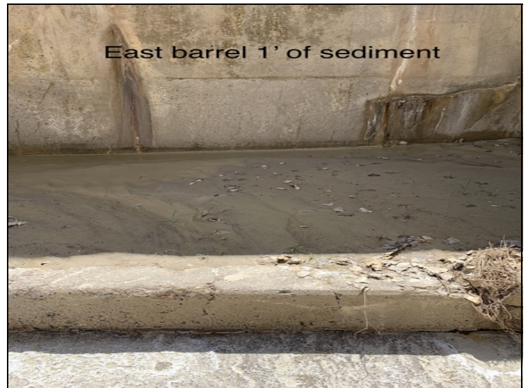
East barrel 1' sediment
