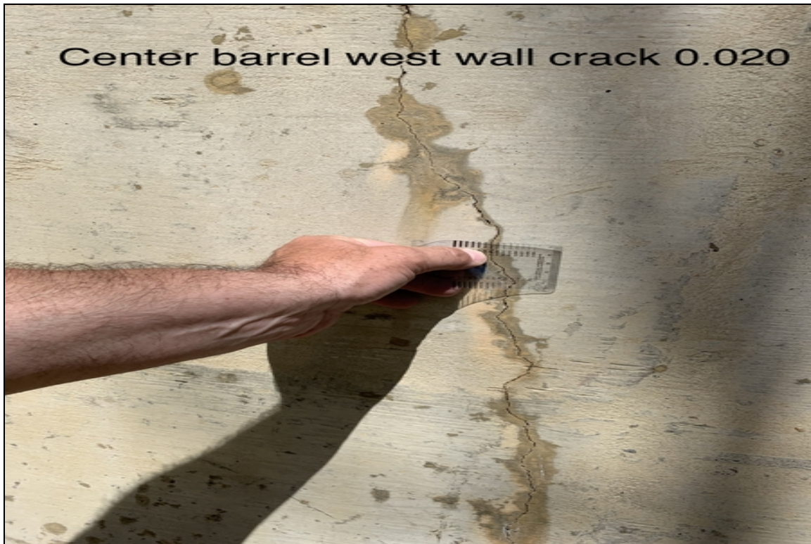
Center barrel west wall crack .020
