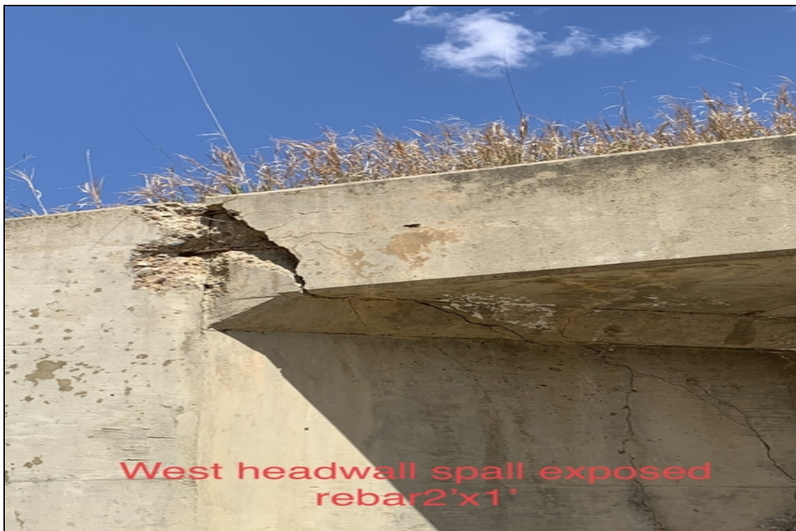
South headwall spall exposed rebar 2'x1'
