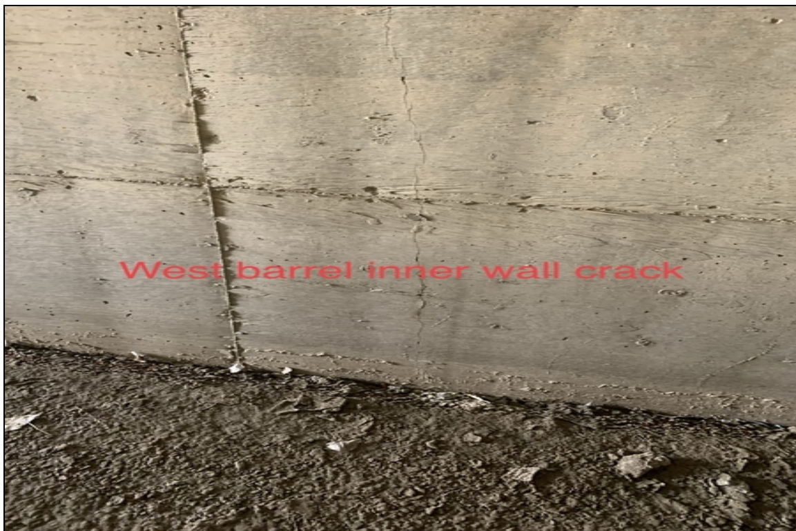
West barrel inner wall crack
