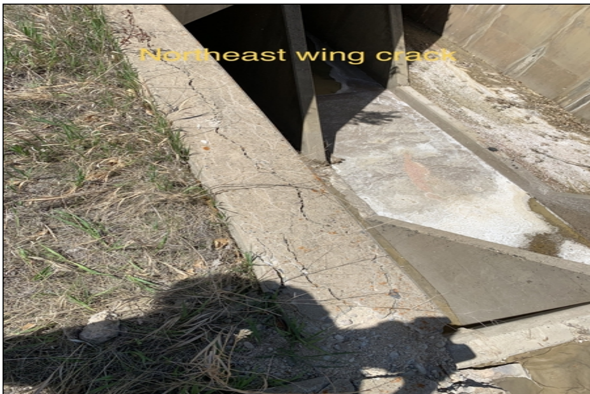
NE wing cracks
