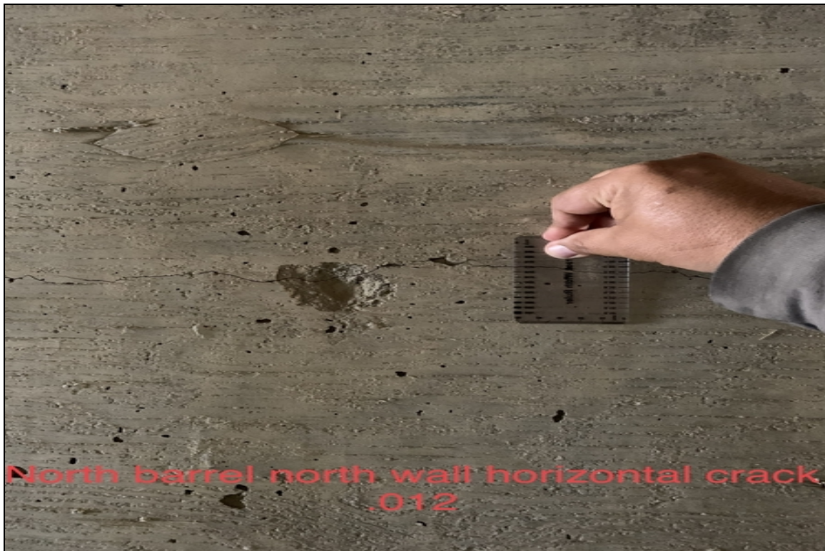
West barrel north wall horizontal crack .012 Not north barrel
