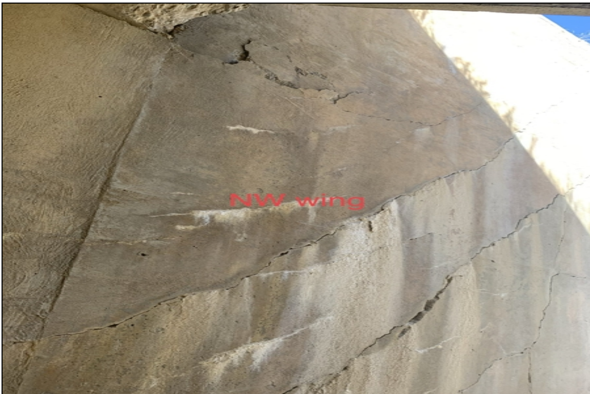
NW wing cracks
