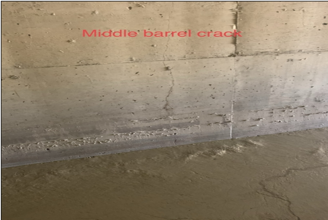
Middle barrel crack
