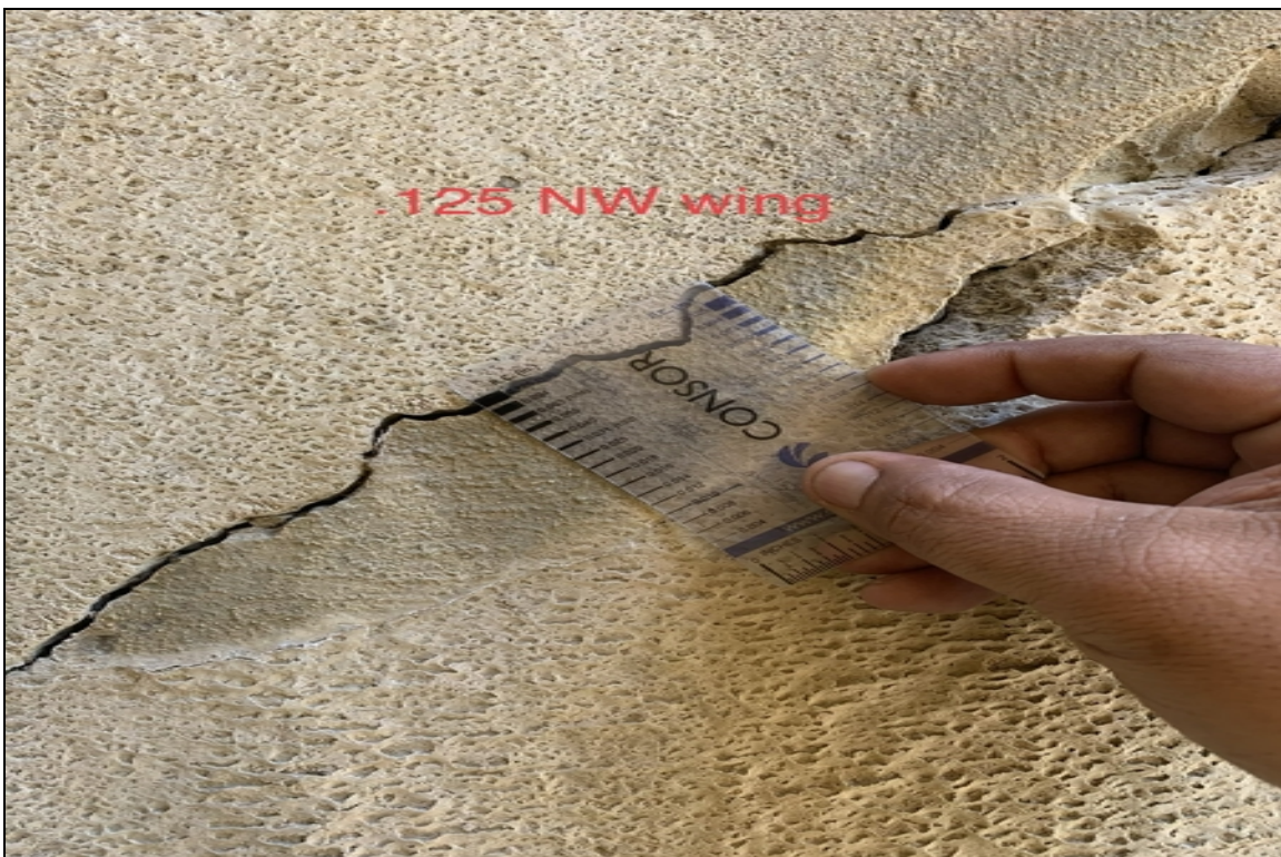
.125 NW wing crack
