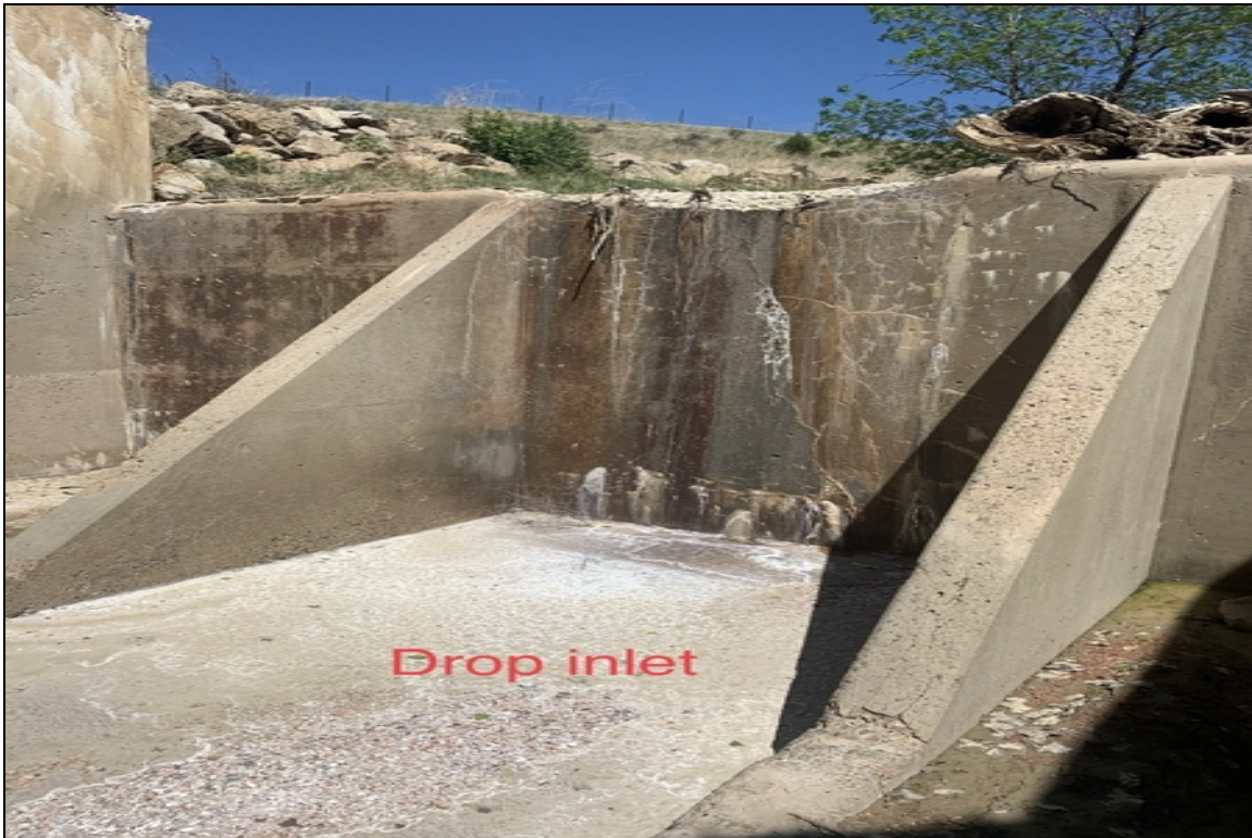
Drop inlet cracking
