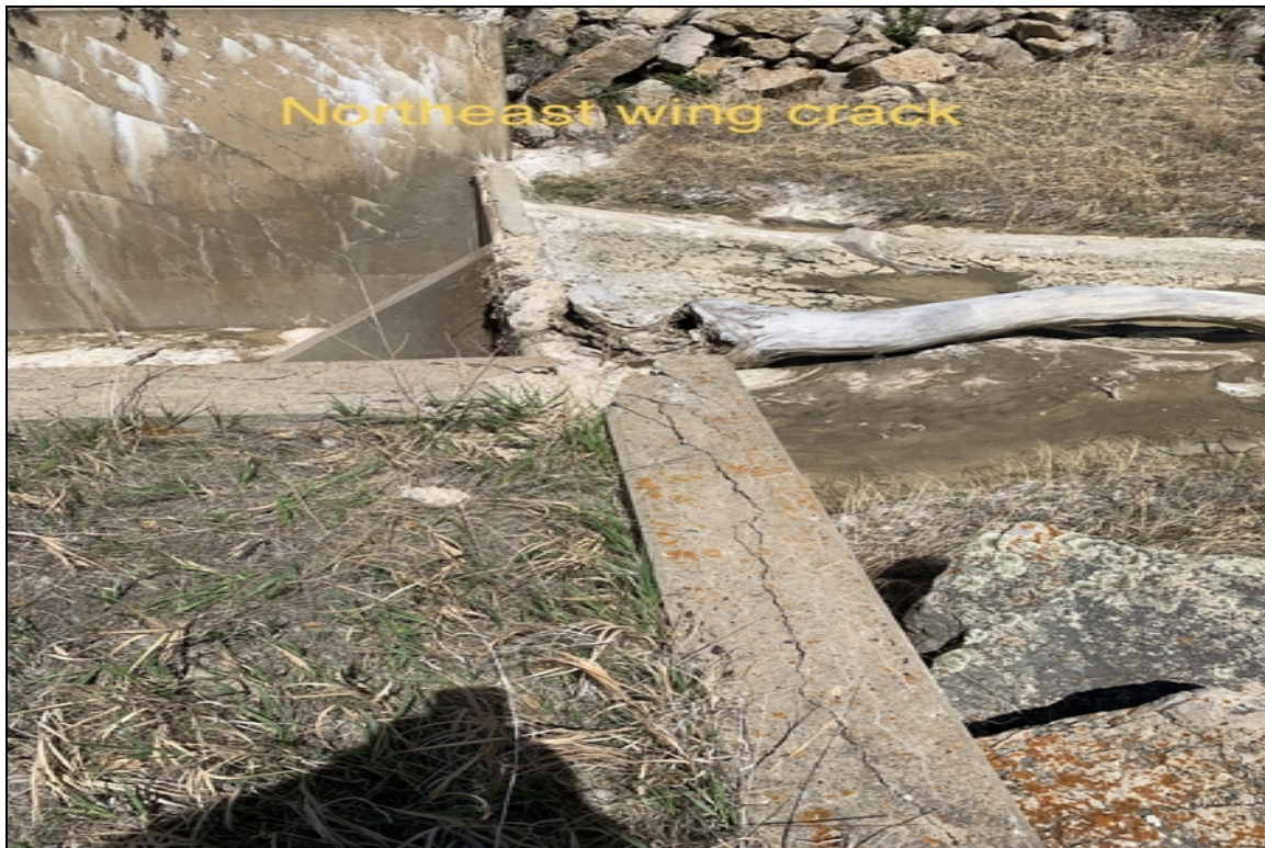
NE wing cracks
