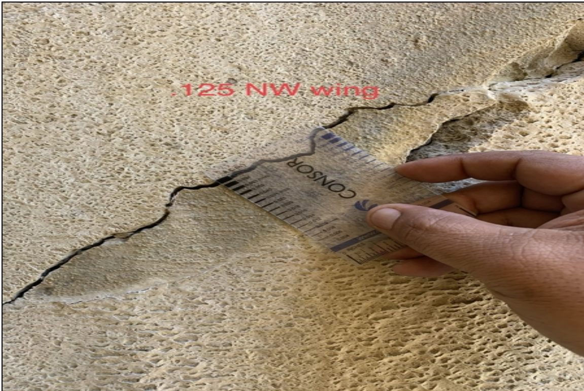
.125 NW wing crack
