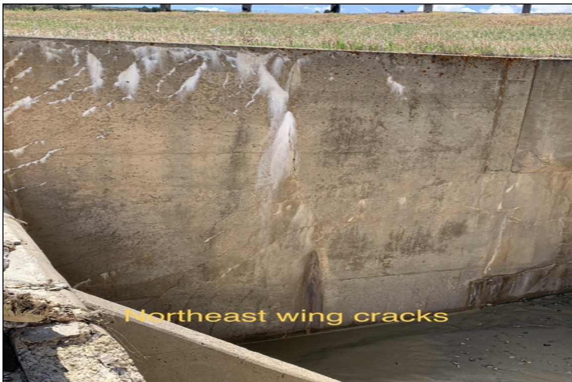
NE wing cracks
