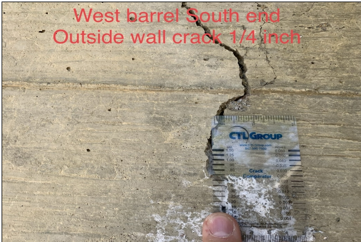
West barrel south end outside wall cracks 1/4"
