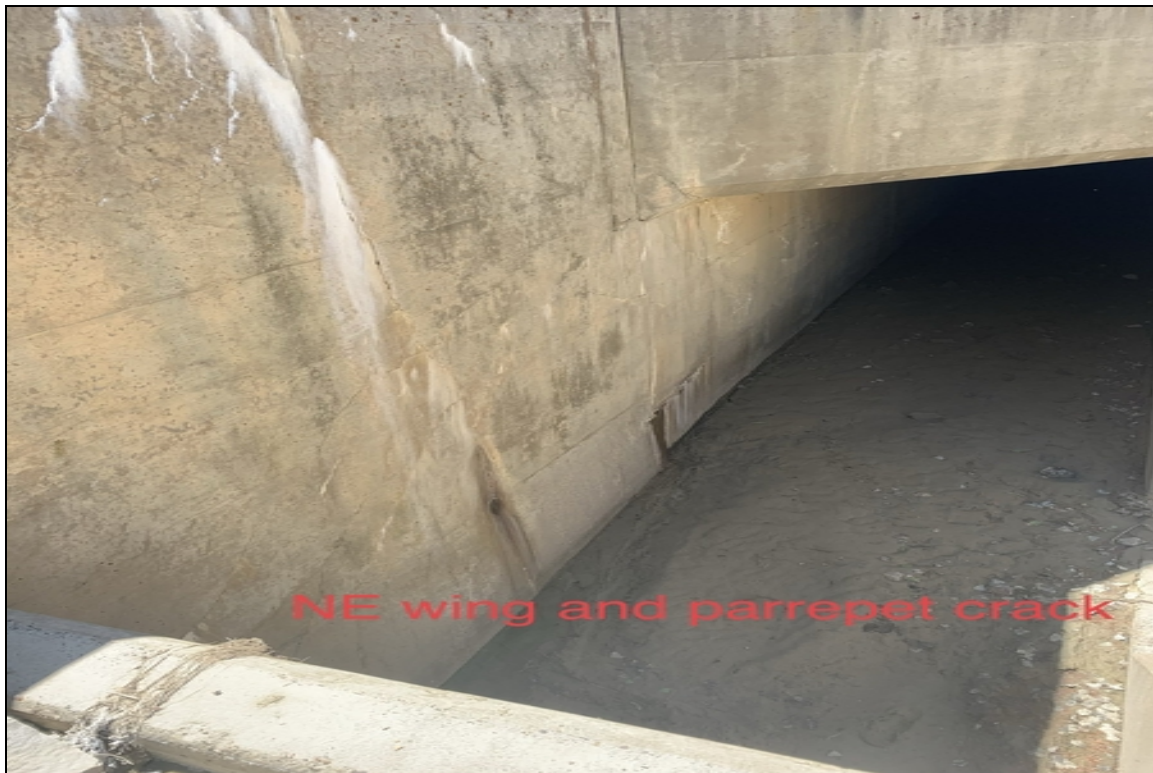
NE wing and parapet cracks
