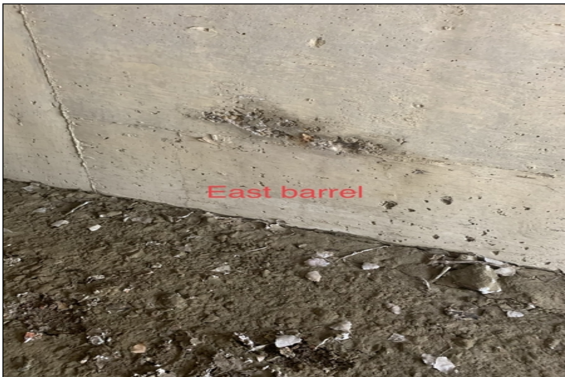
East barrel inner wall honeycomb
