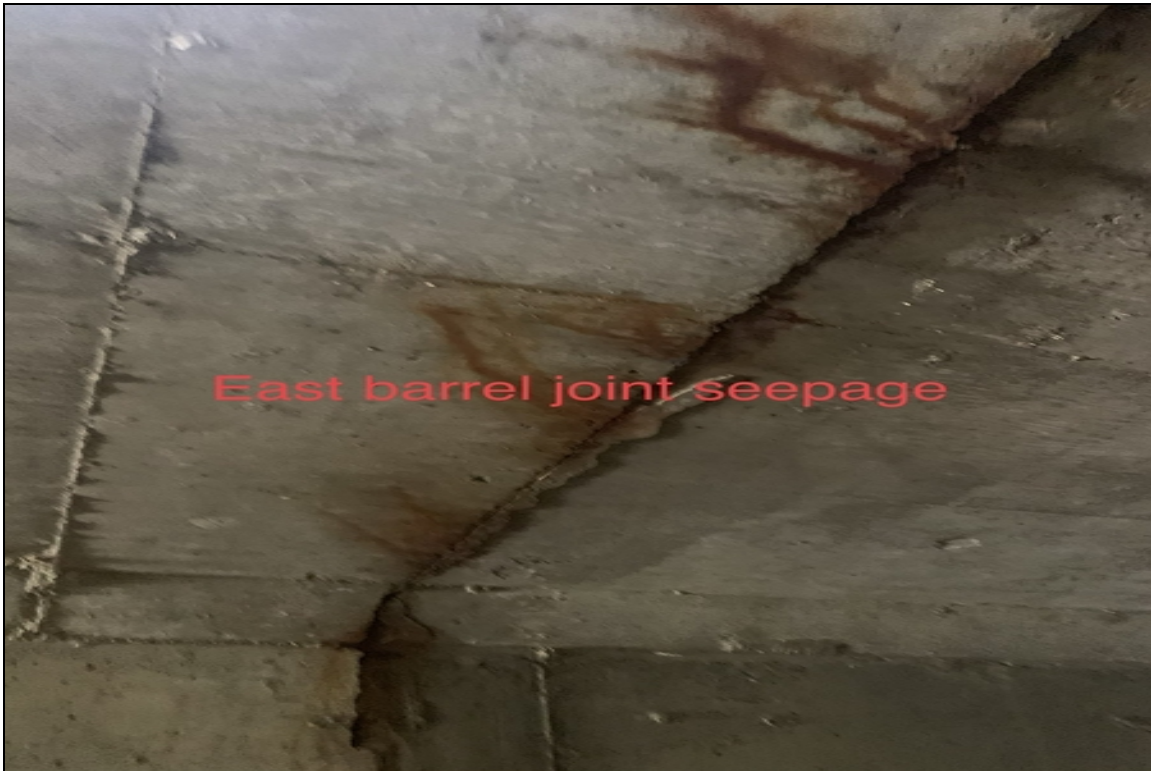
East barrel joint seepage roof
