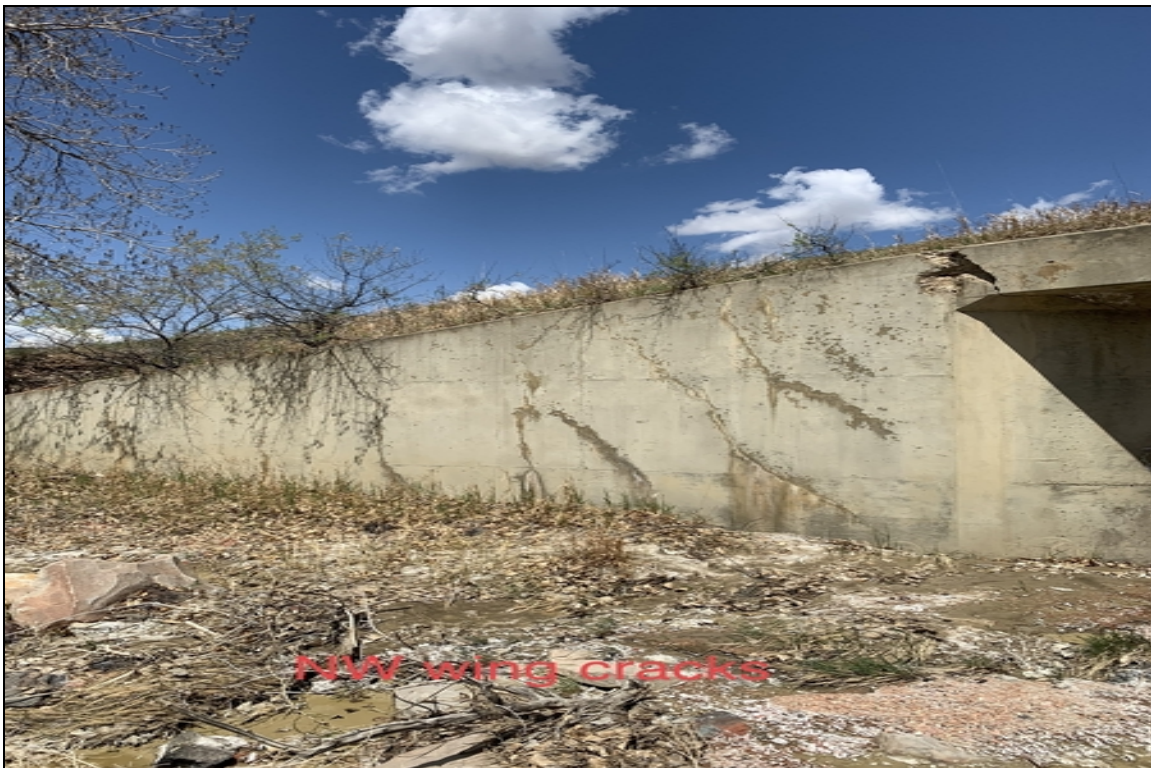
SW wing cracks ....not NW
