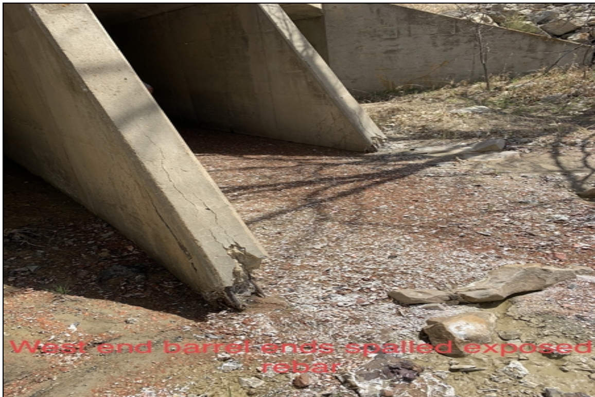
South end barrel ends spalled exposed rebar ..not west
