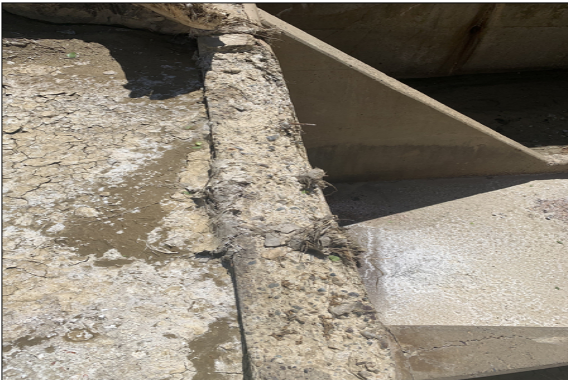
Drop inlet lip spalling
