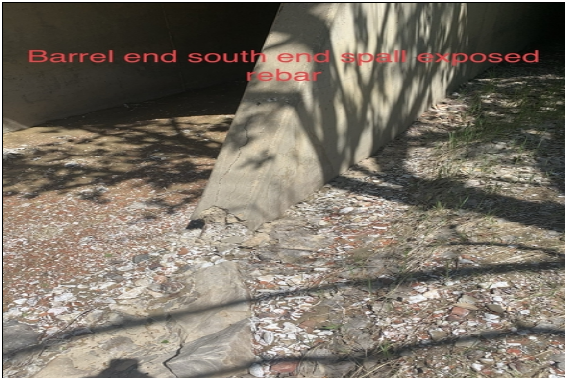
Barrel end south end spall exposed rebar
