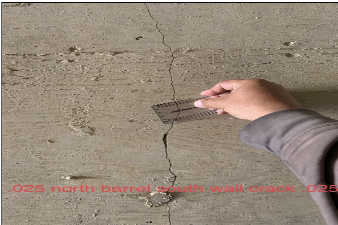
.025 west barrel south wall crack Not north
