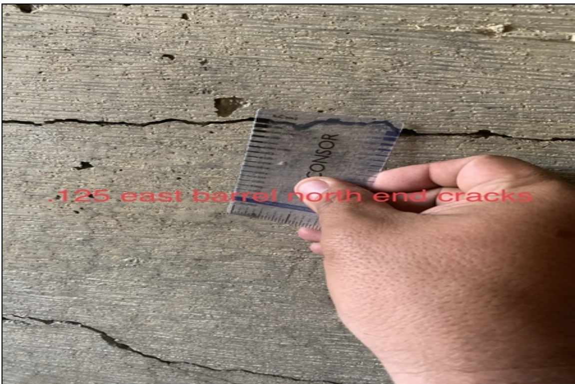
.125 east barrel outside wall crack north end
