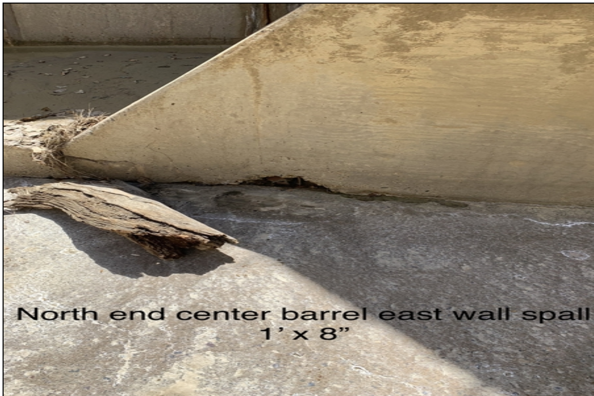
North end center barrel east wall spill 1'x8"
