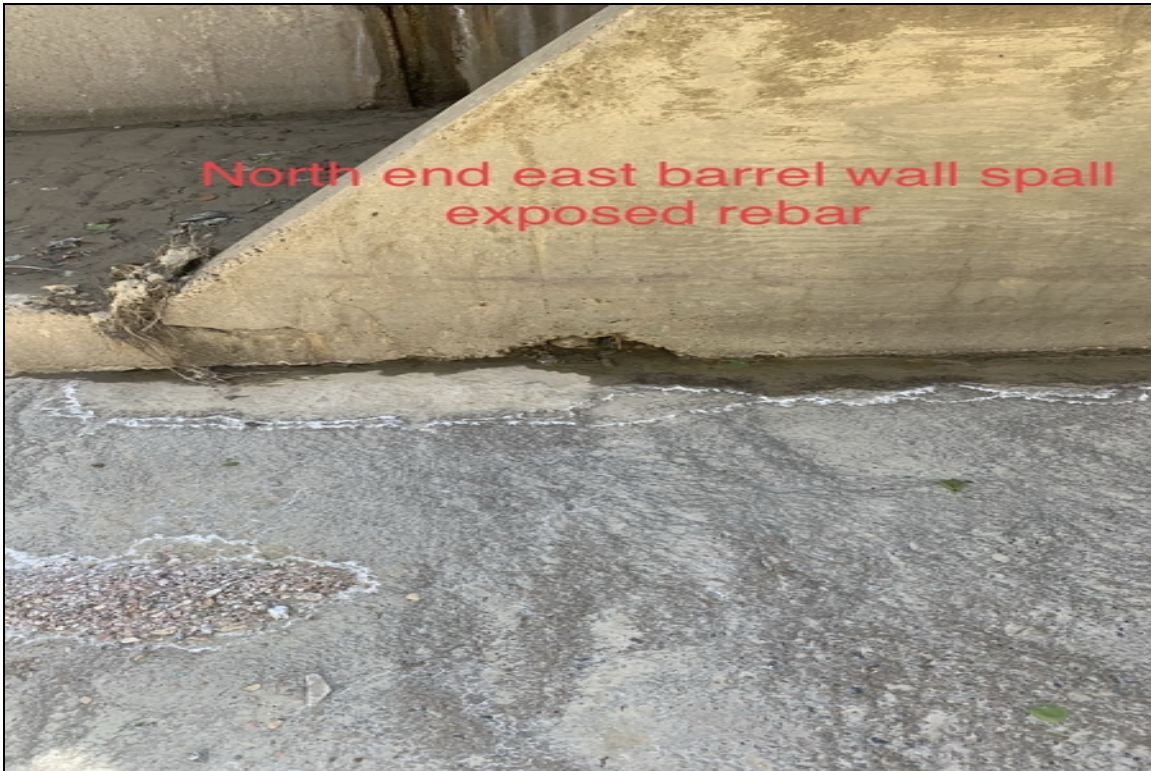
North end east barrel inner wall spall and exposed rebar
