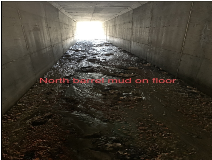
West barrel mud on floor Not north
