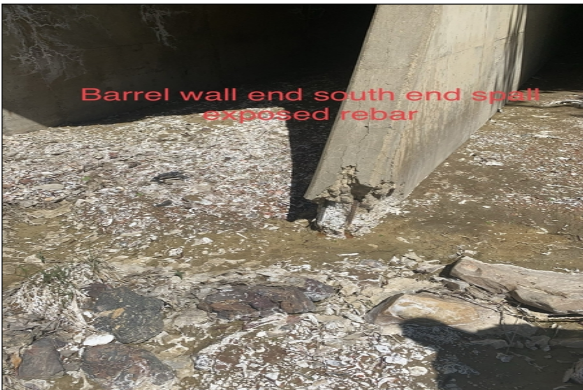
Barrel wall end south spall exposed rebar
