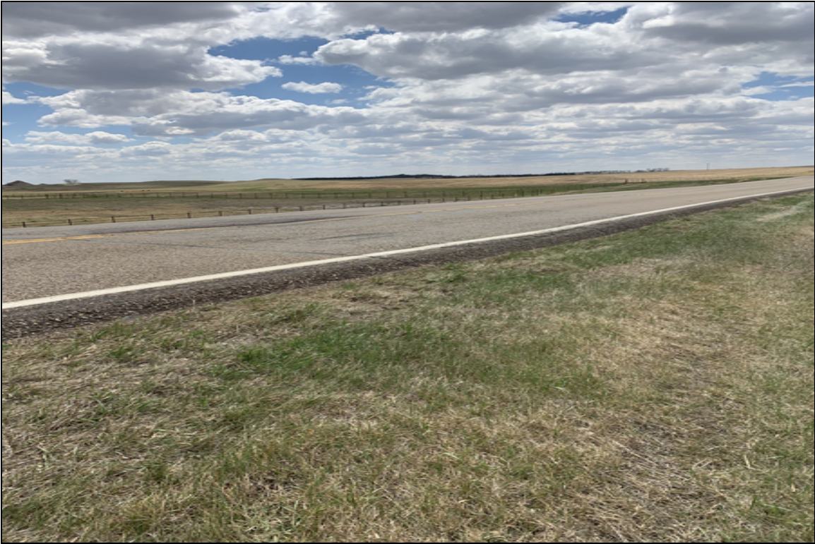
Top road settlement
