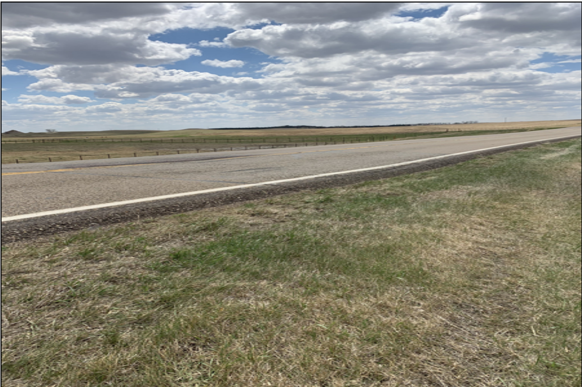
Top road settlement
