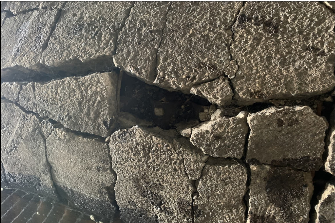
Can see bottom of floor bolts thru conc
