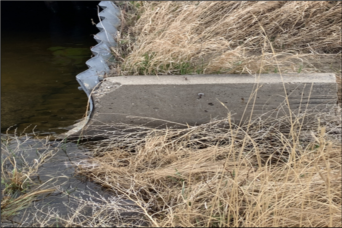
West headwall crack
