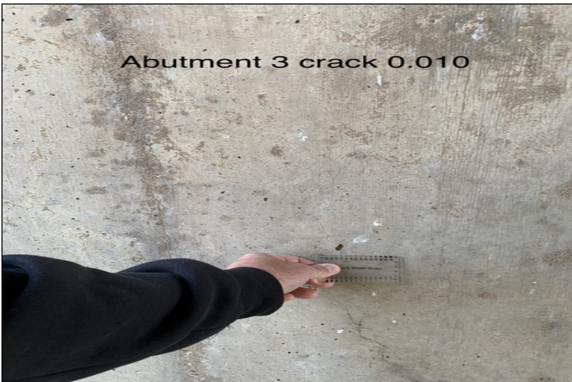
Abutment 3 crack .010
