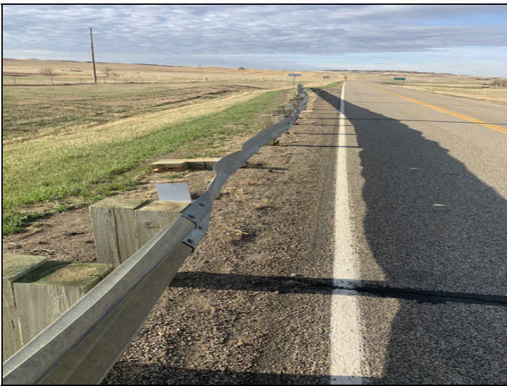
SE guardrail damage 3 post broke
