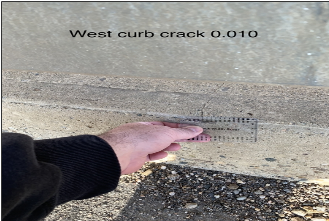
West curb crack .010
