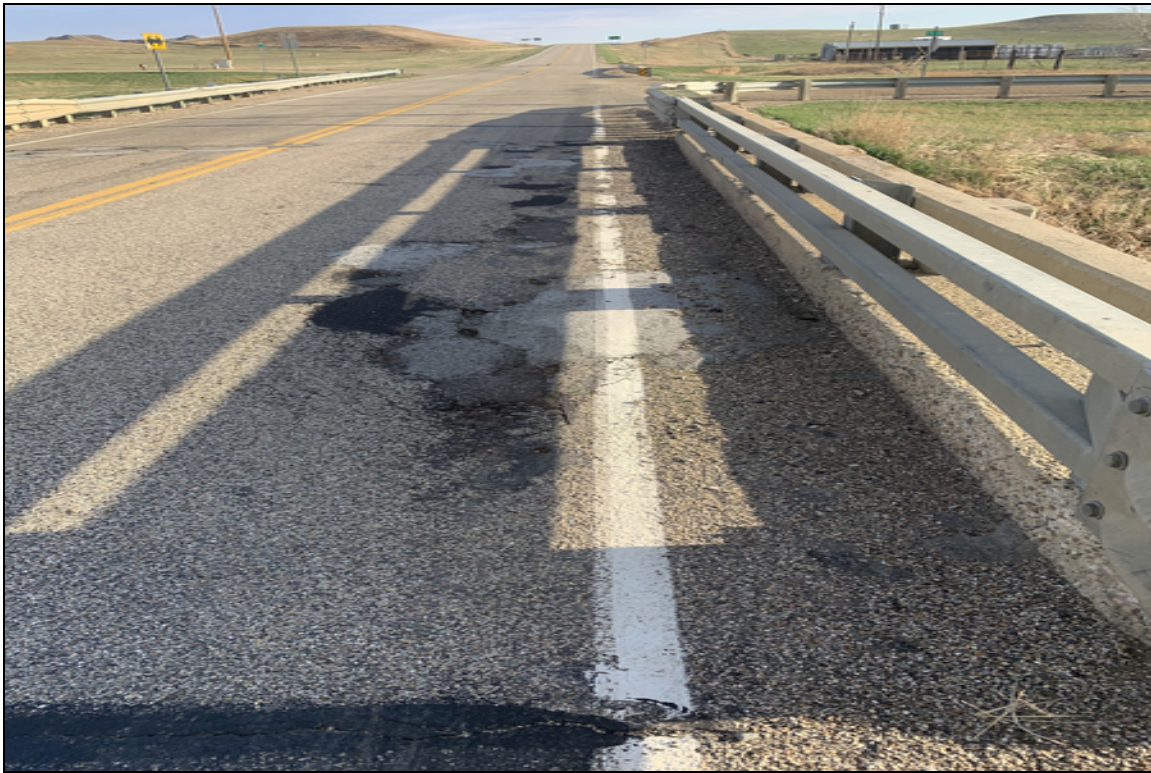
NB lane wearing surface spalls
