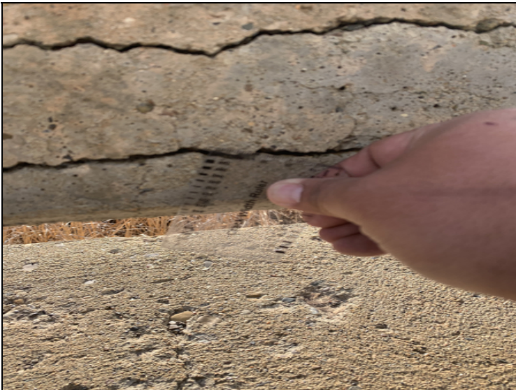
East conc rail crack bigger then .100
