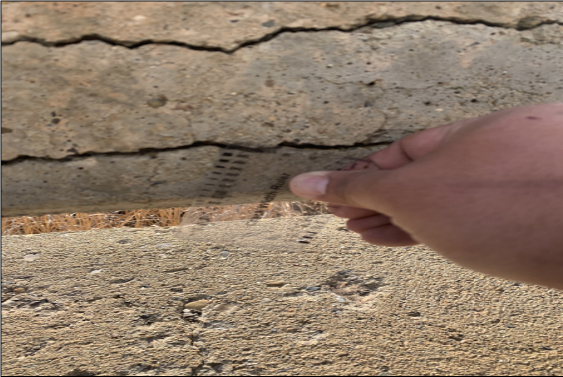
East conc rail crack bigger then .100
