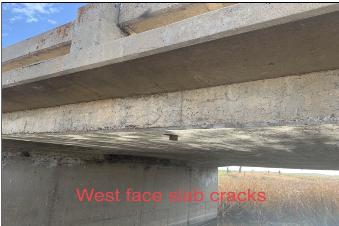
West face slab cracks
