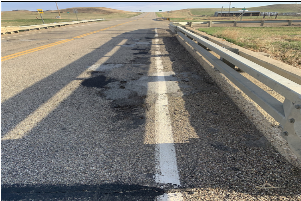
NB lane wearing surface spalls
