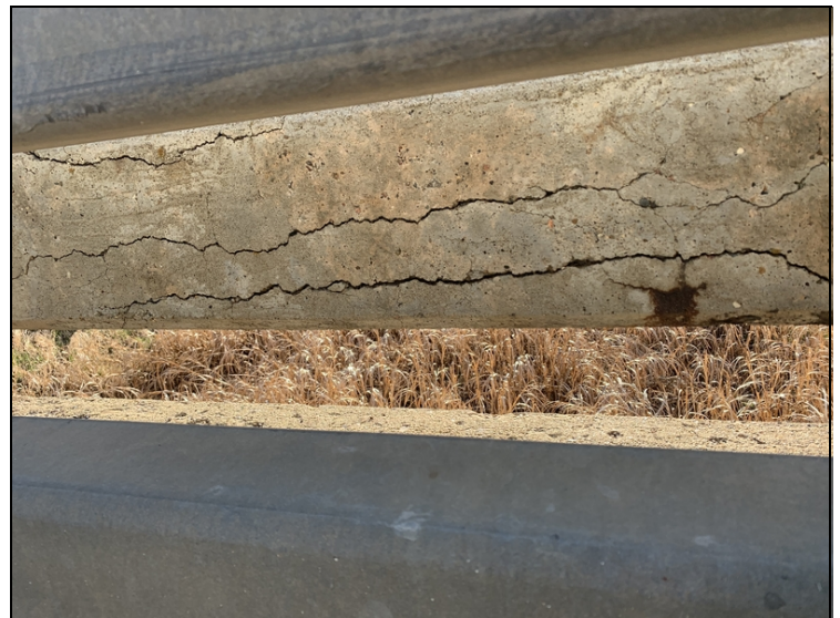
East conc rail cracks
