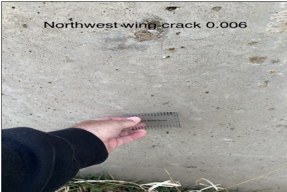
NW wing cracks .006
