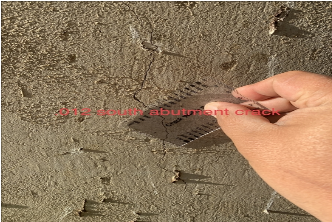
.012 south abutment crack
