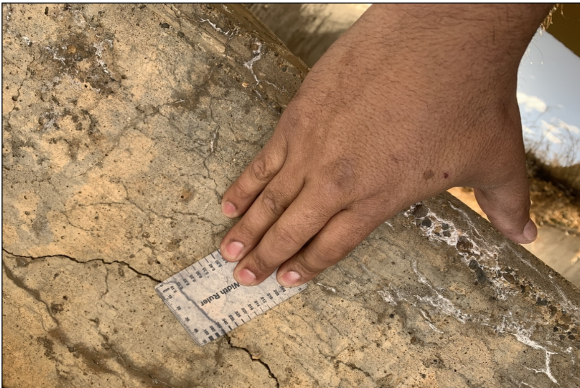
West face slab crack about pier .060
