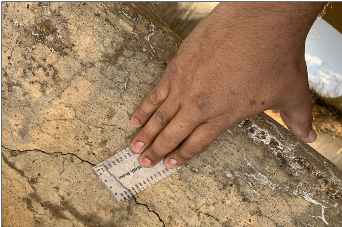
West face slab crack about pier .060
