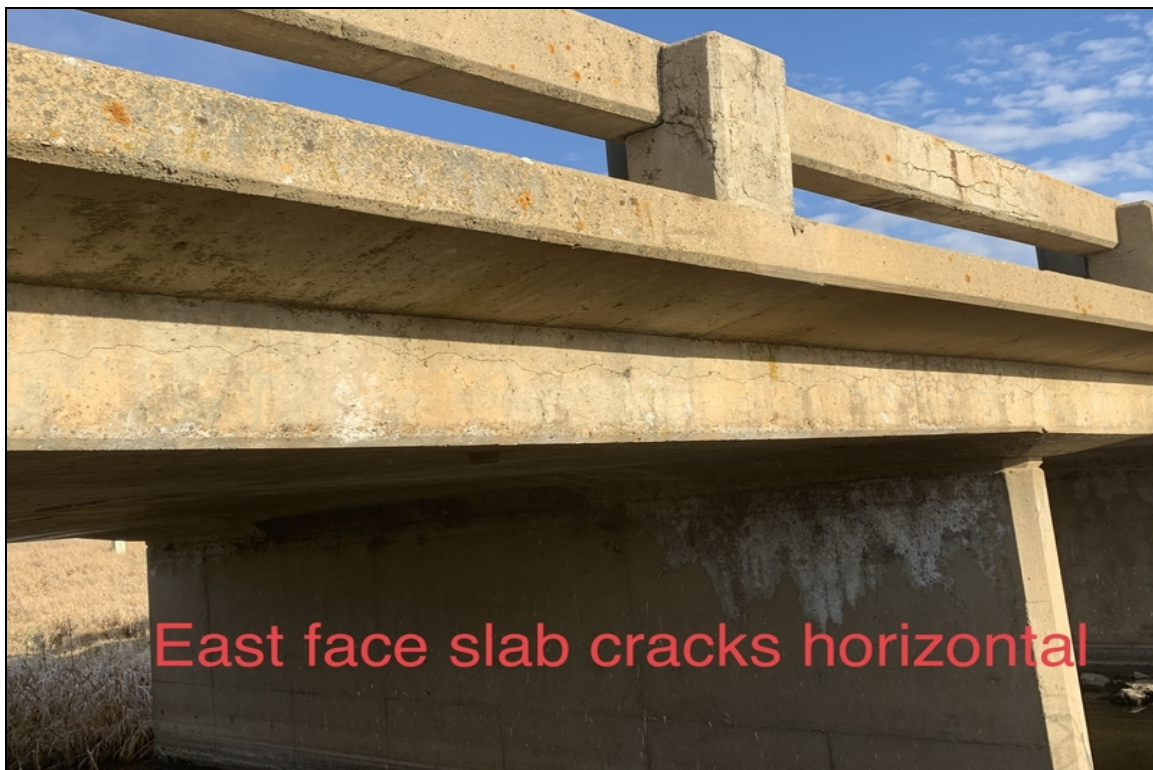
East face slab cracks horizontal
