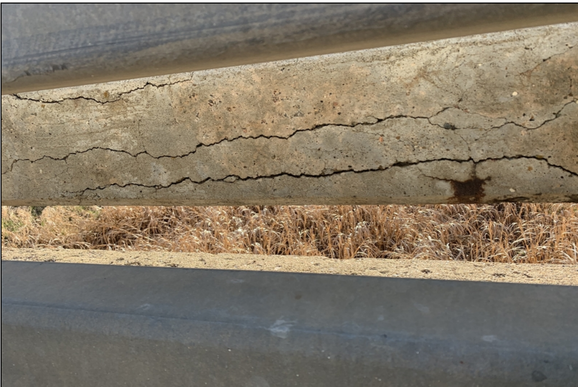
East conc rail cracks
