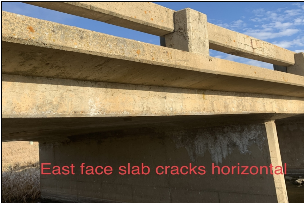
East face slab cracks horizontal
