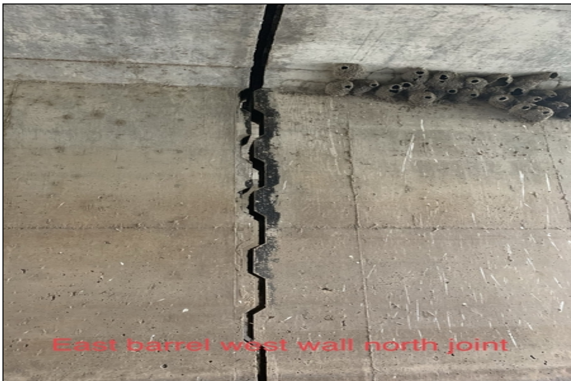
East barrel west wall north const joint open more at top then bottom
