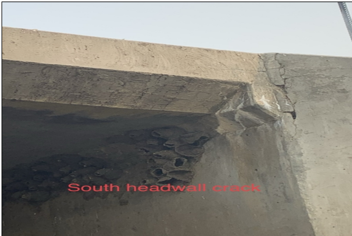
South headwall east end cracks
