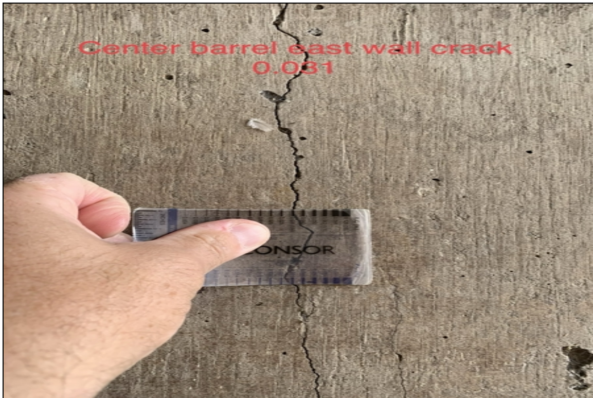
Center barrel east wall crack .031
