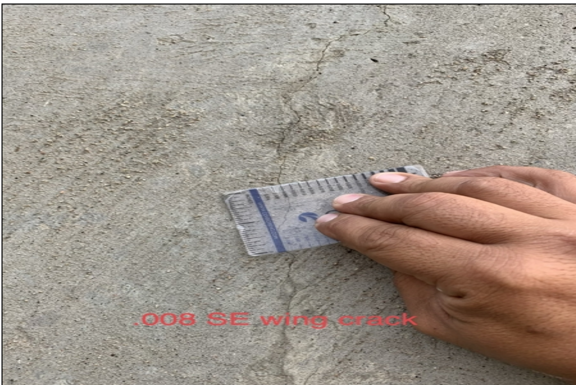
.008 SE wing crack vertical
