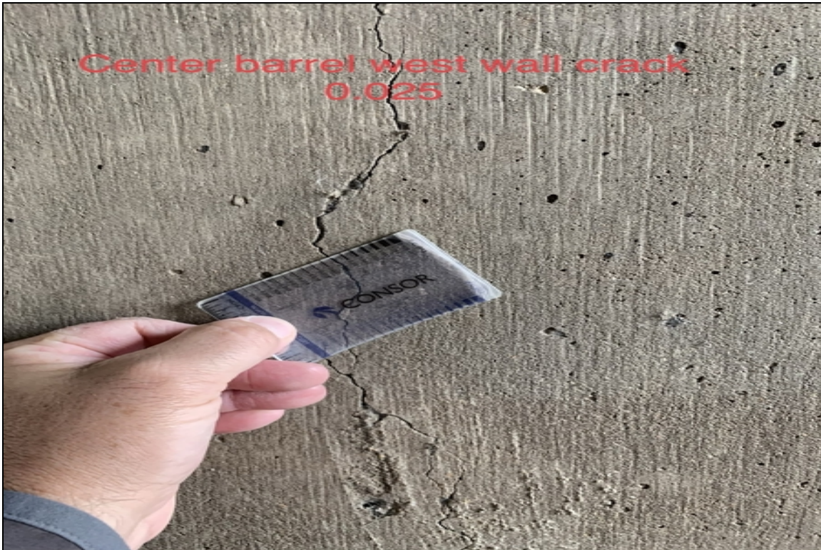
Center barrel west wall crack .025
