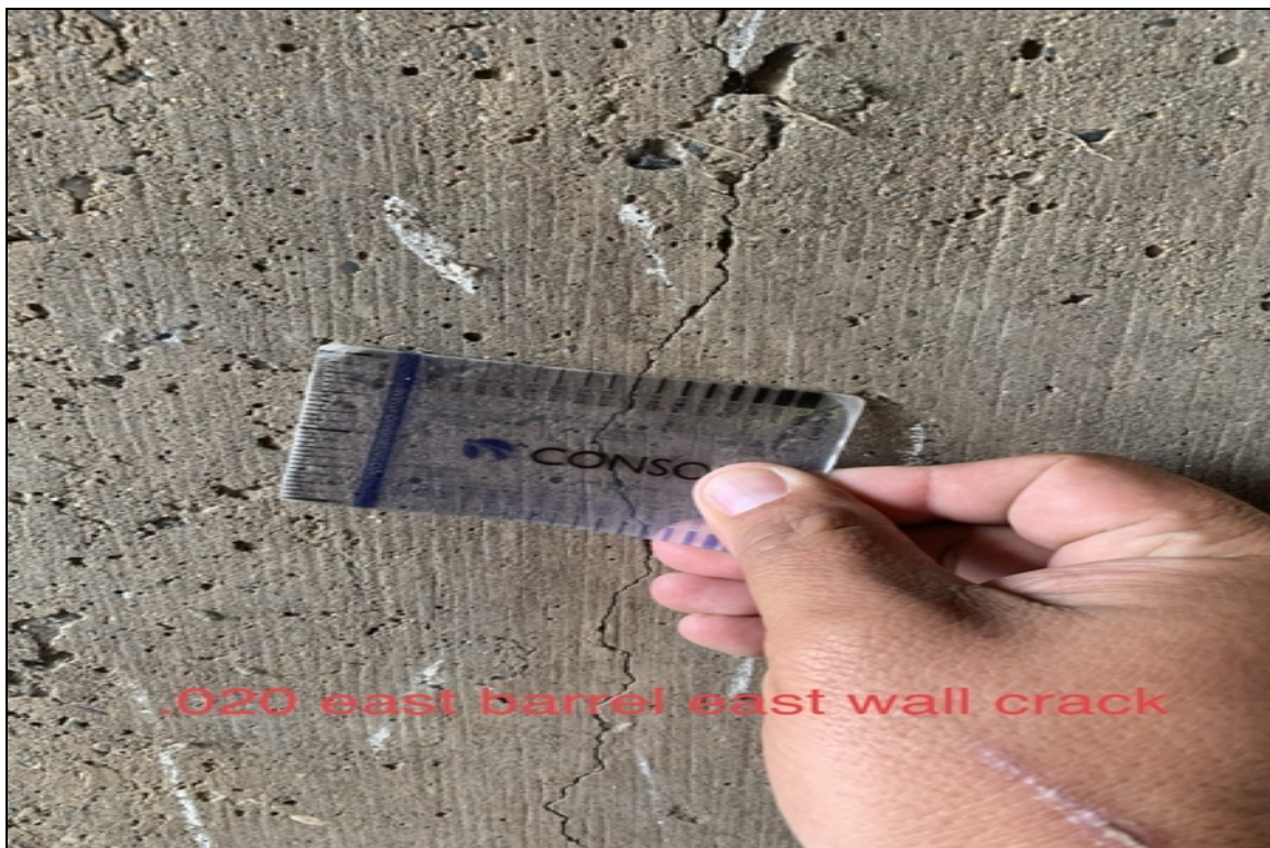
.020 east barrel east wall crack
