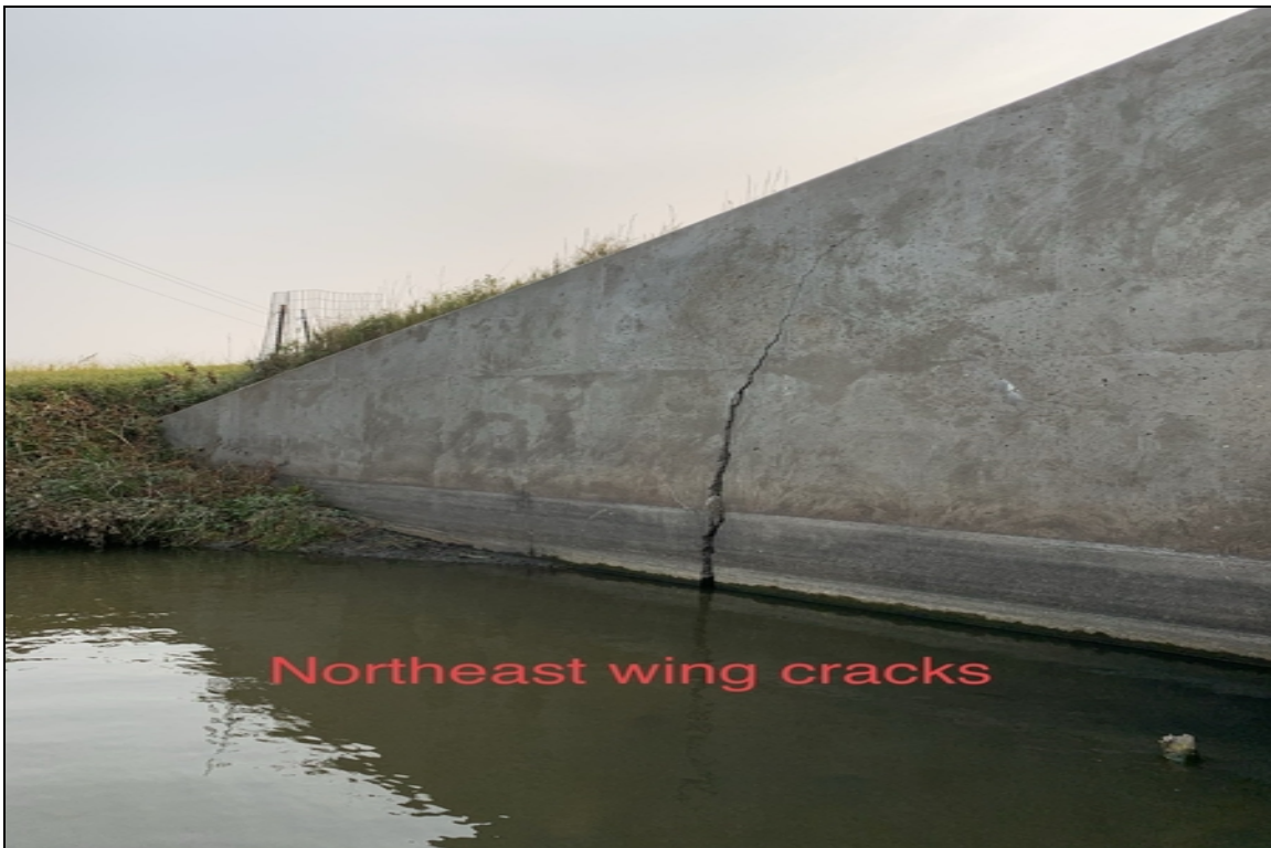
NE wing crack
