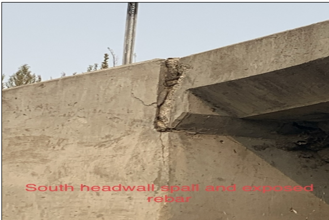
South headwall west end spalled and exposed rebar
