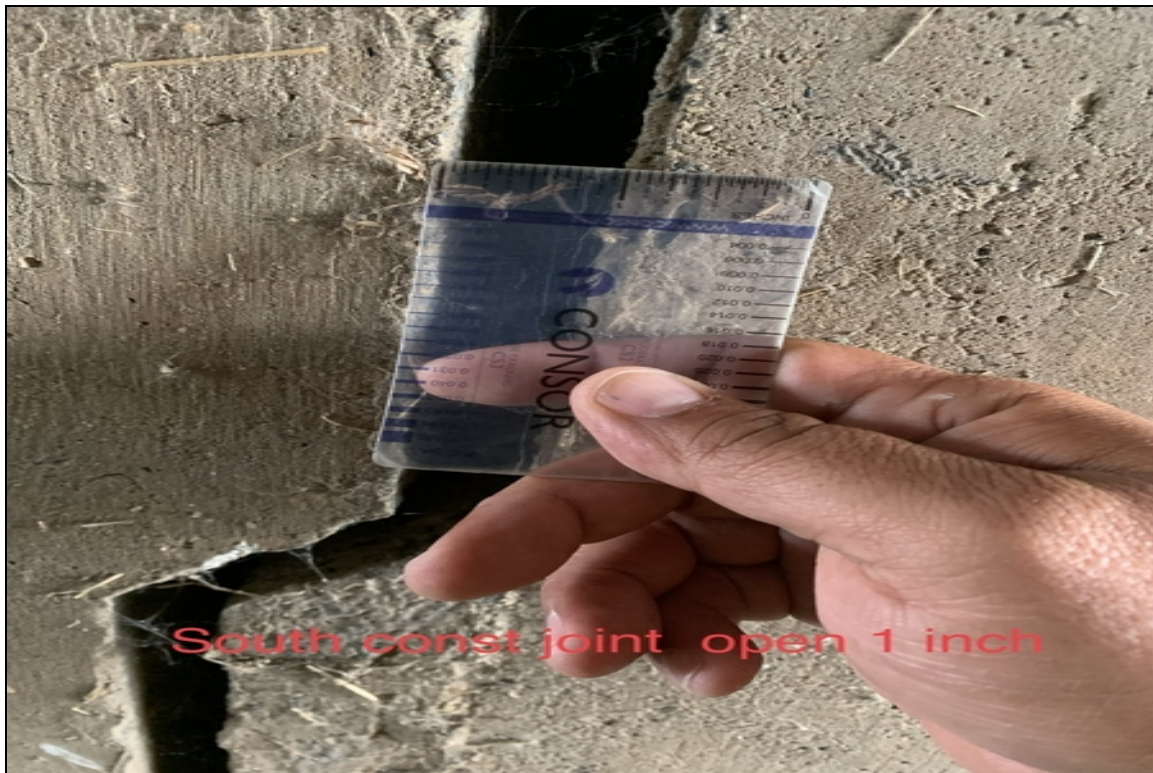
South const joint open 1"
