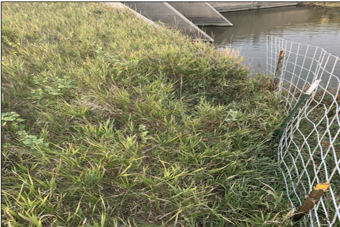
Erosion behind NE wing 5'x3'x1'
