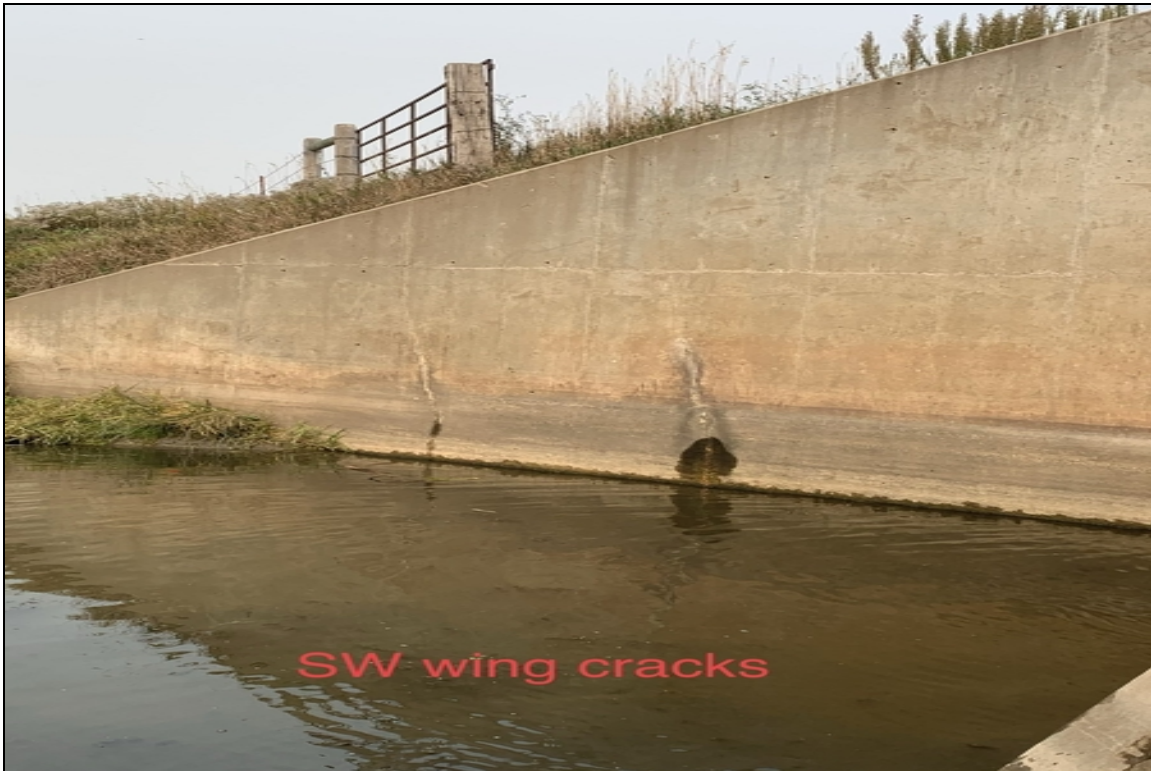
SW wing cracks
