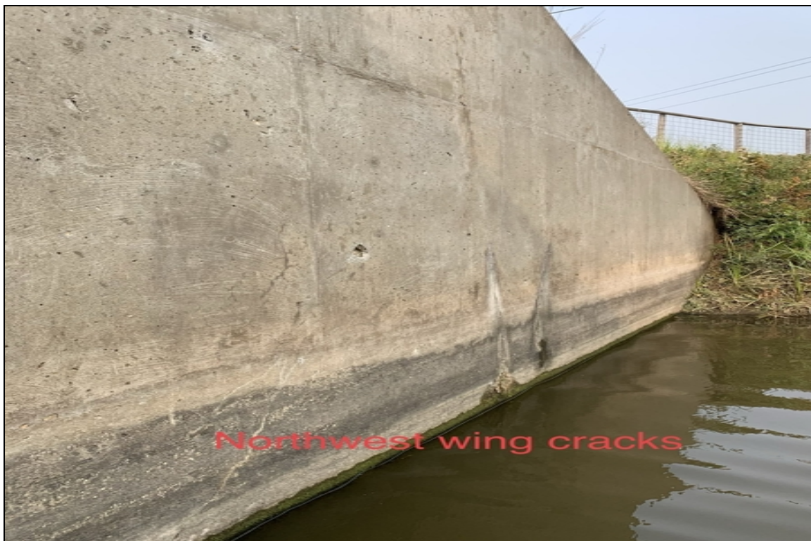
NW wing cracks
