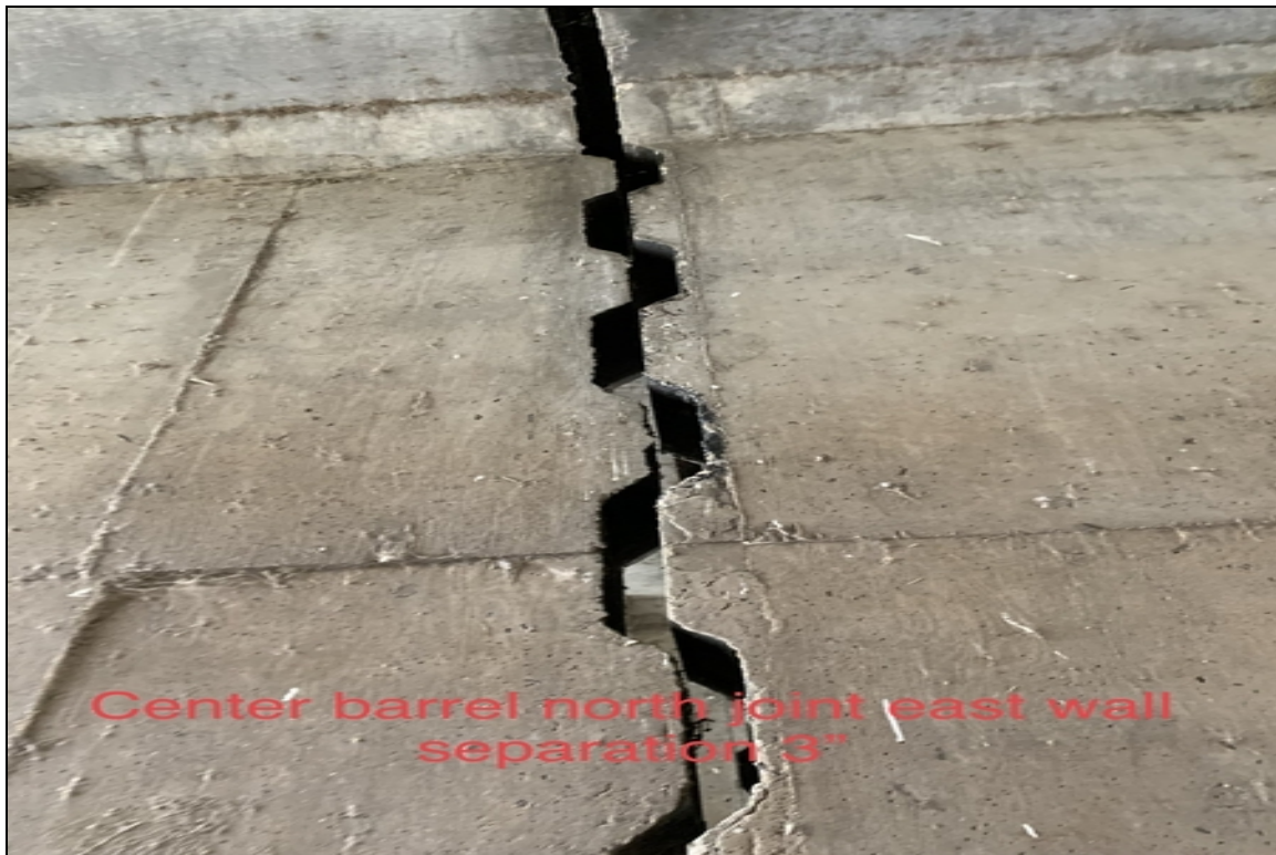
Center barrel north joint east wall separation 3"
