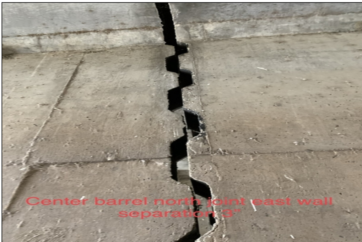
Center barrel north joint east wall separation 3"
