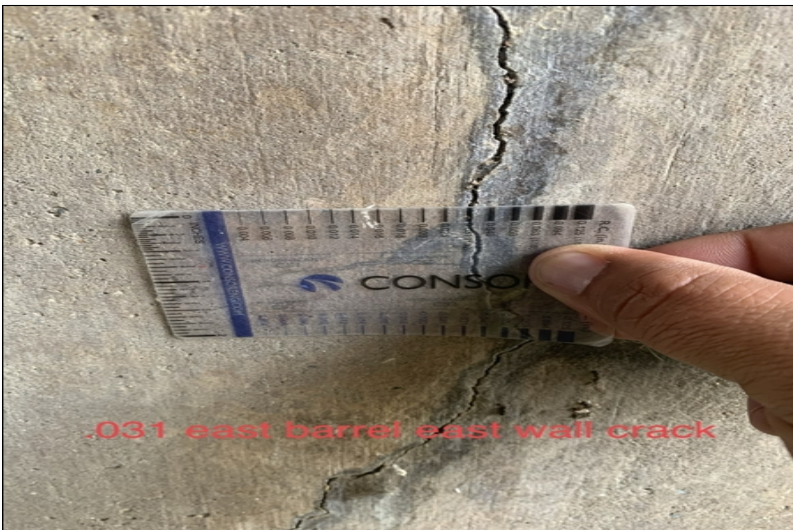
.031 east barrel east wall crack
