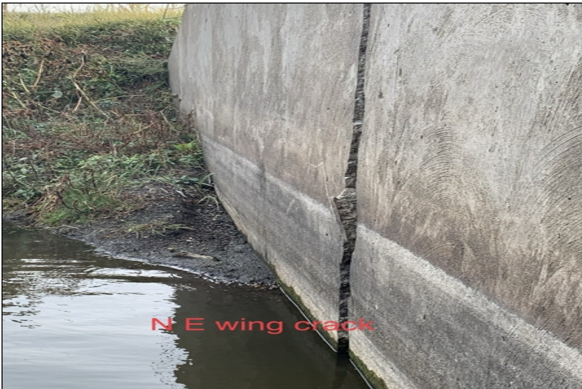
NE wing crack
