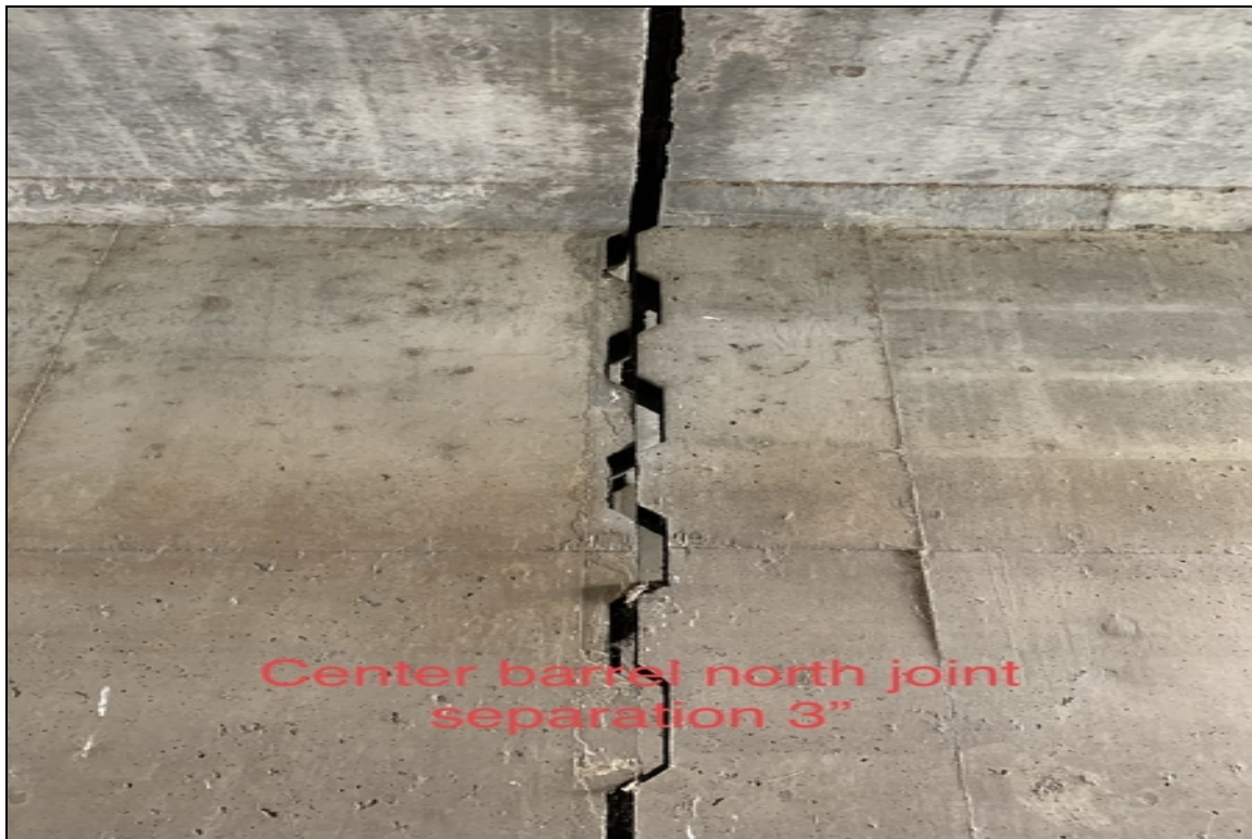
Center barrel north joint separation 3"
