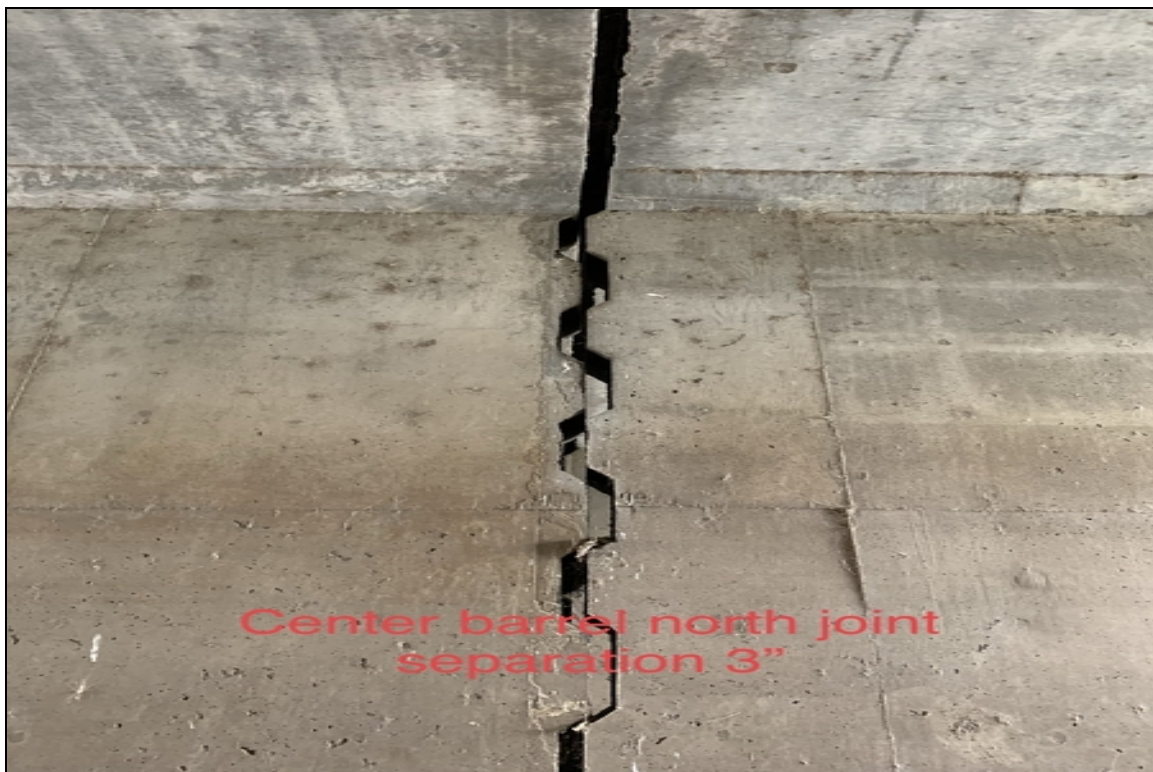
Center barrel north joint separation 3"
