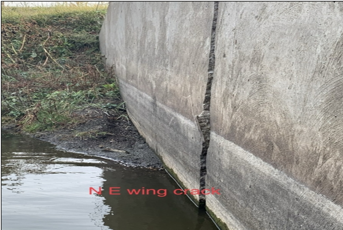
NE wing crack
