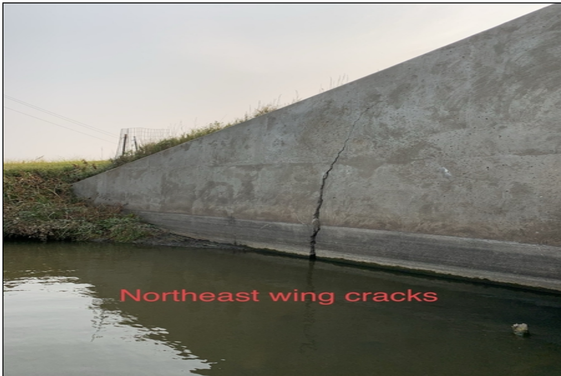
NE wing crack
