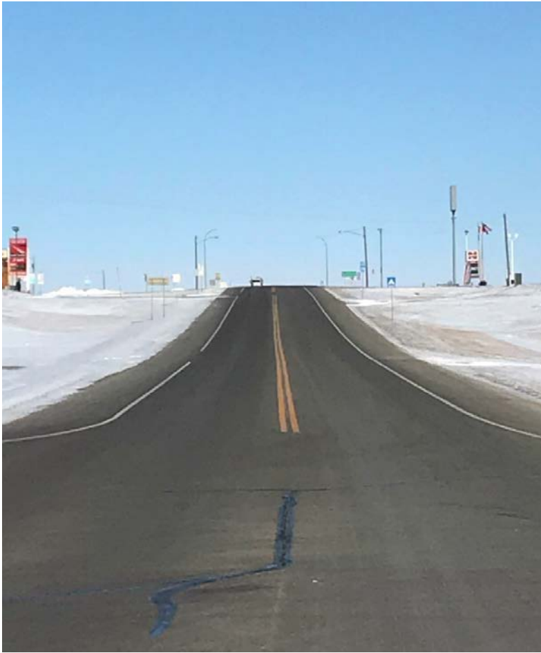
Located at 5 th Avenue NE RP 75.249
