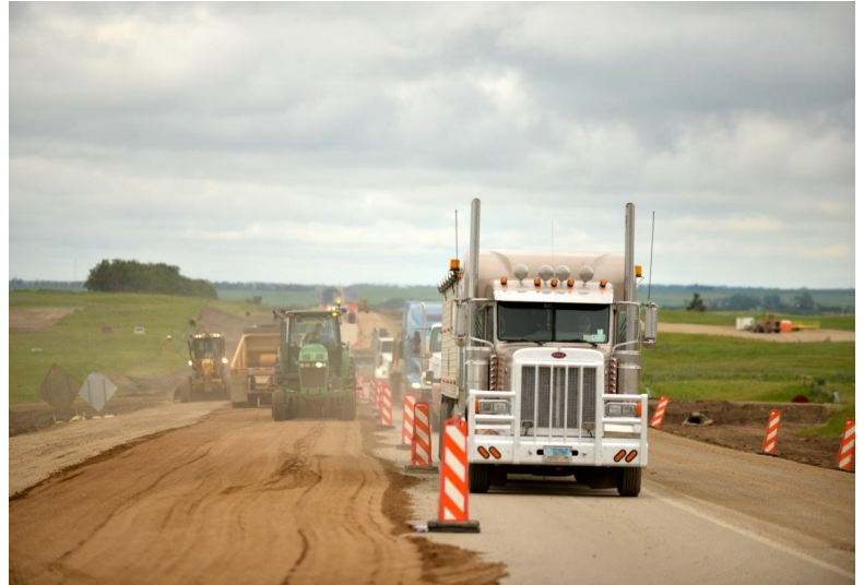
Construction on ND Highway 23 east of New Town.
