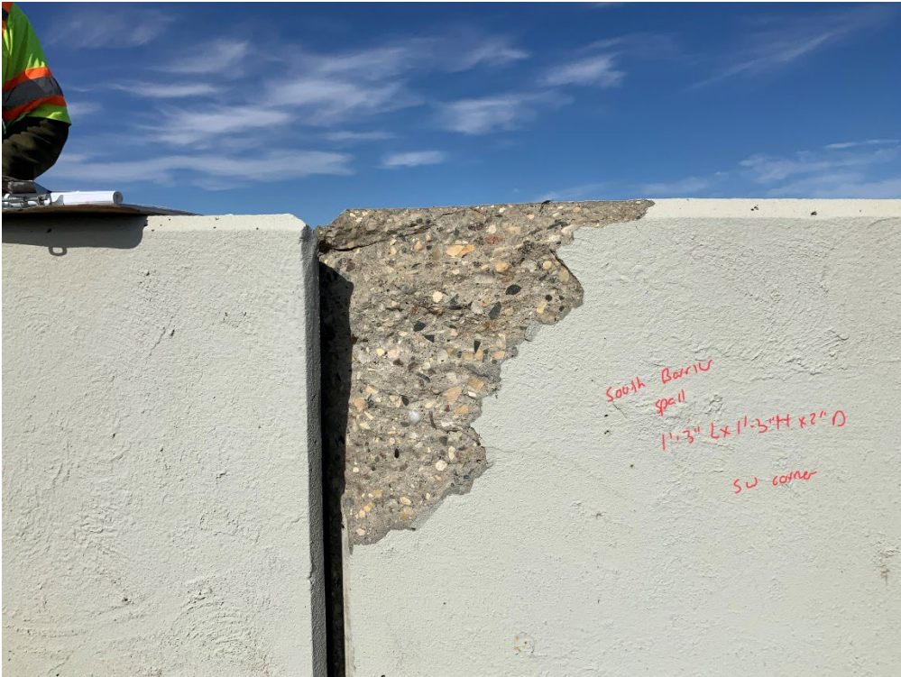
Picture #5 – Back Face Barrier SW Corner
