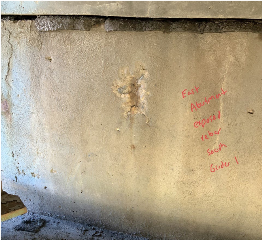
Picture #4 – East Abutment Backwall
