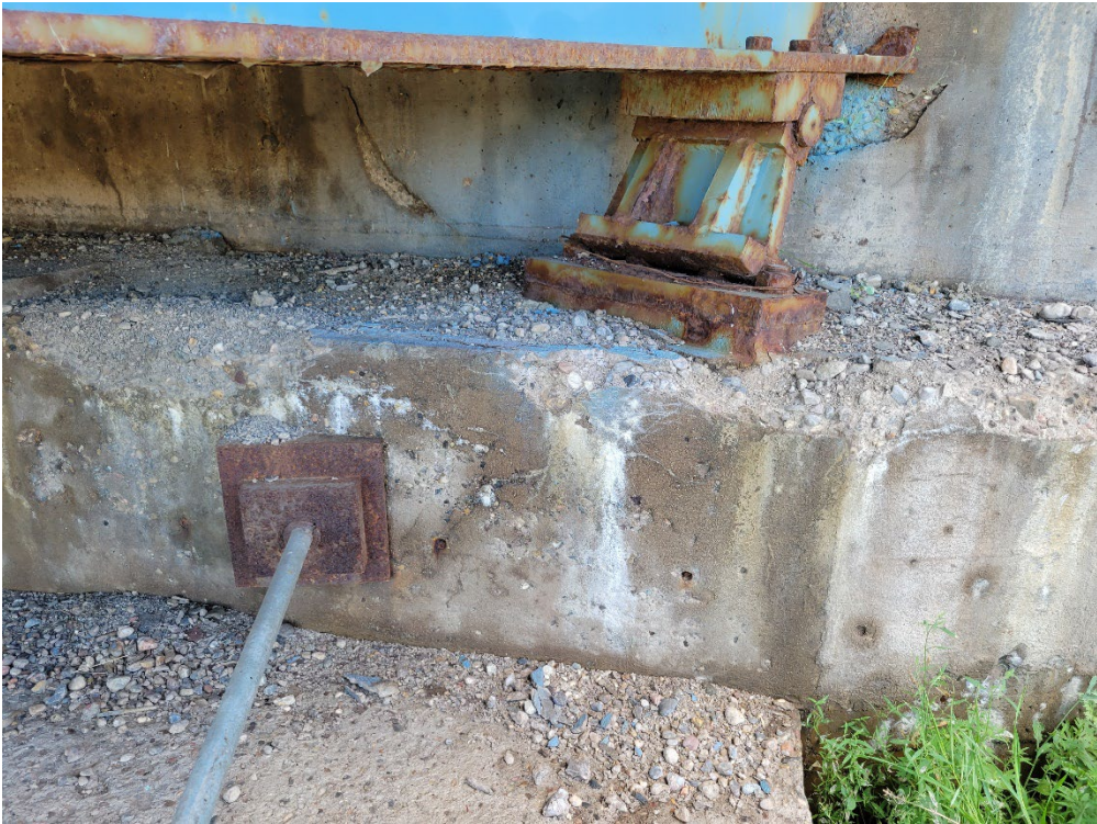
Picture #1 – West Abutment Bearing Seat
