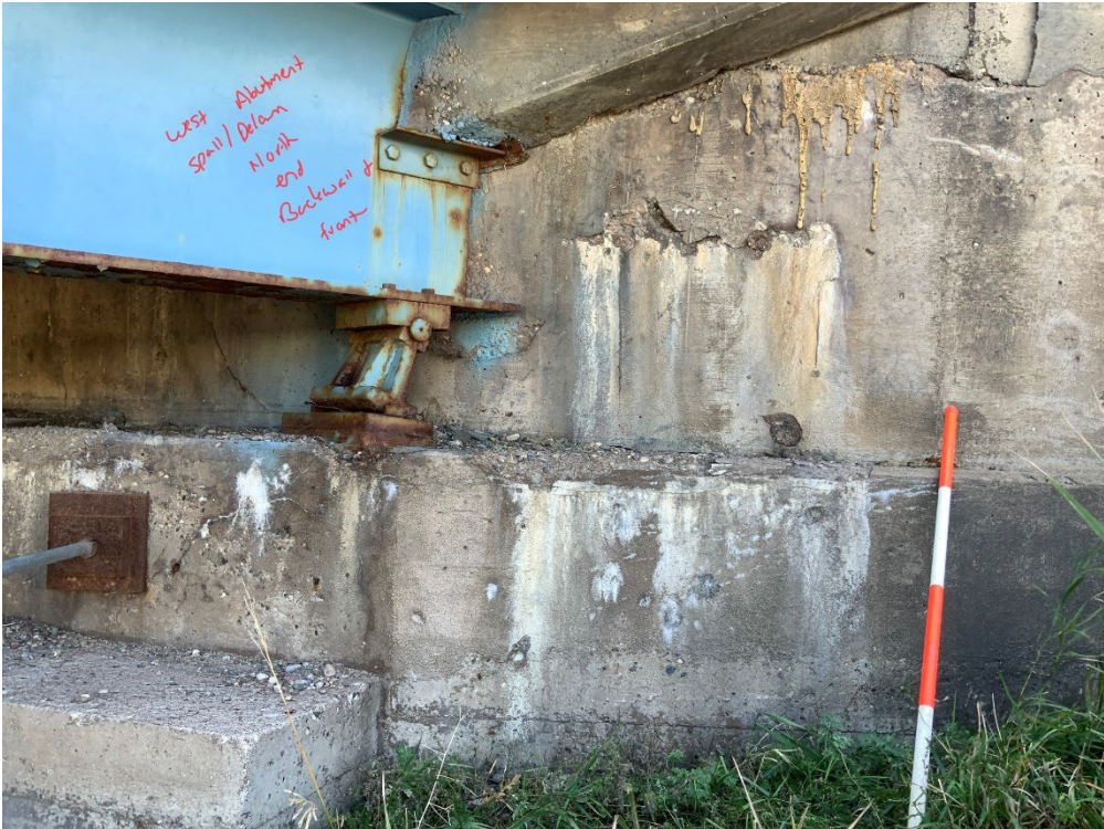
Picture #2 – West Abutment Backwall
