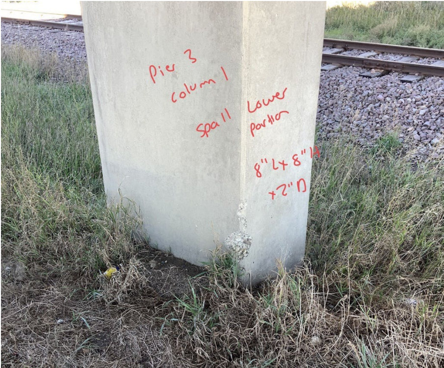
Picture #6 – Pier 3: Column 1
