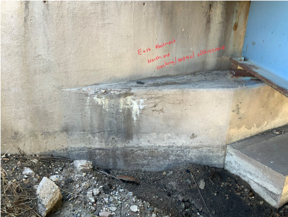
Picture #3 – East Abutment Bearing Seat
