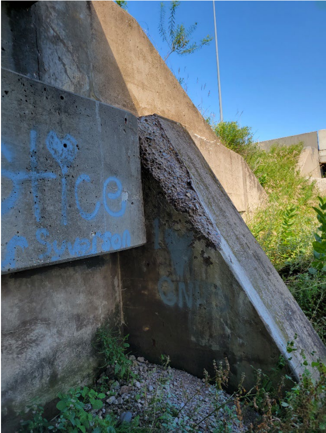
Picture #1 – West Abutment Column/Beam Seat
