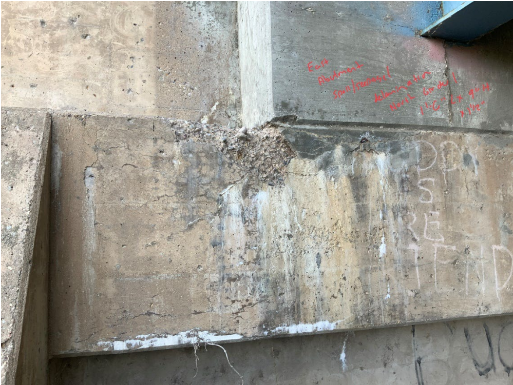
Picture #3 – East Abutment Beam Seat
