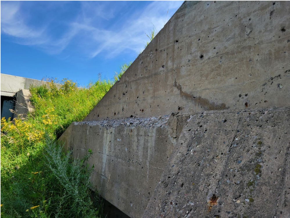
Picture #4 – East Abutment North Wing
