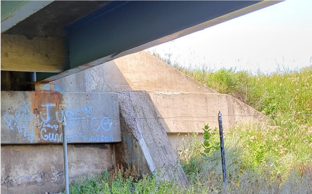
Picture #2 – West Abutment Column/ Beam Seat & North Wing
