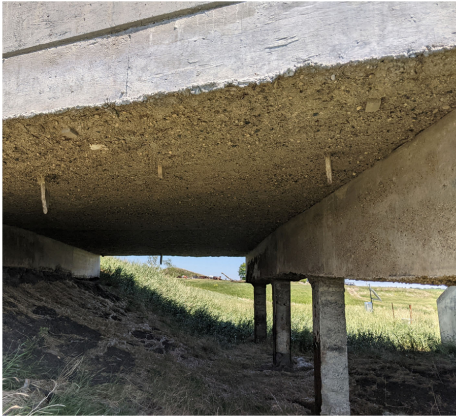
Figure 3 – Excavation Behind Existing Abutment
