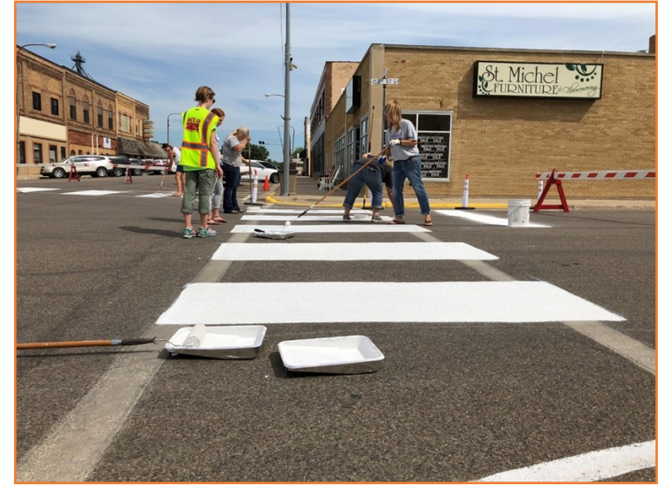
Installations Usually Took Less Than One Day
