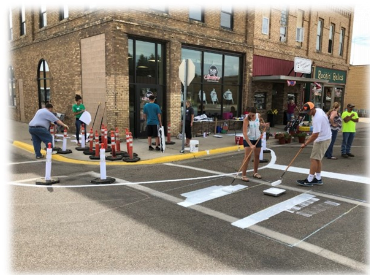
Volunteers Installing Enhanced Crosswalks
