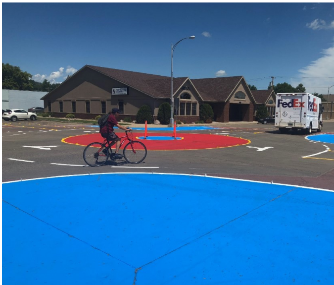
Temporary Roundabout in Mandan, ND
